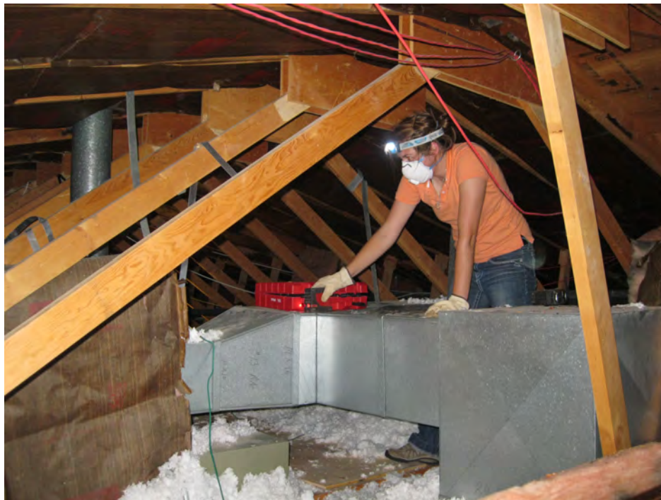
Using a laser level to determine the deflection of a truss
