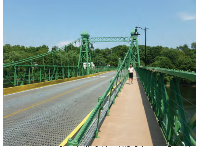
Riegelsville Bridge, NJR, Pohatcong Township
