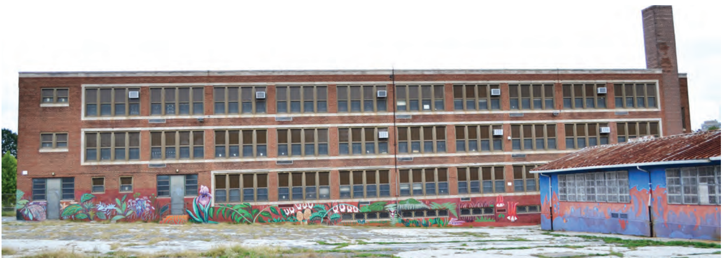
Figure 10. Photograph of Drew School Elementary south elevation. 2012.
