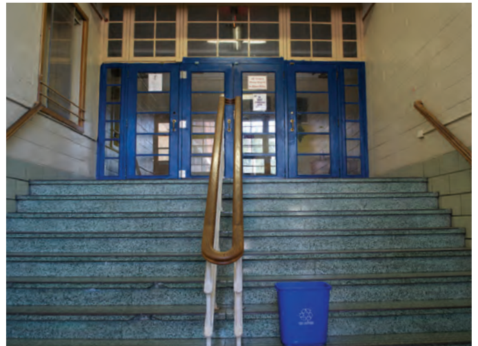
Figure 26. Photograph, main entrance stairs
