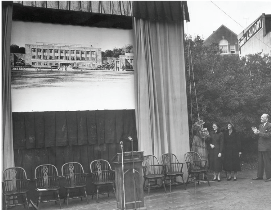
Image 16. The groundbreaking of Dietrich Hall, 1951.
