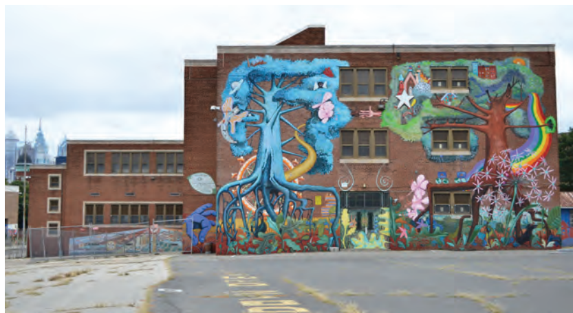
Figure 8. Photograph of Drew School Elementary west elevation. 2012.
