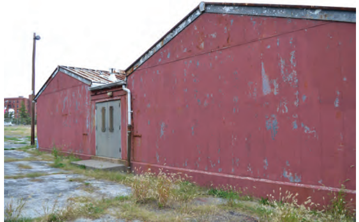
Figure 12. Photograph of Drew School Elementary library south facade. 2012.
