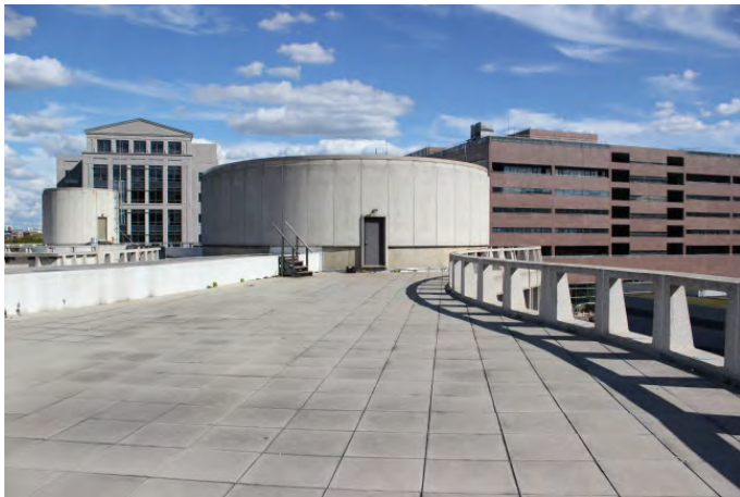
Figure 11. Two of the three penthouses on the roof of the Police Administration Building. This photograph was taken during a site visit on September 20, 2012.
