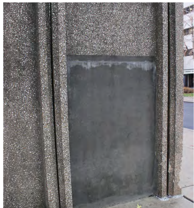
Figure 31. Detail of inappropriate concrete infill.
