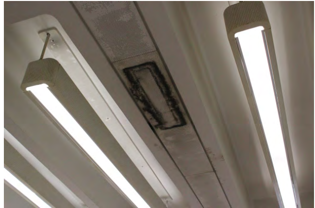
Figure 20. Detail of accumulation of dust.
