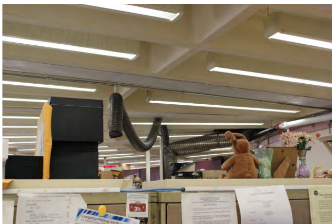
Figure 19. Photo of tube snaking through one of the workspaces.
