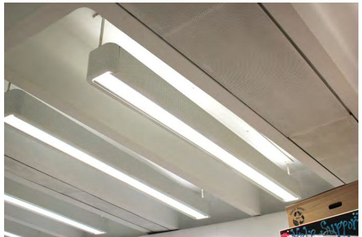
Figure 29. Detail view of the custom lights.
