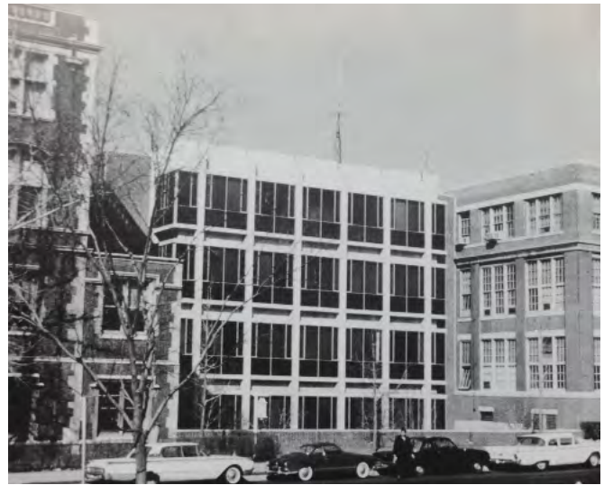
Figure 3. Moore School Pender Laboratory, 1958. Lawrence S. Williams, Inc. Process Architecture 62.
