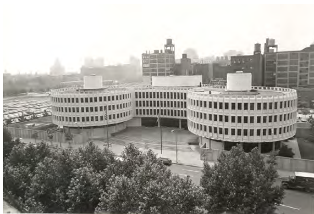
Figure 12. Looking south at the north side showing the plaza and rectilinear concrete panels.
