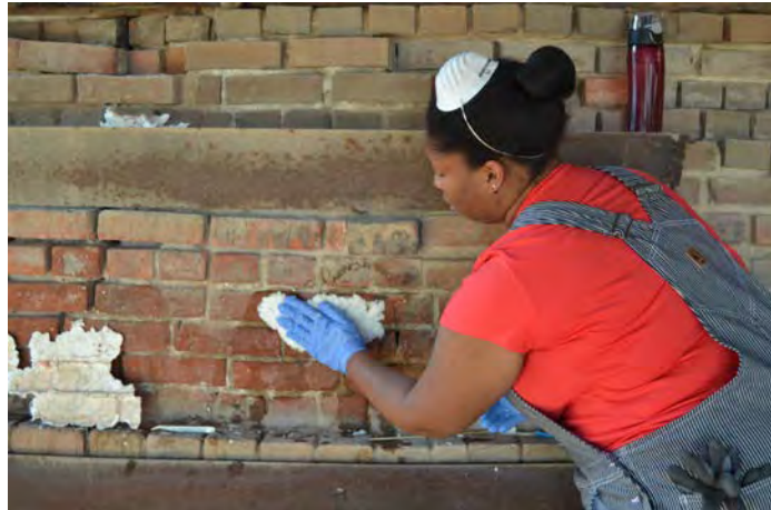
Applying paper poultice to brick kilns, 2013
