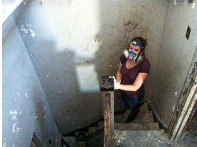
Surveying the Provident Mutual Life Insurance Building, 2013
