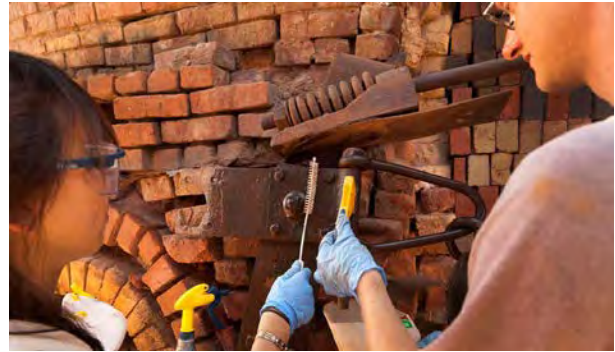
Metal component wash with a desalinating agent
