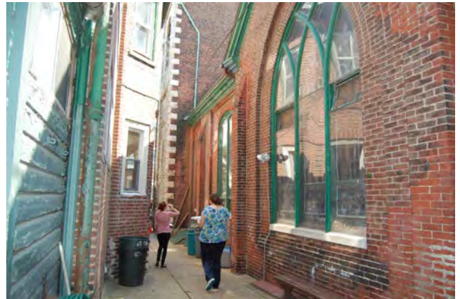
Conditions Assessment at Atonement Lutheran Church, 2013
