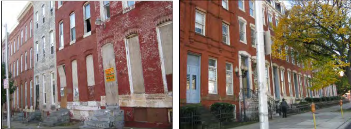
Row Houses in East Baltimore Neighborhood Before and After Rehabilitation, 2006 - 2013
