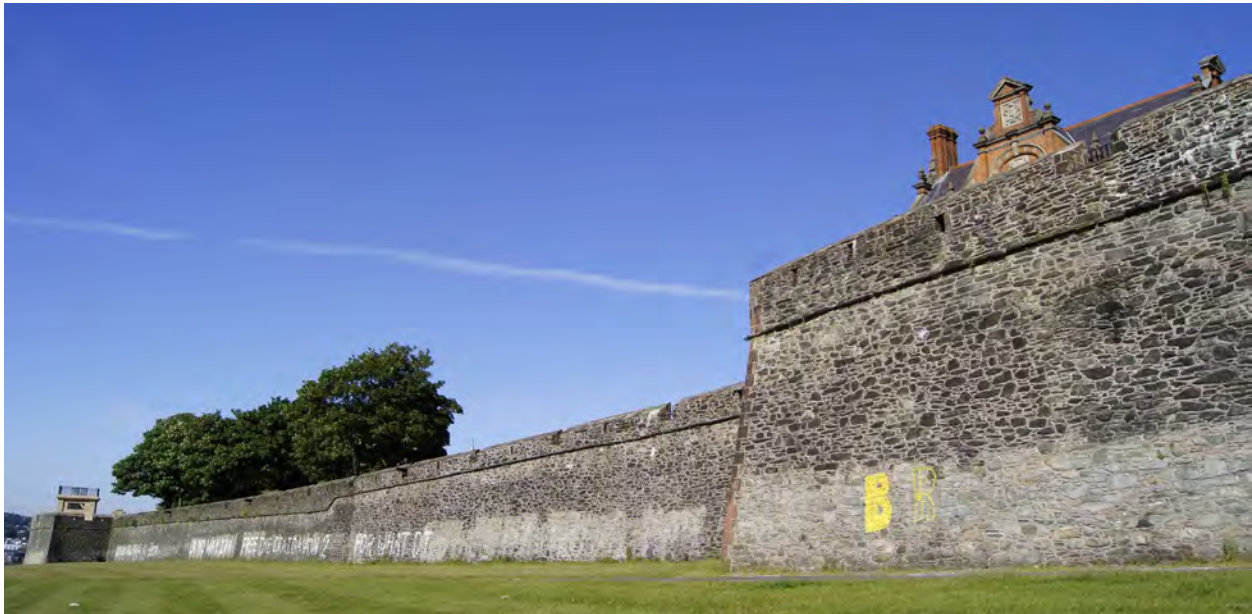
View of the 'Mall Wall' portion of Derry/Londonderry's city walls, 2013.
