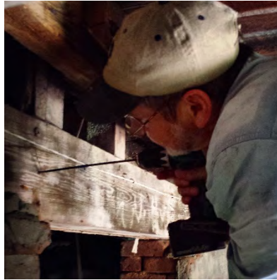
Resistance drilling a support beam under a piazza in the Battery, 2014
