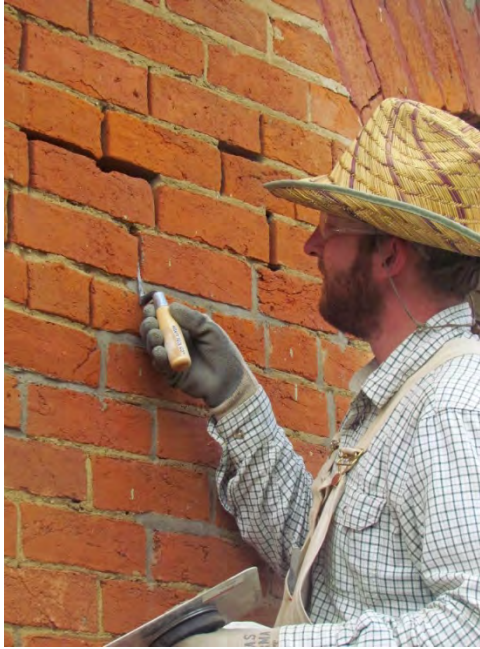
Biogrowth removal at Mt. Pleasant, June 2014
