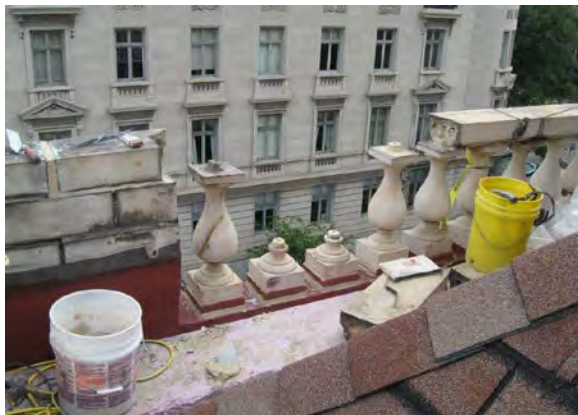
Terra cotta baluster pinning and replacement, Sulgrave Club, Washington, DC, 2014
