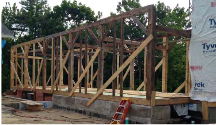
Pennell House ell erection, 2014
