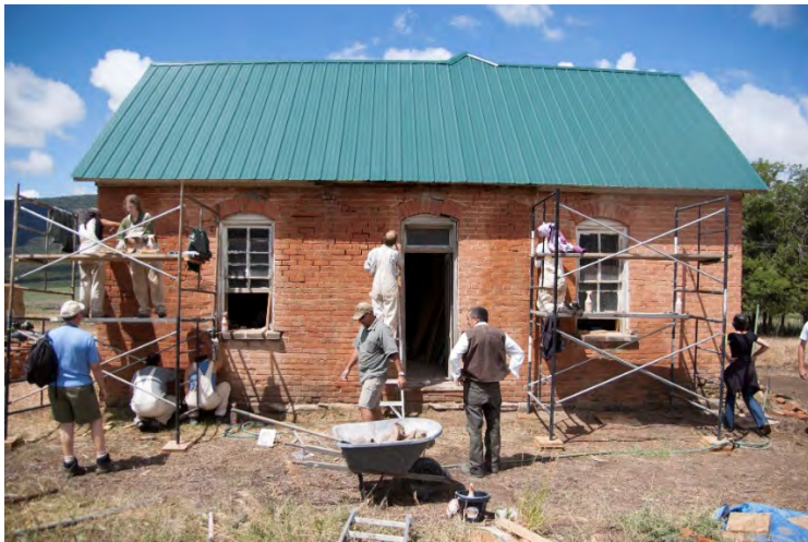
The team working on the Eastern façade of the Smith Homestead, 2014
