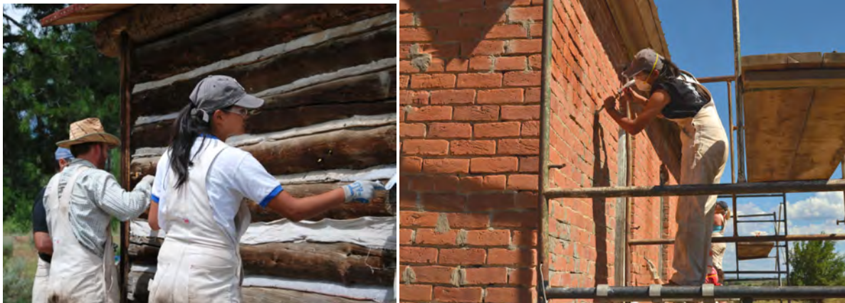
Applying new mortar chinking at Bar BC Dude Ranch in Grand Tetons, WY (left), removing cementitious parging at the Smith Homestead in Mancos, CO (right), 2014.
