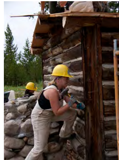
Driving reinforcement spikes into the logs of the cabin, 2014
