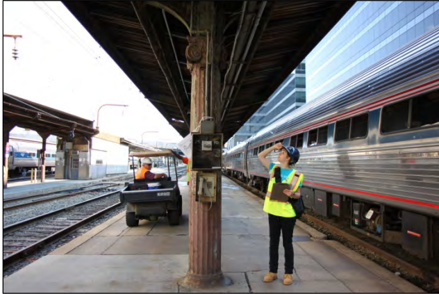
Condition Survey, Union Station, Washington, D.C., 2014
