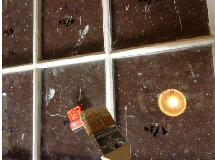
Repair and paint the historical windows, 2014
