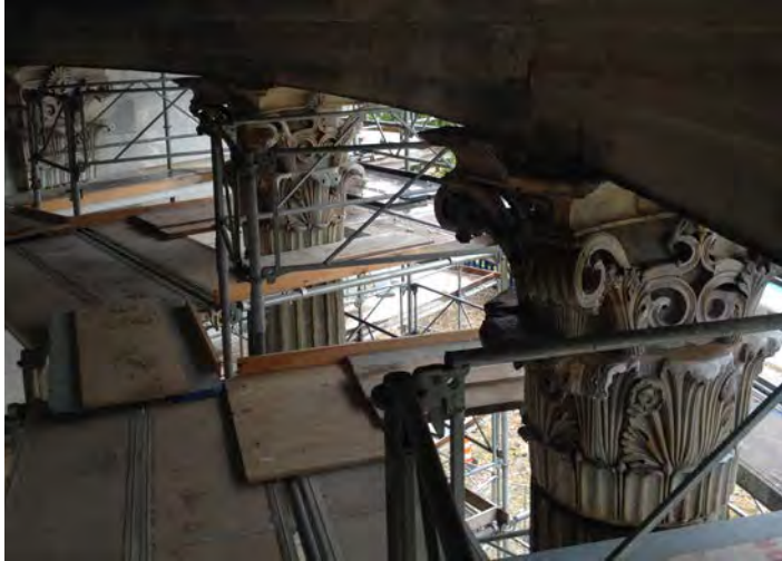
Column capitals after consolidation and cleaning, Merchants' Exchange Building, Philadelphia, PA, 2014
