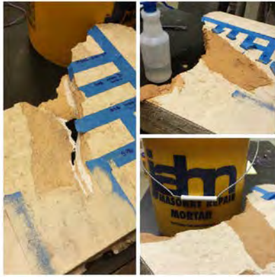
Patching a block using Jahn terra cotta repair mortar, 2014
