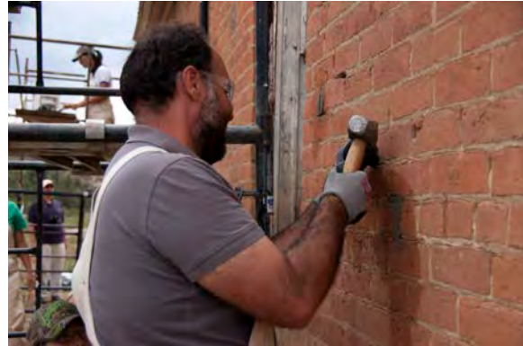
Removing cement parge at Smith's Homestead, 2014
