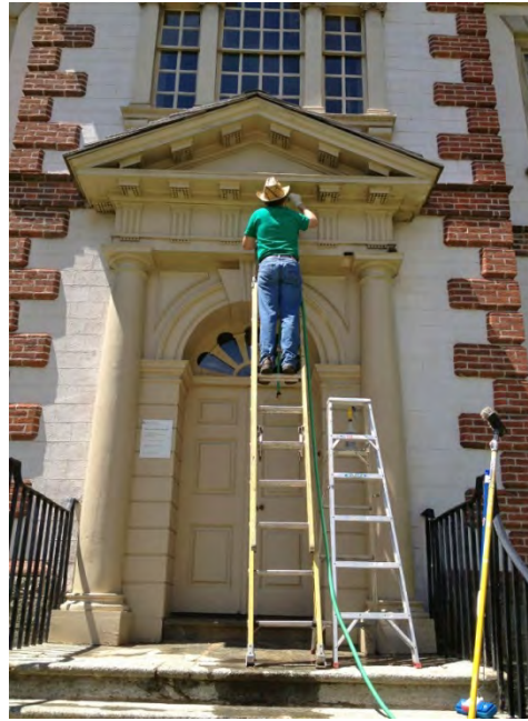
Mortar repointing of Smith farmhouse, August 2014
