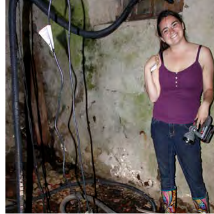
Fixing the sump-pump at a revolving fund property, 2014
