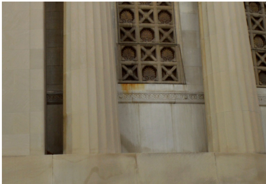
Figure 4.1.14 Isolated iron stain on below east elevation grille. (S. Loos)
