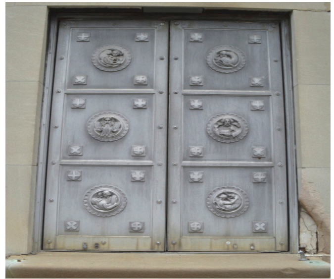
Figure 1.1 - Patina on aluminum doors and soiling around doors on southeast elevation.
