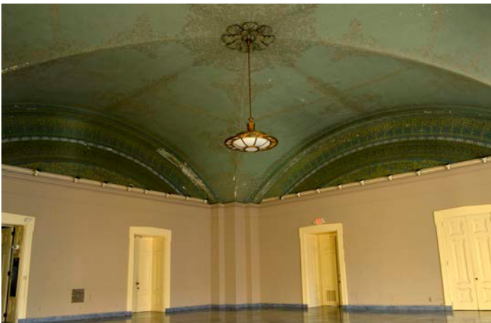
Figure 1.4.13 Southwest room. (S. Loos)
