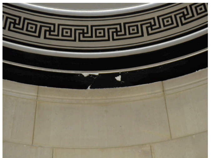
Figure 1.1 - Cracking and loss of material on ceiling in southwest rotunda.
