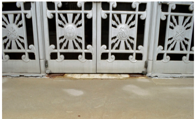
Figure 1.1 - Corrosion on entrance doors on northwest elevation.
