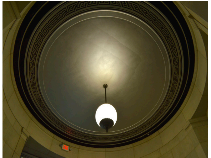
Figure 1.1 - Peeling paint around light in rotunda.
