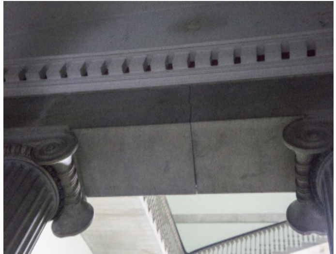
Figure 1.1 - Crack in marble beam in north vestibule.
