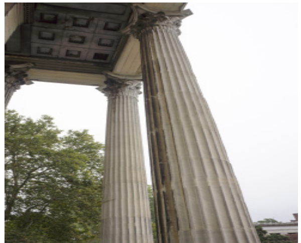
Figure 1.1 - Interior soiling on columns and coffers on south elevation.
