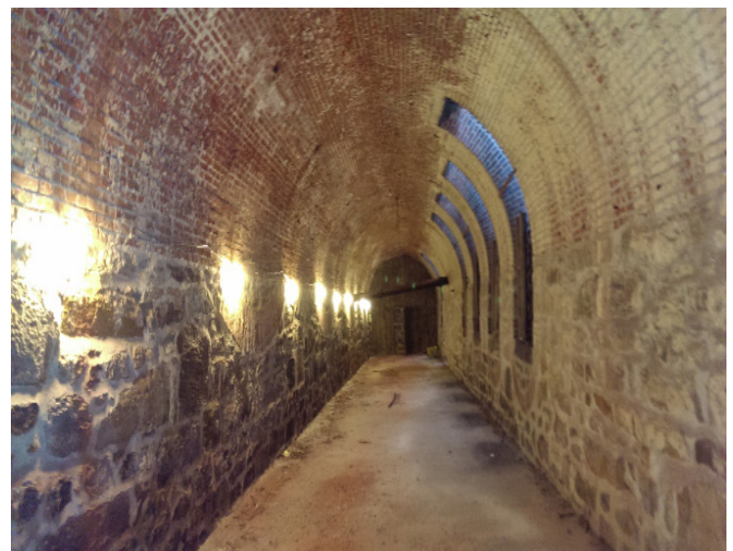
Figure 1.1 - Brick deterioration and loss of whitewash in basement.
