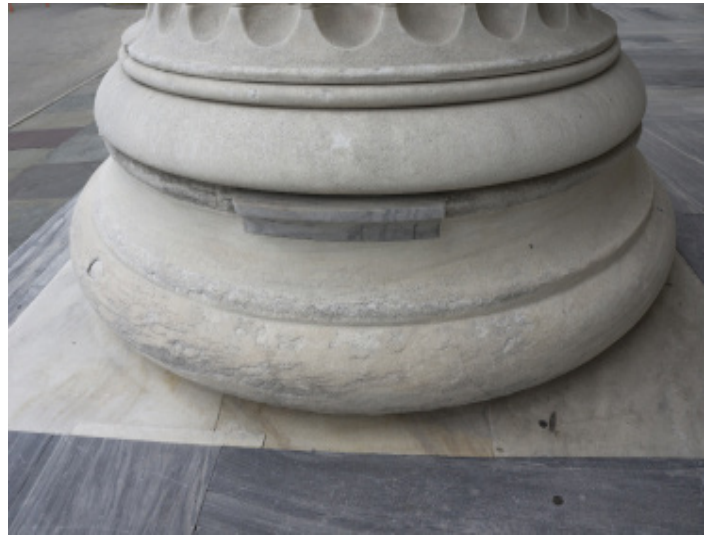
Figure 1.1 - Dutchman repair on south elevation.
