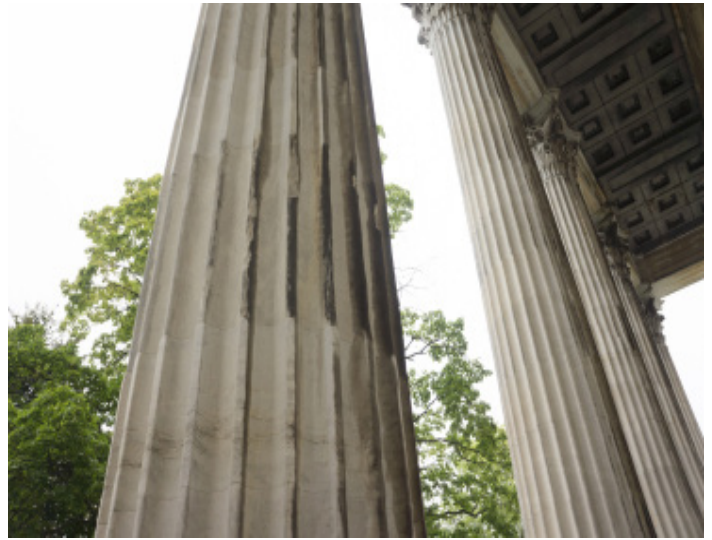
Figure 1.1 - Biogrowth, soiling, and chipping on columns on west elevation.
