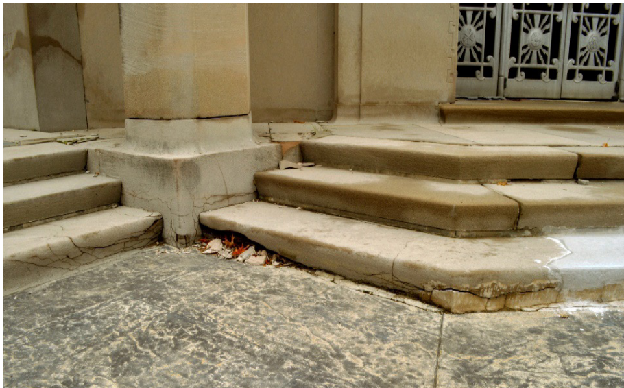
Figure 4.1.11 Cracks, voids and lost mortar on northwest main entrance stairs. (S. Loos)
