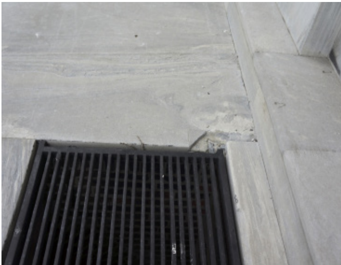
Figure 1.1 - Cracked marble paving stones on portico on north elevation.
