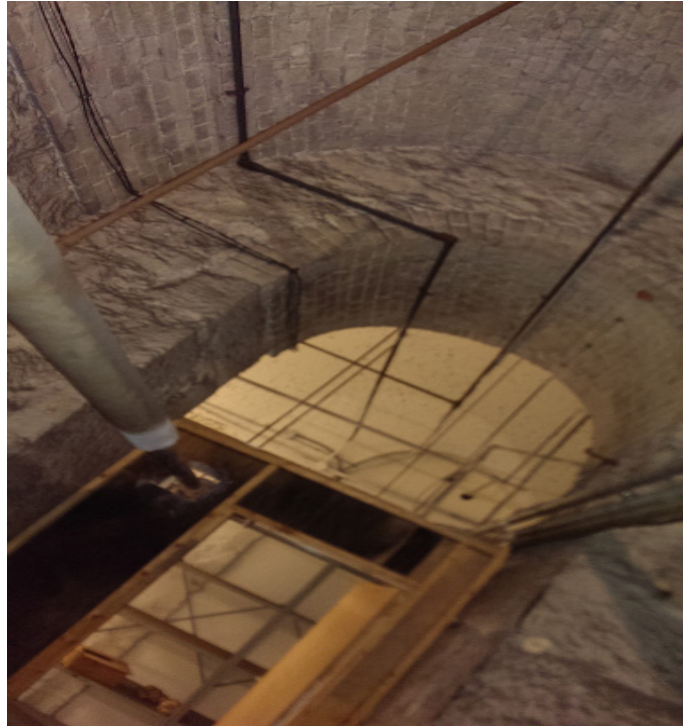
Figure 1.1 - Pipes running through basement.
