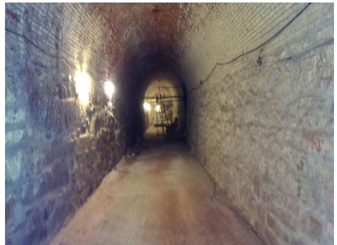
Figure 1.1 - Basement with brick barrel vaults and rubble fill.
