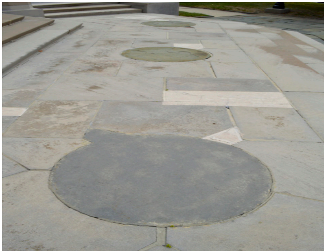
Figure 1.1 - Cracked ghost circles and chipping on landing on southwest elevation.
