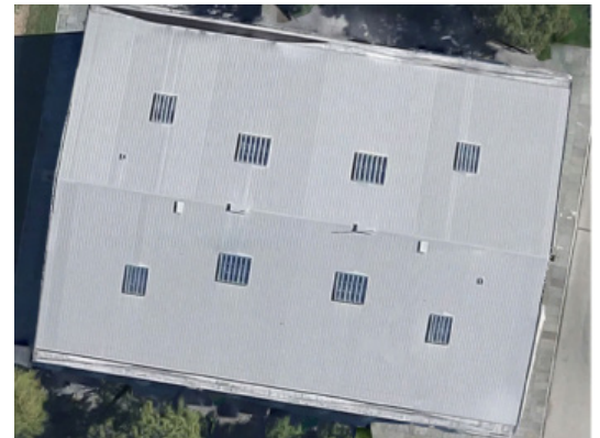
Figure 1.1. Metal roof on Founder's Hall.
