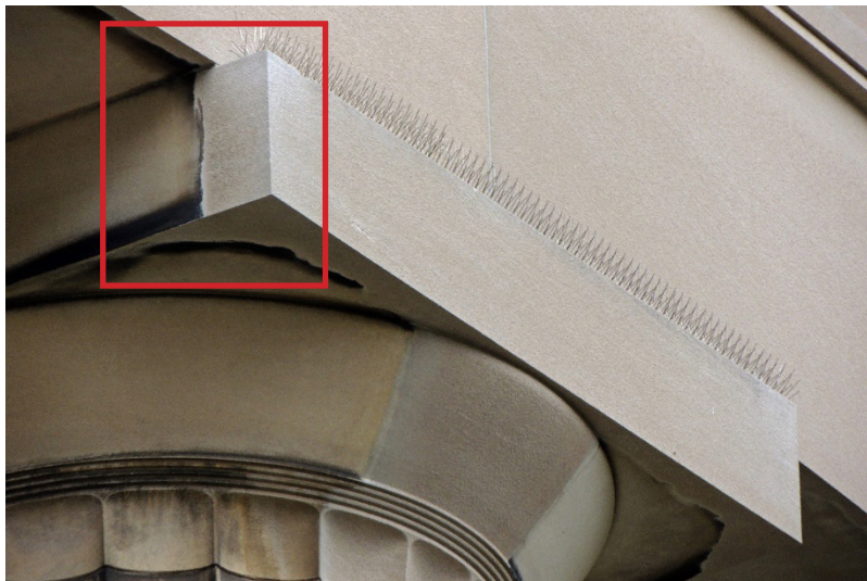
Figure 4.1.1 Original stone finish (left) and eroded surface. (right) (S. Loos)
