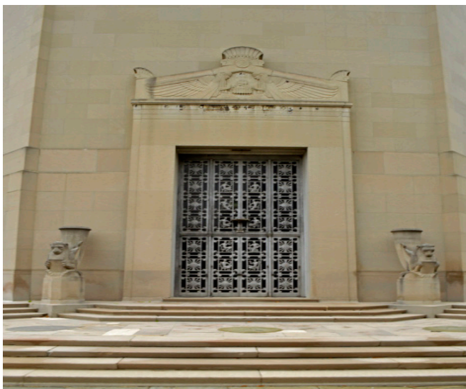
Figure 1.1 - Chipping around jamb and lintels of entrance on southwest elevation.
