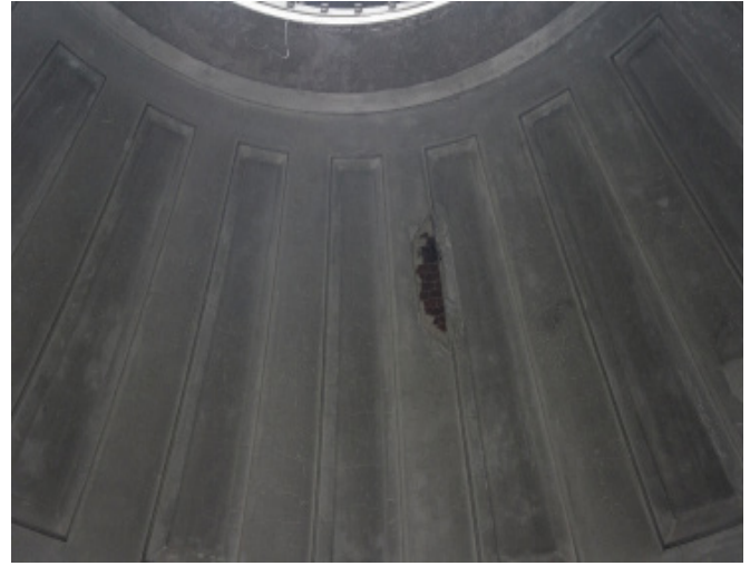
Figure 1.1 - Exposed brick framing in room 303.
