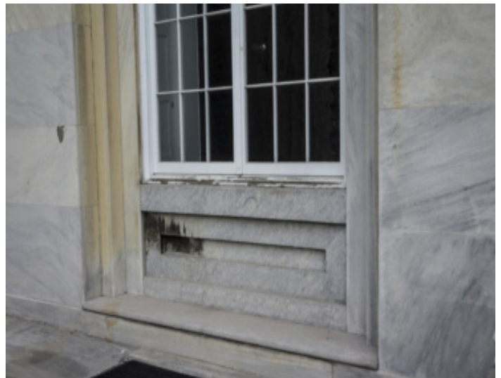
Figure 1.1 - Soiling below window on west elevation.
