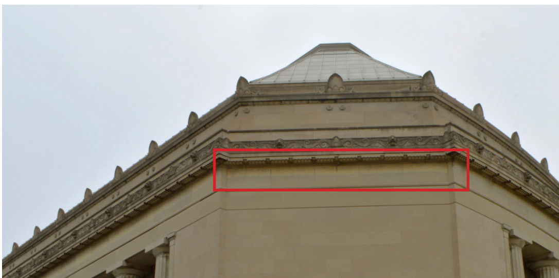
Figure 4.1.7 Band of coloration below first cornice. (S. Loos)
