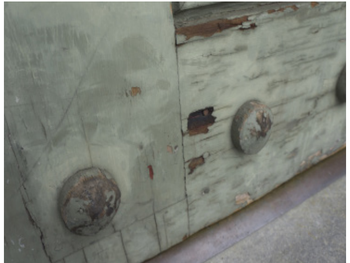
Figure 1.1 - Rot at bottom of door on south elevation.
