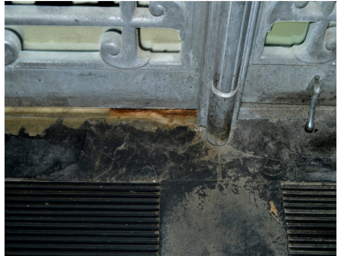
Figure 1.1 - Rusty metal and deterioration of stone work at northwest entrance.
