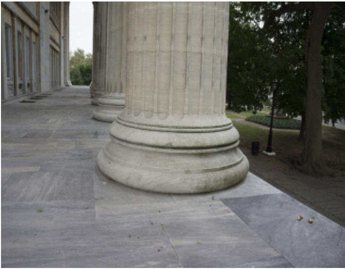
Figure 1.1 - Biogrowth on columns on east elevation.
