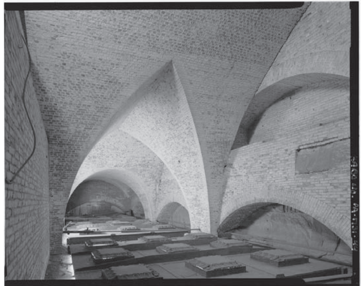
Figure 1.6.13 Attic above portico. (HABS)
