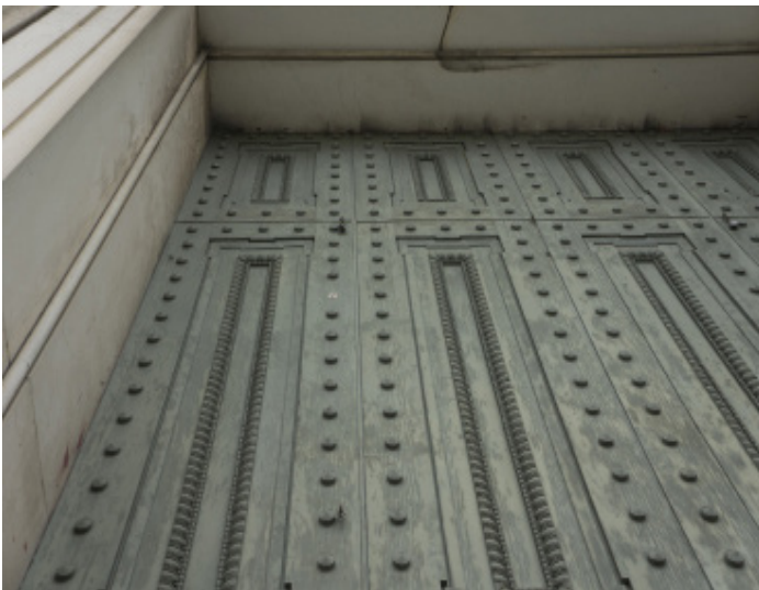
Figure 1.1 - Cracked lintel above door on south elevation.
