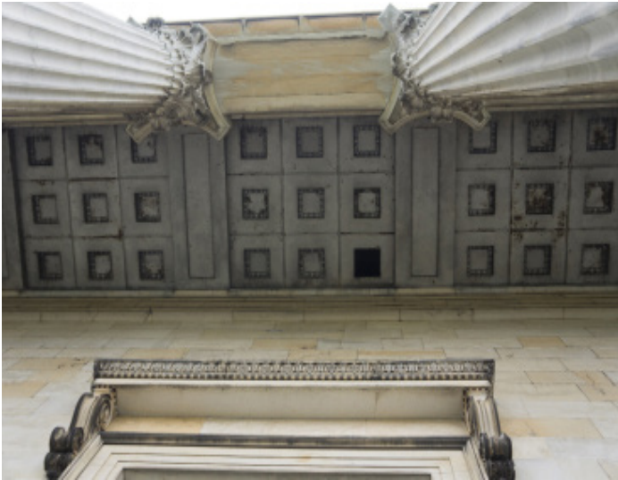
Figure 1.1 - Missing tile from ceiling over portico on north elevation.
