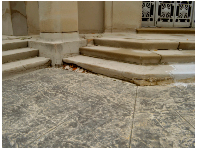
Figure 1.1 - Cracks and minor repairs to stairs on northwest elevation.
