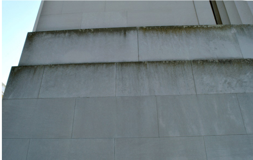
Figure 4.1.4 Biogrowth on north elevation. (S. Loos)
