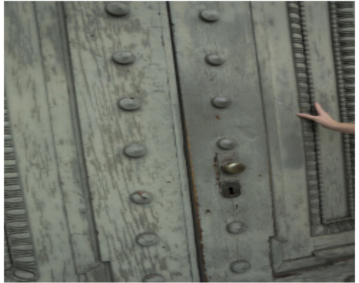
Figure 1.1 - Peeling, cracking and chipping paint on door on south elevation.
