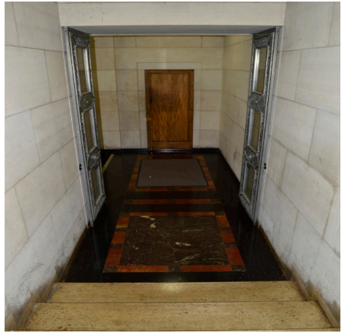
Figure 1.1 - Wax staining and stair wear in south hallway.
