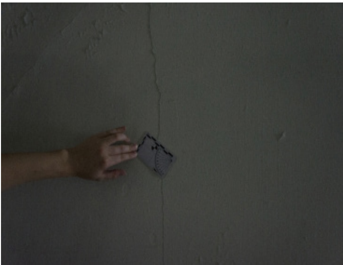
Figure 1.1 - Representative of plaster cracks in north and south halls.
