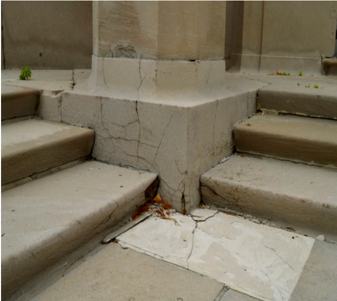
Figure 1.1 - Cracking on base of St. Mark Lion statue on southwest elevation.
