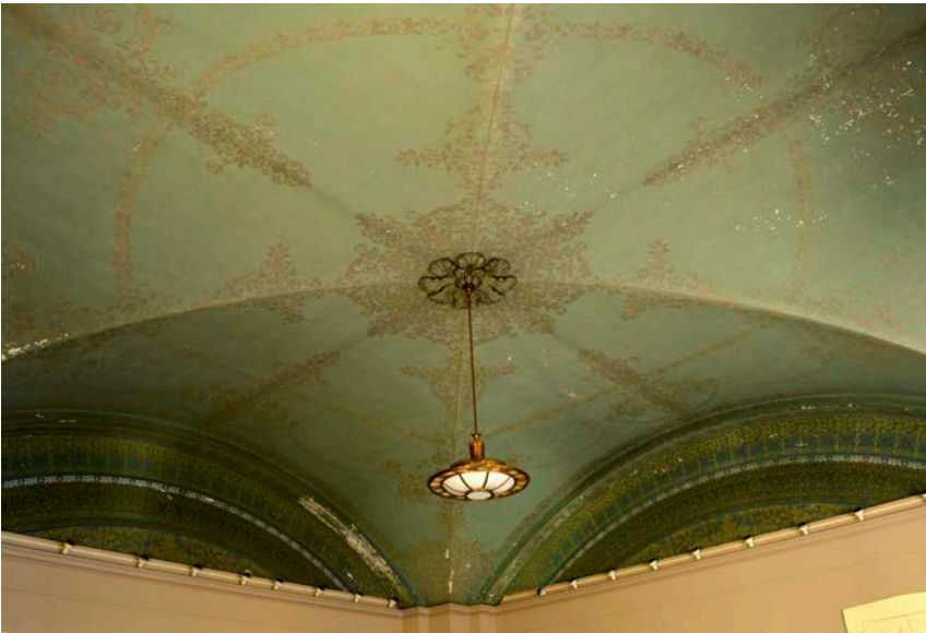
Figure 1.6.12 Southwest room, 1st floor.(S. Loos)
