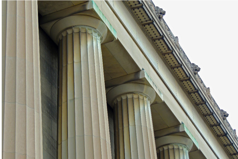
Figure 4.1.13 Copper staining on columns of south elevation. (B. Winter)
