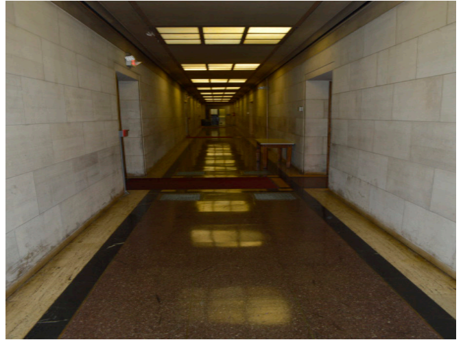
Figure 1.1 - Wax staining at base of stone walls in southeast ambulatory.
