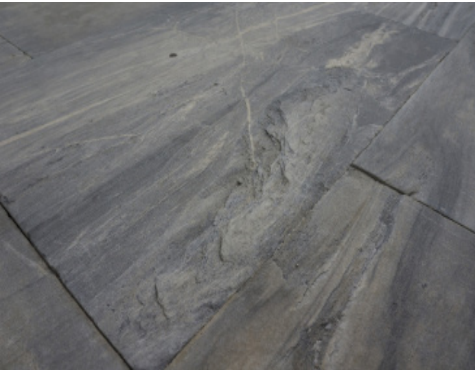
Figure 1.1 - Delamination of marble paving stones on portico of north elevation.
