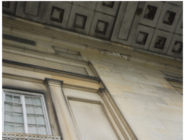
Figure 1.1 - Biogrowth, coloration, and bird guano on east elevation.
