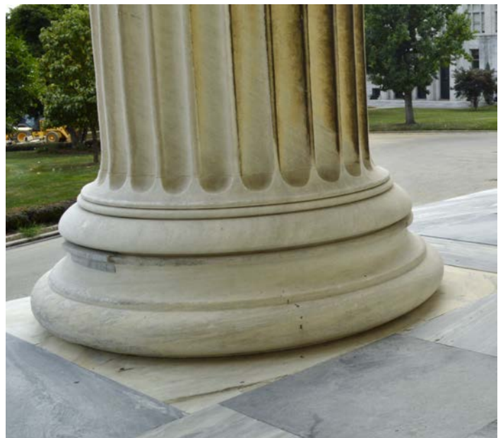
Figure 1.4.5 Column base, south elevation. (S. Loos)
