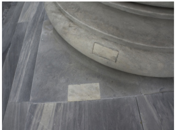
Figure 1.1 - Dutchman repair on west elevation.
