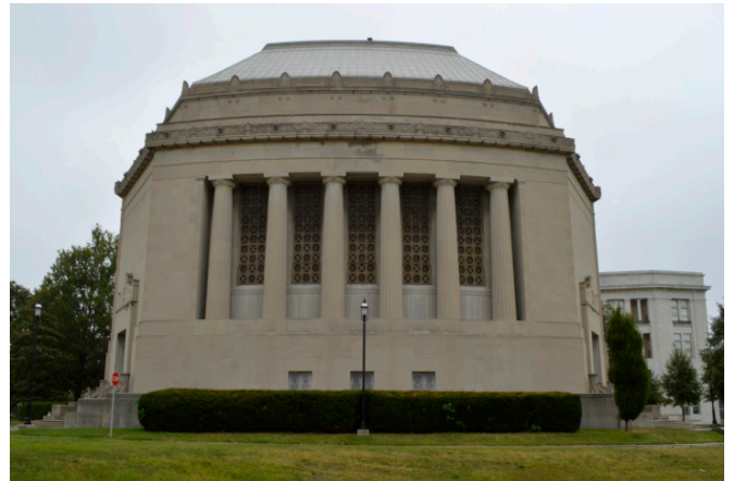
Figure 1.1 - Deterioration of west elevation.
