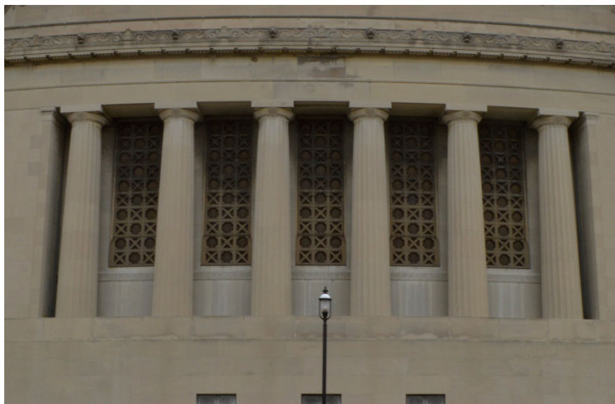
Figure 4.1.6 Bleaching below bronze grilles on west elevation. (S. Loos)
