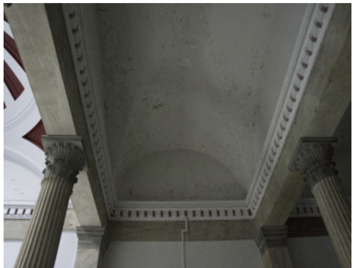
Figure 1.1 - Representative of peeling paint in third floor halls.
