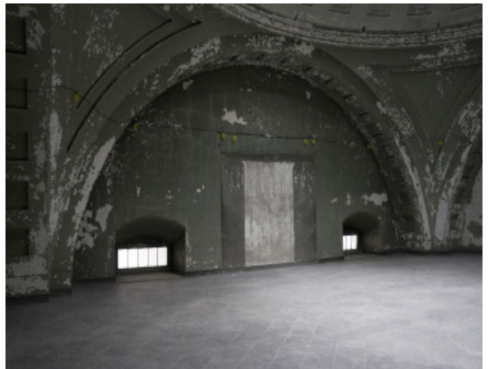
Figure 1.1 - Peeling paint and damaged plaster in room 305.
