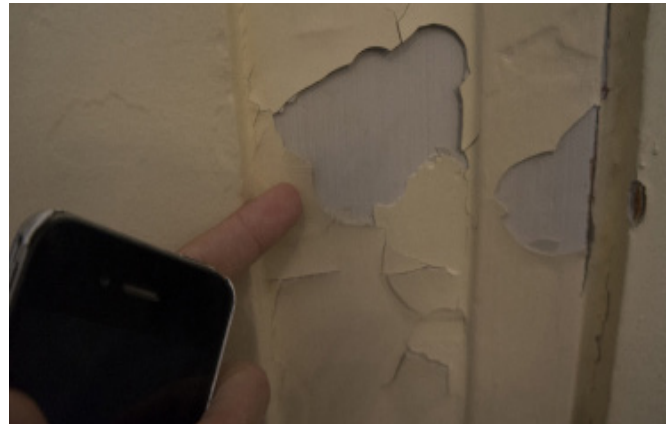
Figure 1.1 - Representative of layers of paint on interior doors.
