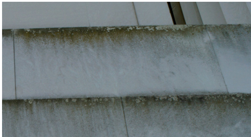
Figure 4.1.5 Biopitting on north elevation. (S. Loos)
