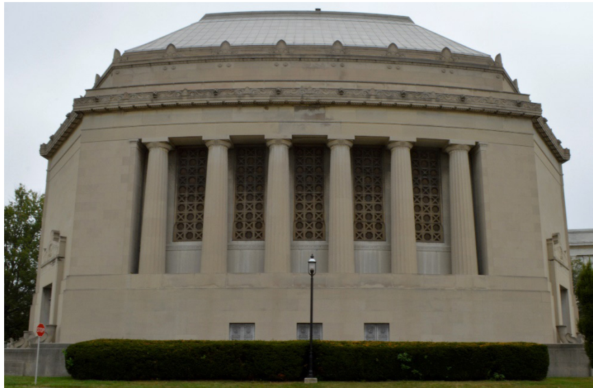
Figure 4.1.2 Soiling on the Chapel base, grilles and cornices of south elevation. (S. Loos)
