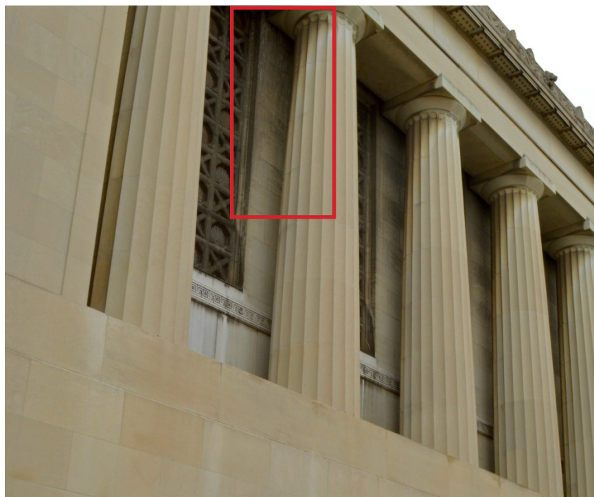
Figure 4.1.8 Bird excrement on wall behind colonnade of south elevation. (S. Loos)
