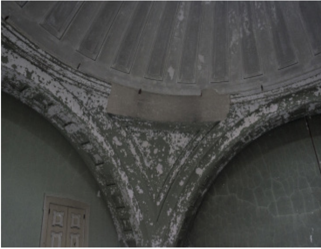
Figure 1.1 - Section of plaster removed from dome in room 303.
