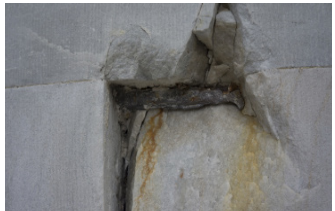
Figure 1.1 - Marble bursting and rusted iron fastener visible on south elevation.
