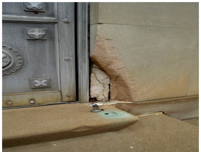
Figure 1.1 - Abrasive damage to limestone at base of side door on southeast elevation.
