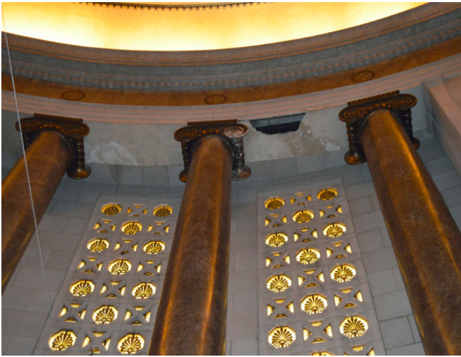
Figure 1.1 - Missing plaster above columns and possible evidence of water damage behind the stage.
