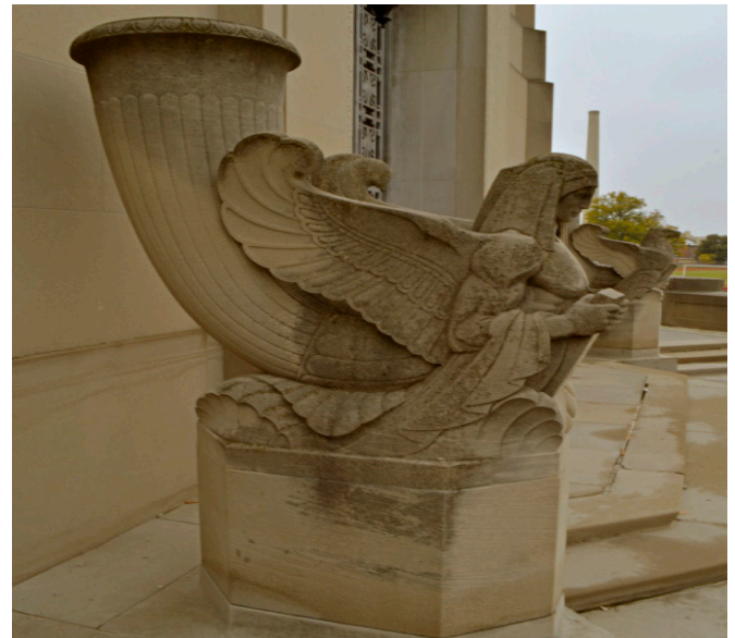
Figure 1.1 - Biogrowth on statues by entrance on northwest elevation.
