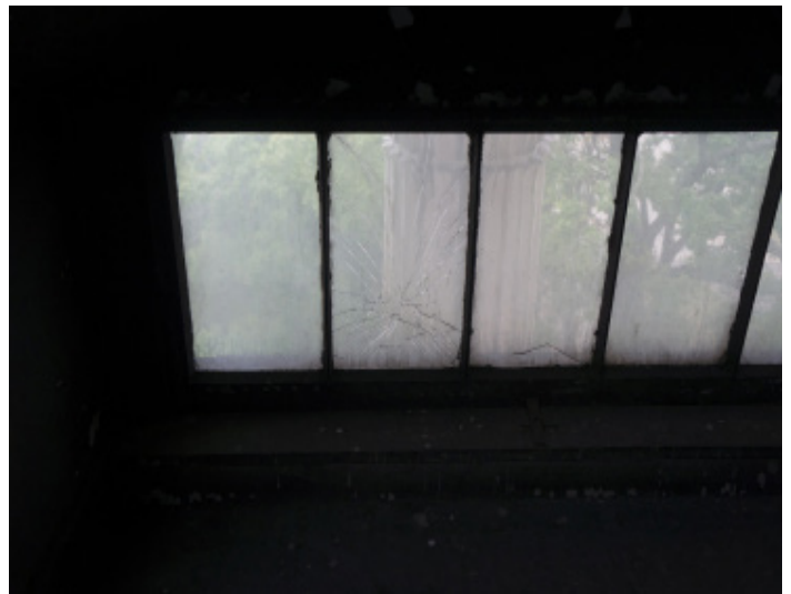
Figure 1.1 - Cracked window pane in room 305.
