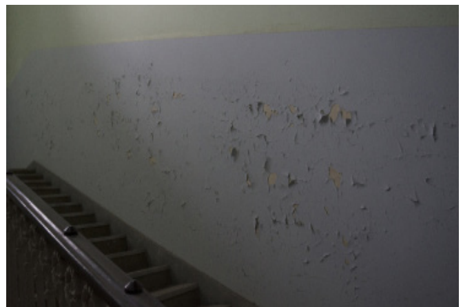
Figure 1.1 - Representative of peeling paint around staircase.
