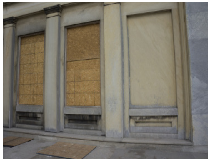
Figure 1.1 - Windows being restored on east elevation.
