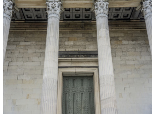
Figure 1.1 - Soiling on south elevation.
