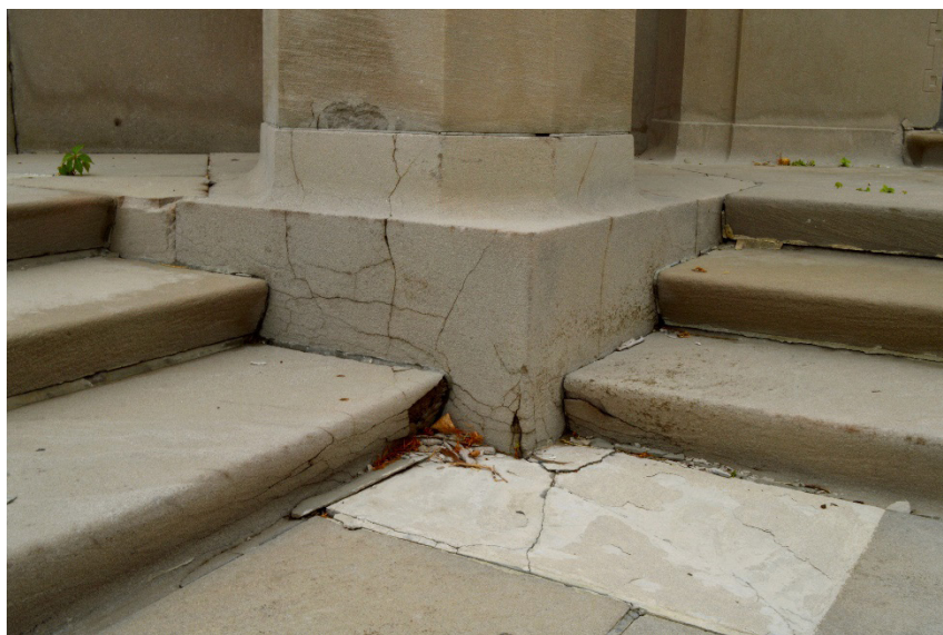
Figure 4.1.12 Cracks, voids and lost mortar on southwest main entrance stairs. (S. Loos)
