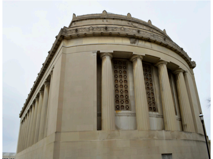
Figure 1.1 - Rust staining below southernmost window on southeast elevation.
