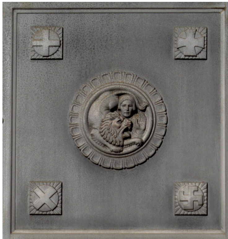
Figure 4.1.15 Representative shot of patina and spotting of aluminum. (S. Loos)
