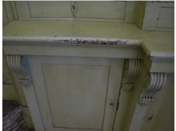
Figure 1.1 - Peeling paint on bookshelves in Board Room.
