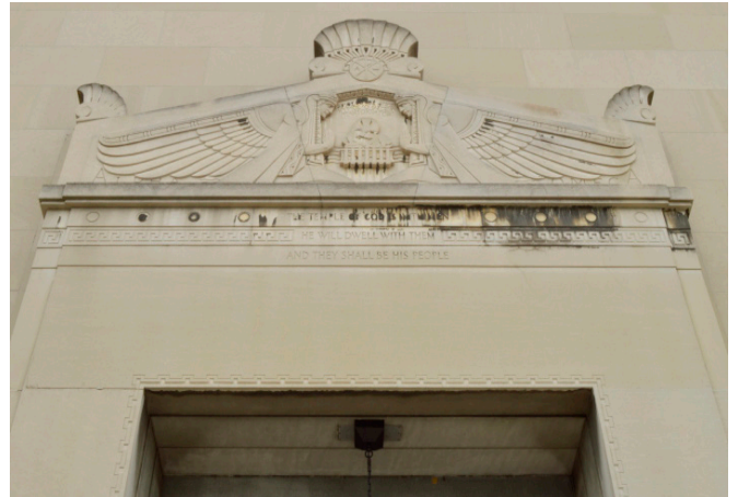
Figure 1.1 - Biogrowth on pediment above entrance on northwest elevation.
