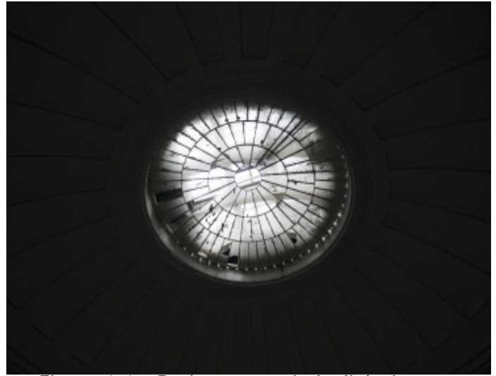
Figure 1.1 - Broken panes in laylight in room 306.
