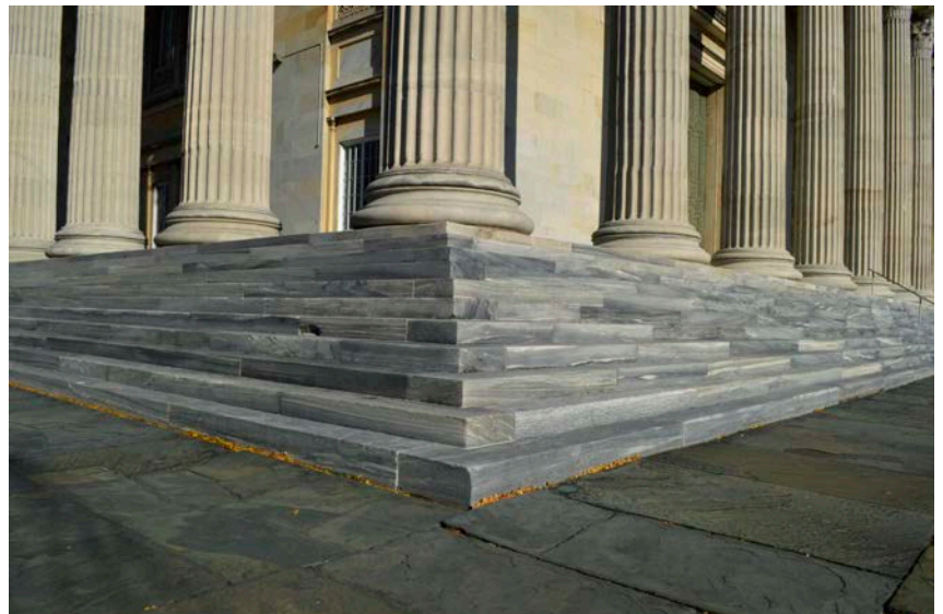
Figure 1.6.20 Southwest corner. (S. Loos)
