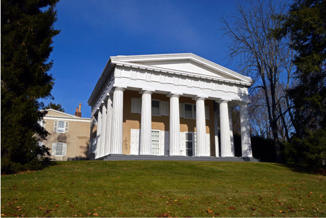
Figure 5.10.1 Portico on east elevation of the Big House. (S. Loos)
