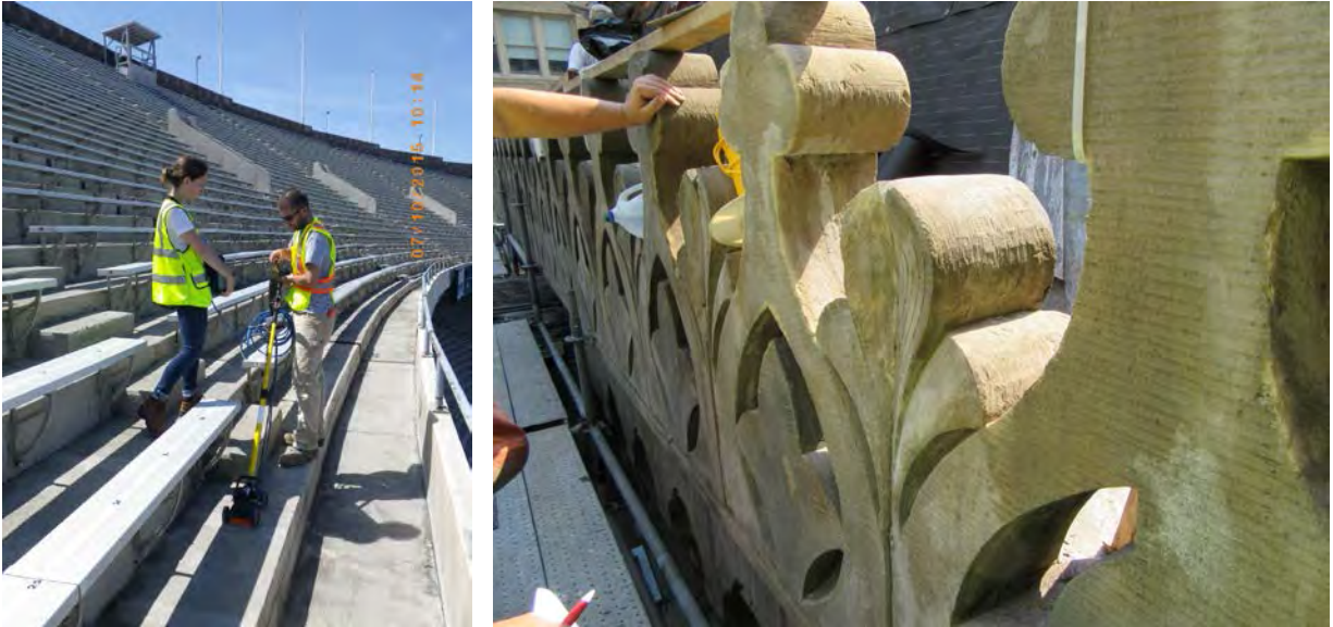
(Left) Collecting sound penetrating radar data, 2015. (Right) Reviewing stone cleaning mock ups, 2015.
