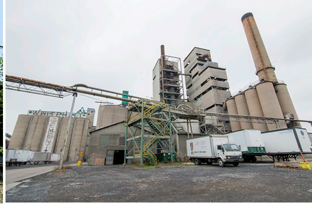
Lafarge (Whitehall) Cement, 2015
