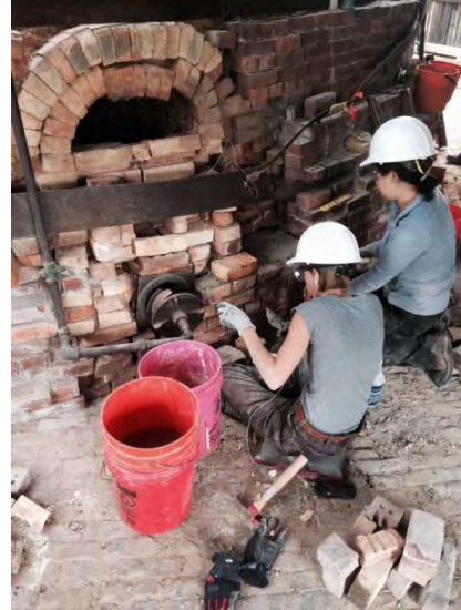
Repointing the kiln wicket, 2015
