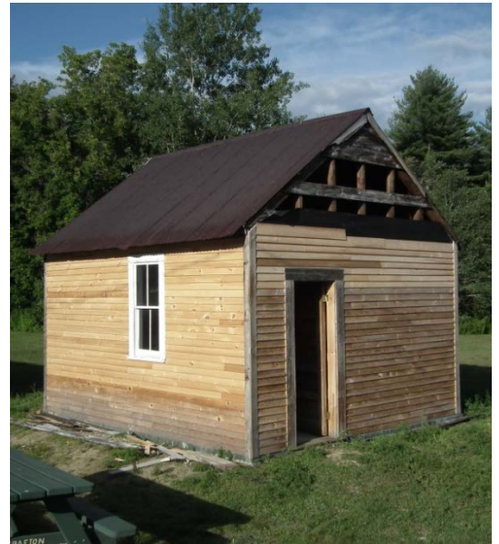
Residing and re-sheathing the tramp house, 2015
