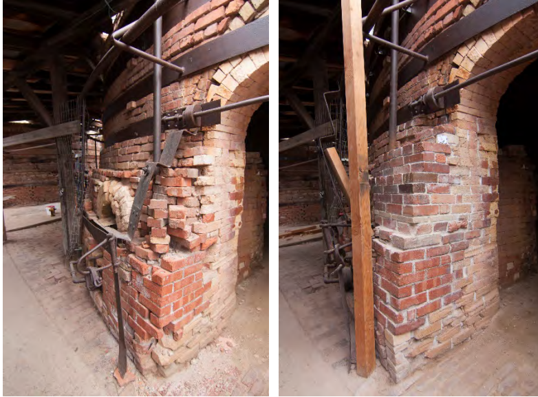
Before (left) and after (right) stabilization treatment on an entrance of the Kiln 7, 2015
