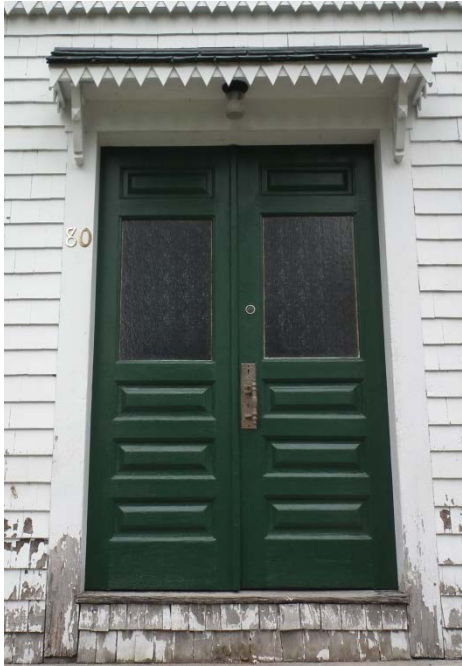
The fresh doors made the rest of the church look not-so-fresh, 2015
