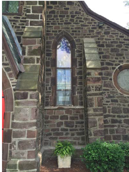
Figure 7: Brownstone composite patching at All Saints’ Torresdale Episcopal Church (1855), Edison Coatings with mica aggregate amendments.
