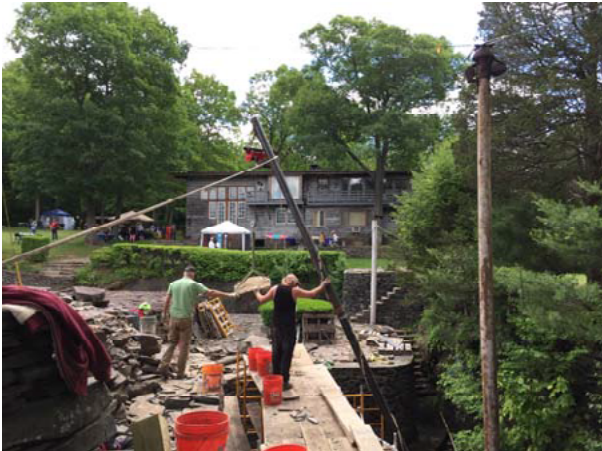
Figures 16 & 17: Opus 40 , wall restoration with the help of a gin-pole.
