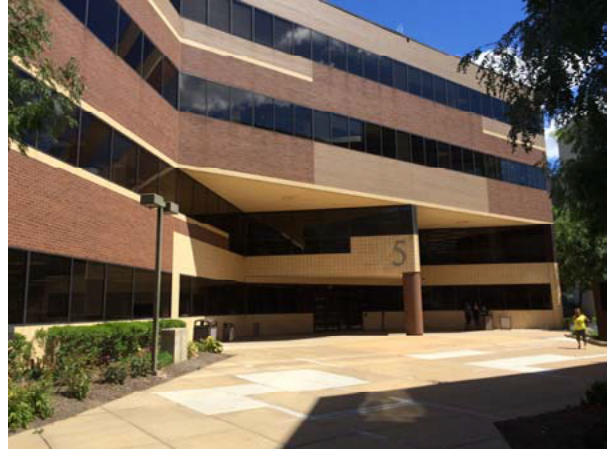
501 E State Street, home of the NJHPO, 2016.
