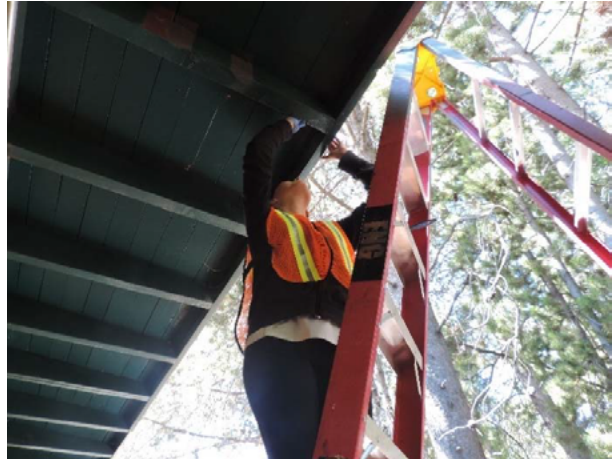
Retrieving a paint sample from a wooden rafter at one of the outbuildings (cabins), 2016.
