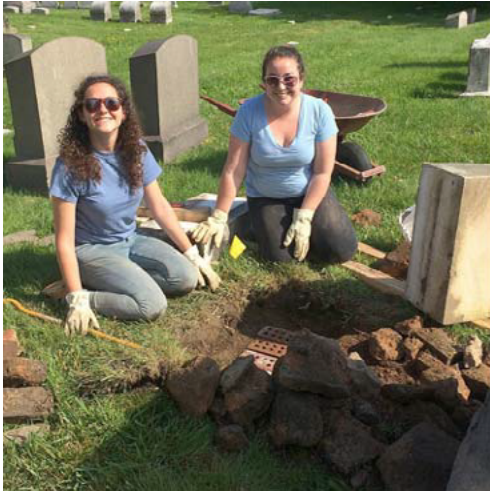
Summer interns Lucy Midelfort and Danielle Pape relaying new brick foundations for misaligned grave markers.
