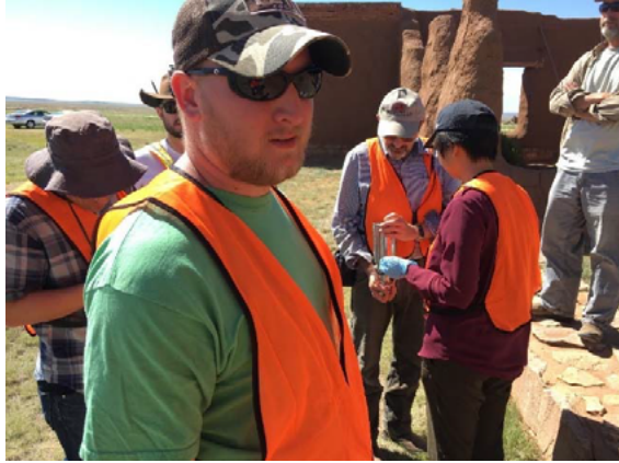
The team conducting moisture meter testing on the adobe walls. 2016.
