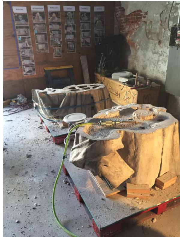
Figures 10 & 11: Removal of cementitious mortar from Mr. Caldwell & others with pneumatic driven carbide tipped chisels.
