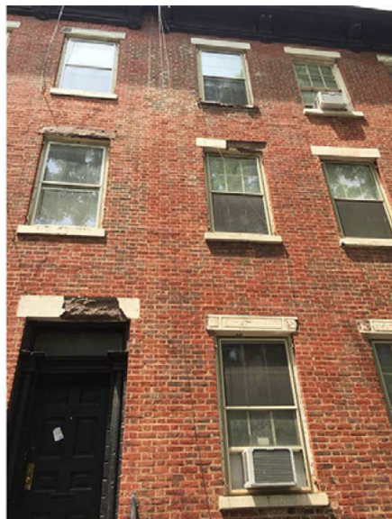
The deteriorating windows and brownstone lintels being documented in the survey, 2016.
