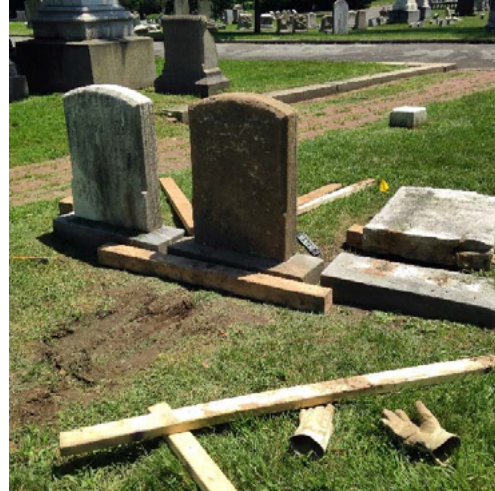
A marble headstone that had to have the corroded pins removed and reset.
