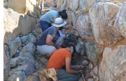
Repointing walls at Mochlos, 2016.
