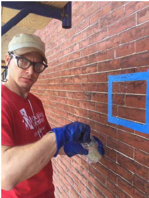
Figures 5 & 6: Mock-up and testing cleaners for atmospheric pollutants. 2041 Delancey scaffold ready for work.
