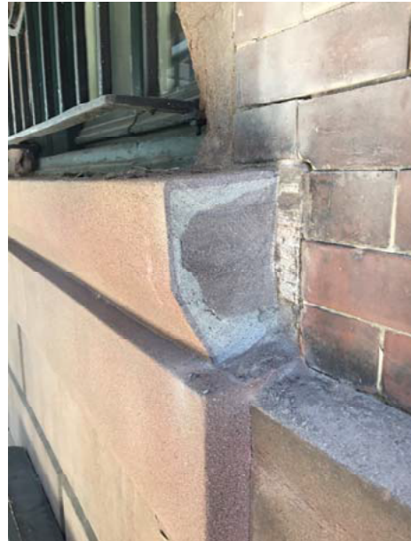
Figures 3 & 4: Prepared Samples of Composite Patches for Brown Stone & Building Archaeological Investigation of Mouldings at 2041 Delancey Street, Philadelphia.
