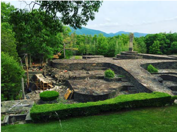
Figures 16 & 17: Opus 40 , wall restoration with the help of a gin-pole.
