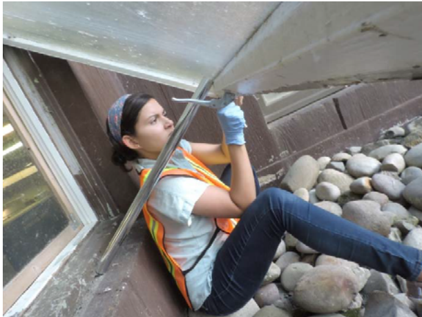
Taking a paint sample from an original window sash at Jackson Lake Lodge, 2016.
