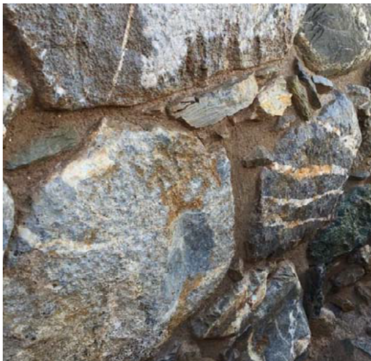
A freshly repointed wall of Ave. 2. Mochlos, 2016.
