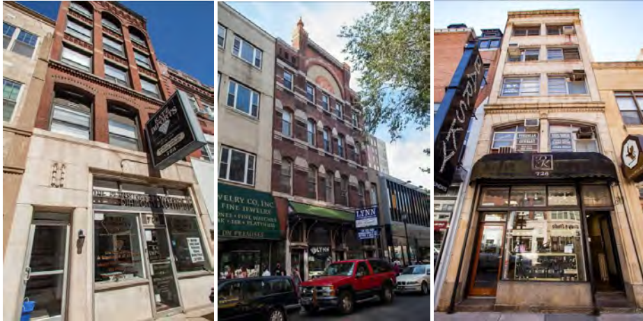
Left to right: View of an art deco storefront modification to the late 19 th century building at 723 Sansom; A late Victorian façade remodel at 706-08 8 th that unified two existing properties; five-story terra cotta commercial building at 726 Sansom. Photos: Starr Herr-Cardillo, 2016.
