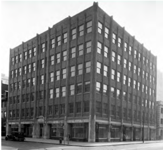
The Neff Building at the southeast corner of 8th and Sansom circa 1931, courtesy of City of Philadelphia Department of Records
