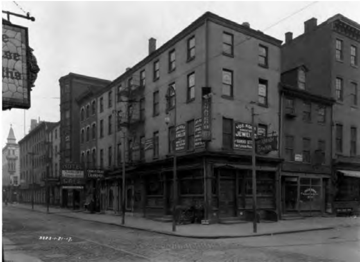
View of the northeast corner of 8th and Sansom circa 1917, courtesy of City of Philadelphia Department of Records
