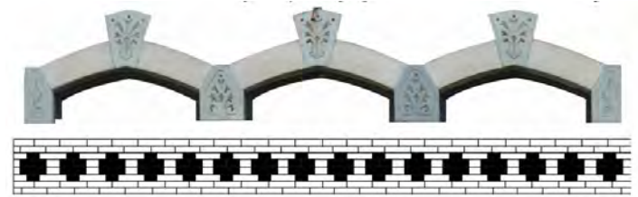
Figure 11: (Upper) Stone tripartite lintel. (Lower) polychromatic brickwork design of 710.
