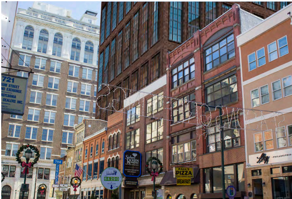
Brick Toll Bros. Tower - With facadectomy
