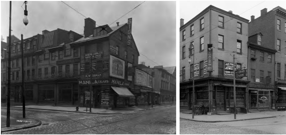
These 1917 photos of the southeast and northeast corner of 8 th and Sansom, respectively, show the slow architectural evolution of the street from domestic to primarily commercial use. Photos courtesy of the City of Philadelphia Department of Records.
