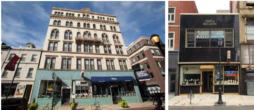
Left to right: The Press Building at 701-07 Sansom with its mid-century aqua tile storefront; The Testa Building at 126 S. 8 th Street was refaced in opaque black structural glass and anodized gold aluminum in the 1960's. Photos: Starr Herr-Cardillo, 2016.
