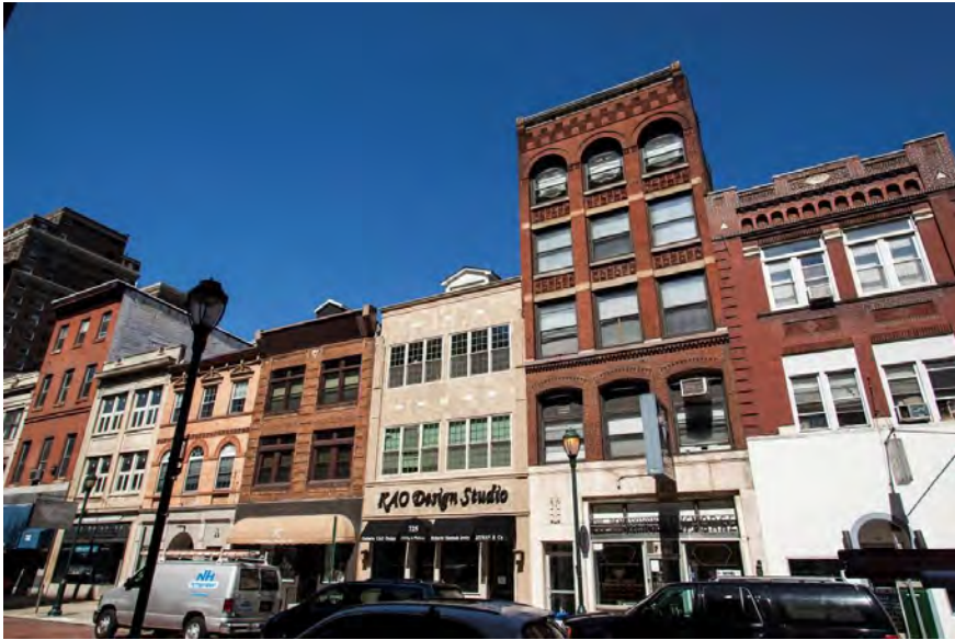
View of the north side of the 700 block of Sanso, facing northwest. Photo: Starr Herr-Cardillo, 2016.
