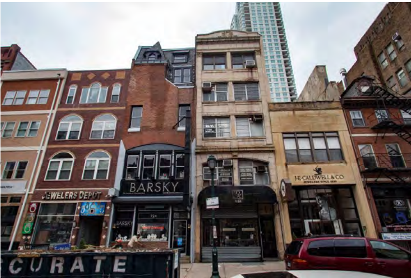
View of the south side of the 700 block of Sansom , facing south. Photo: Starr Herr-Cardillo, 2016.
