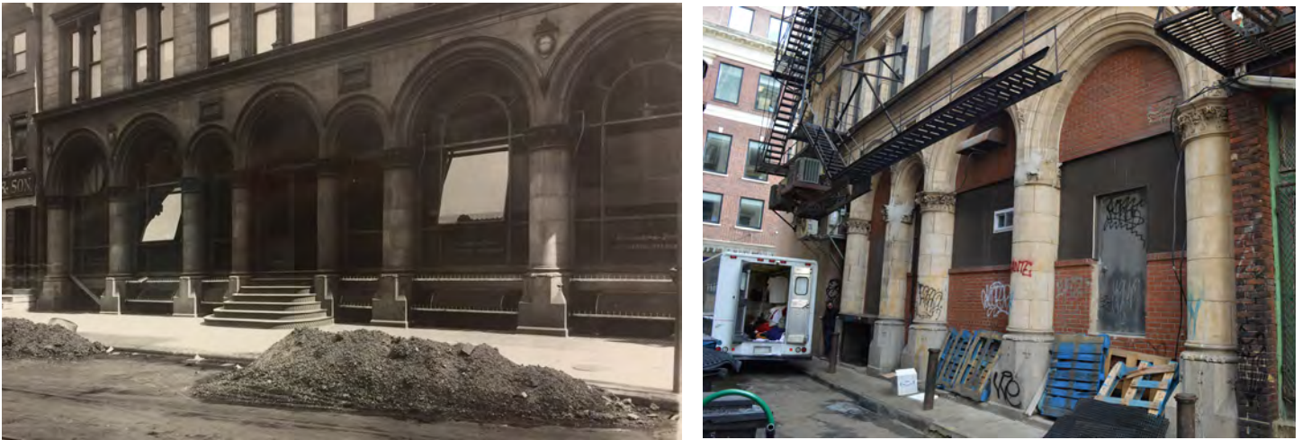
Figure 19: (Left) The front facade of the Philadelphia Press Building, 1918. (Right) The rear of the Philadelphia Press Building still intact, 2016.
