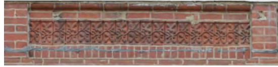
Figure 14: Detail of terra-cotta spandrel.
