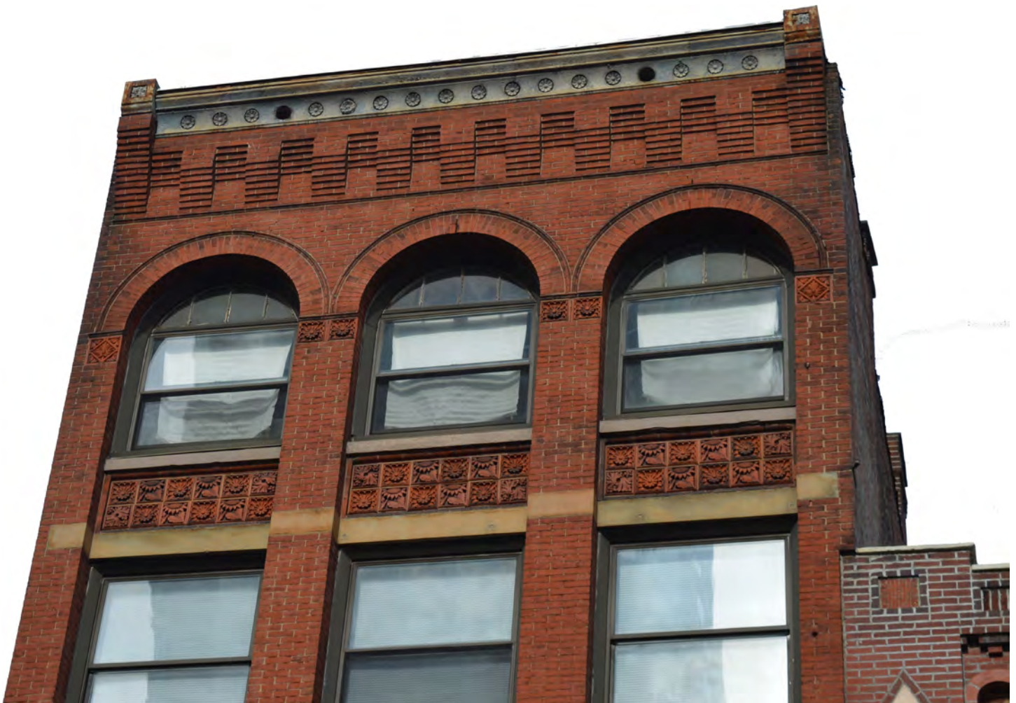
Figure 22: Front elevation, pressed tin metal cornice with floral detail pattern. 2016, Silvia Callegari.
