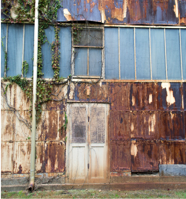
Figure 11, Exterior view, one of the small doors located at south side of 611, photo: Sh. Torkzaban, 2016
