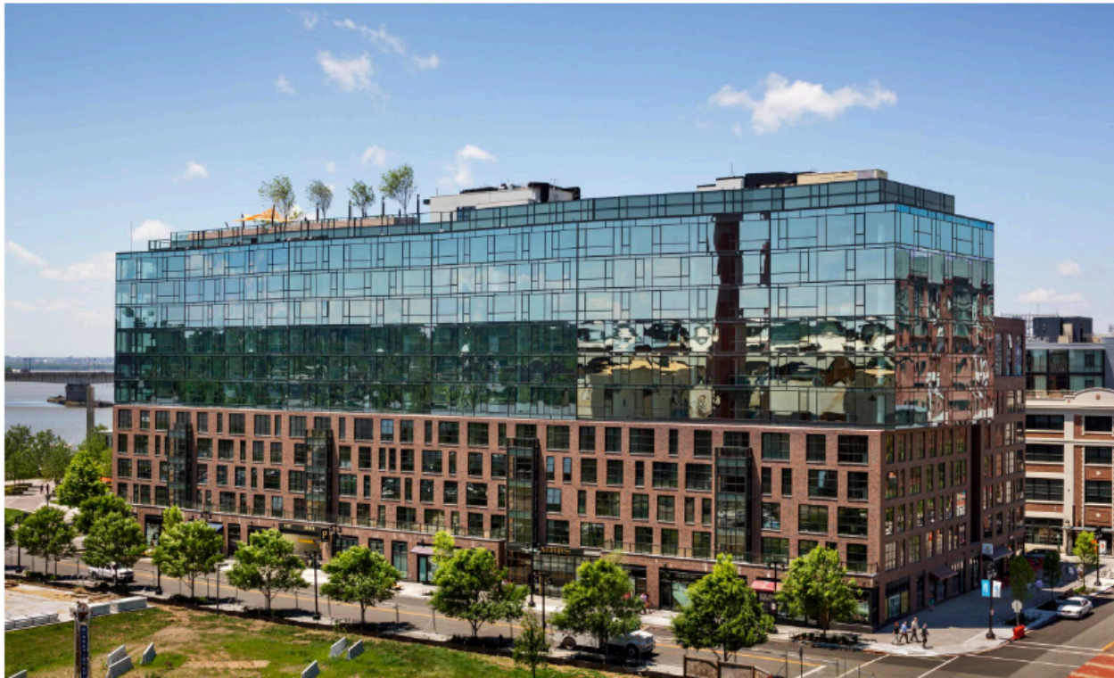
Arris Apartments, Robert A. M. Stern Architects
