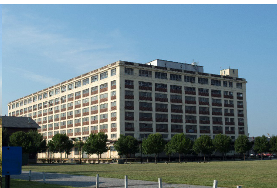
Figure 2, building 83, concrete with brick infills, photo: Z. Qin, 2016
