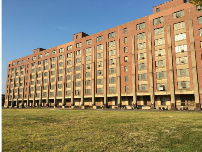
Fig. 4. Type II, Building 83. Photo by author.
