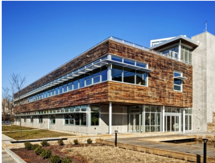
Fig. 15. LEED Certified building at the Phipps Center for Sustainable Landscape, Pittsburgh, PA. 8
