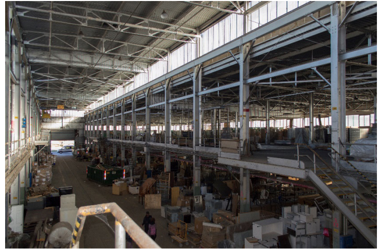
Figure 4, A general view of inside of the 611, photo: Sh. Torkzaban, 2016
