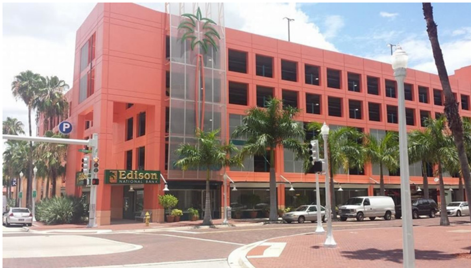
Fig. 19-20. High density parking that respond to their historic contexts. Staunton, VA and Fort Myers, FL. 1112
