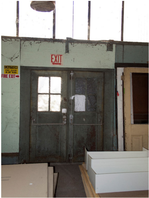
Figure 12, Interior view, one of the small doors located at south side of 611, photo: Sh. Torkzaban, 2016
