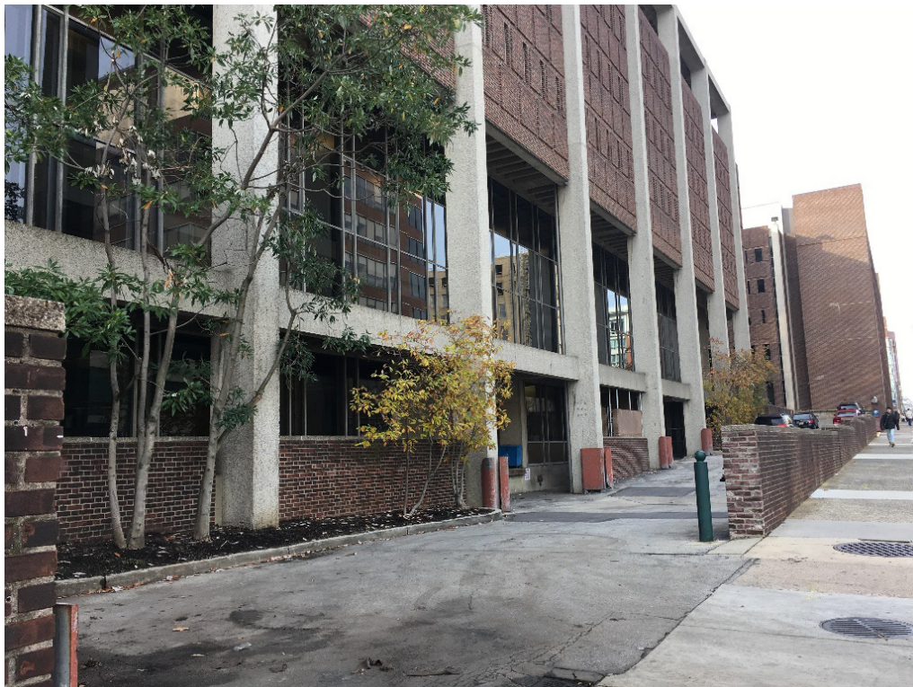
Fig. 18. Discrete vehicle loading dock, University of Pennsylvania.
