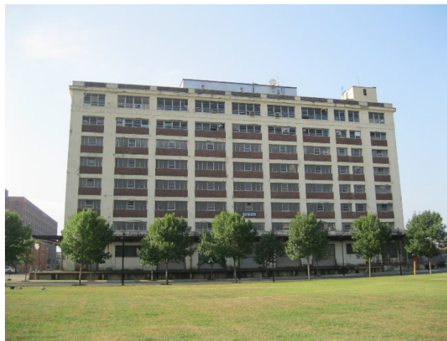
Fig. 5. Type II, Building 624. Photo by author.
