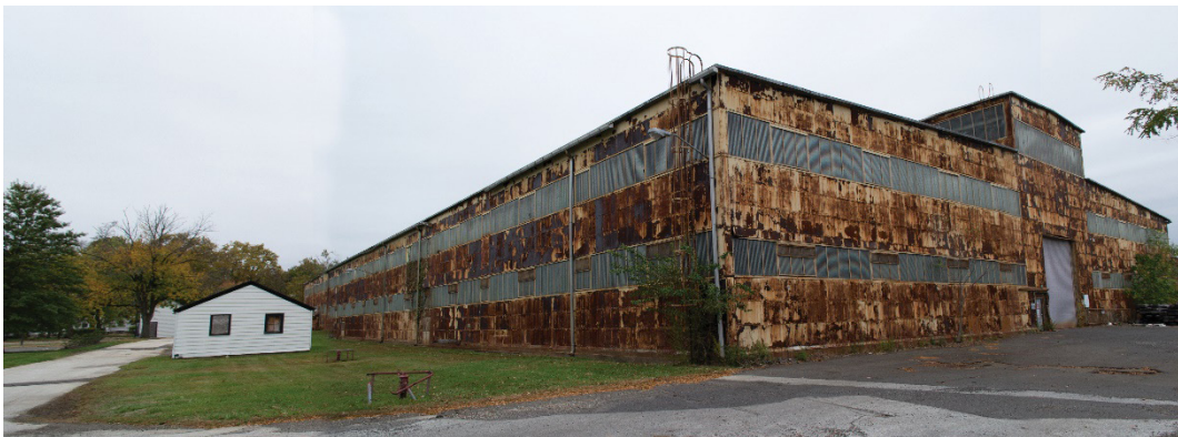
Figure 1, Building 611, metal structure, photo: Sh. Torkzaban, 2016
