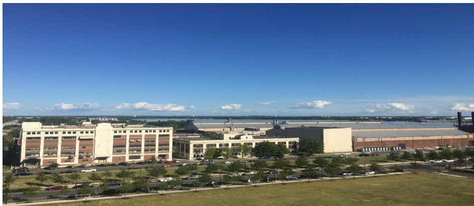
Fig. 6. Type II, Buildings bordering the Eastern Historic Core to the East. Photo by Arielle Harris.
