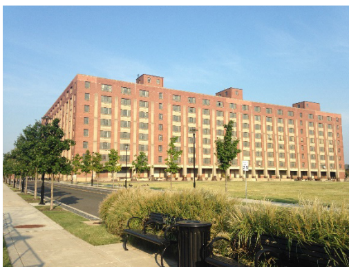
Figure 3, Building 624, concrete with brick infills, photo: Sh. Torkzaban, 2016
