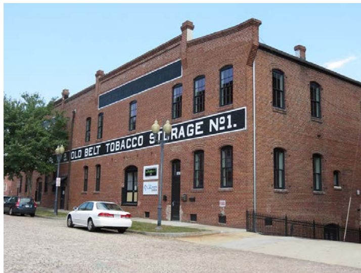
Fig. 11. An industrial building in Danville, VA, built to the lot line. 4
