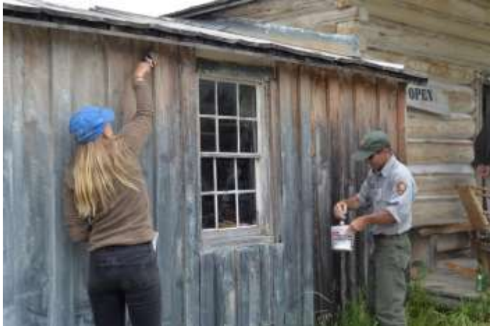
Applying lime wash to a wooden structure during a workshop about traditional finishes at Grand Teton National Park, 2017
