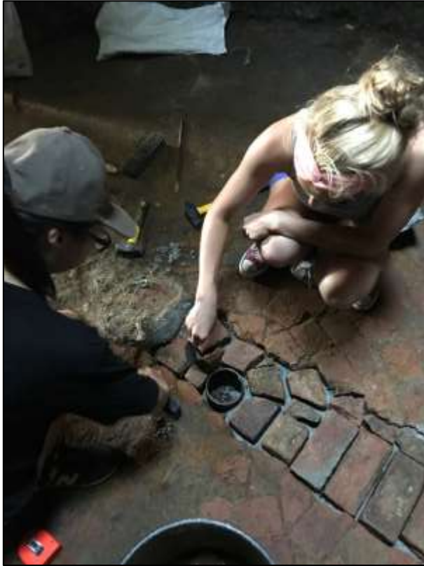
Restoring brick floor in the Root Cellar, 2017
