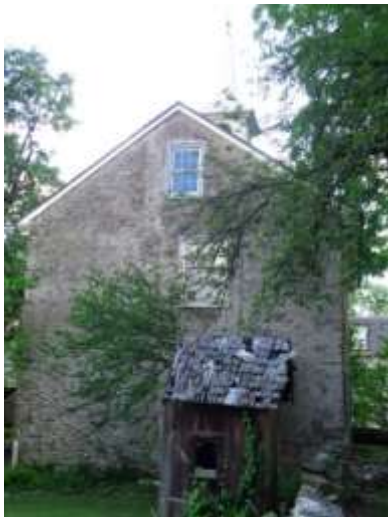
Back of the Concord Schoolhouse and the privy.
