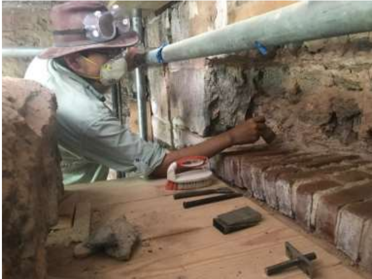
Anthony Hita working on structural masonry repairs at an Undisclosed Philadelphia landmark, July 2017
