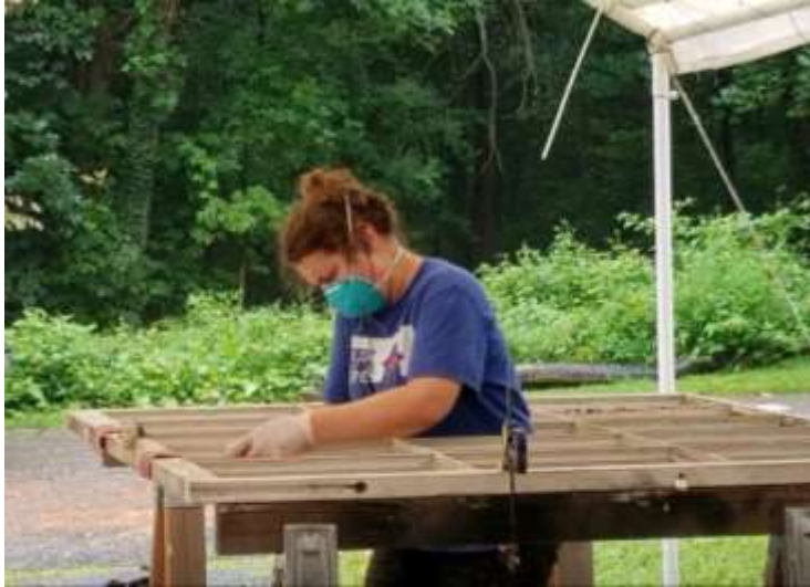
Sanding window sash from Old First, 2017
