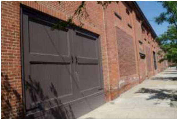
East Side of the rebuilt barn along 41 st Street, 2017
