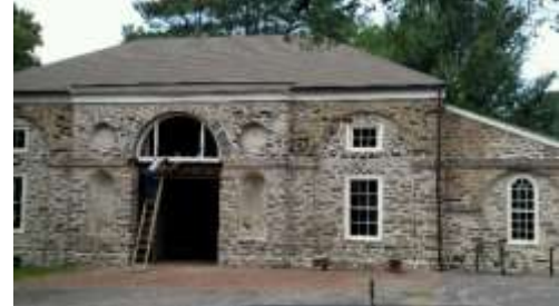
Window and Door Restoration project at The Woodlands with The Fairmount Park Conservancy, 2017
