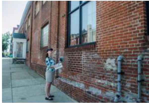
Surveying the north side of the trolley barn, along Chestnut Street, 2017
