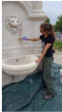
Applying a sacrificial lime wash coating at the Catholic Total Abstinence Fountain, 2017
