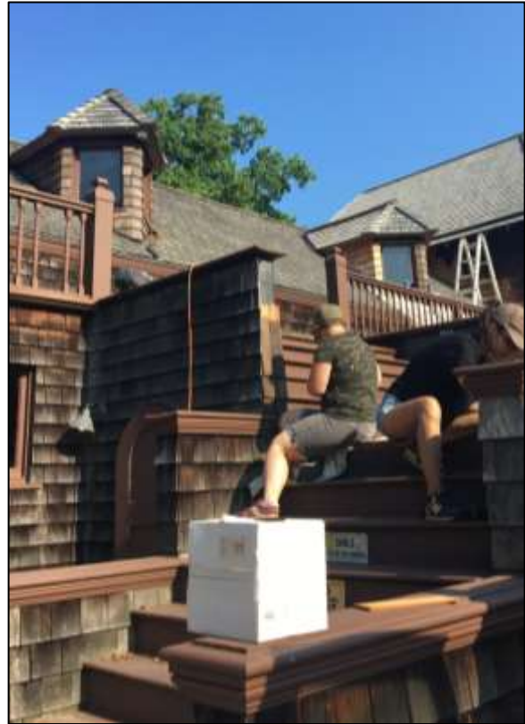
Installing shakes at Bowling and Recreation Pavilion, 2017
