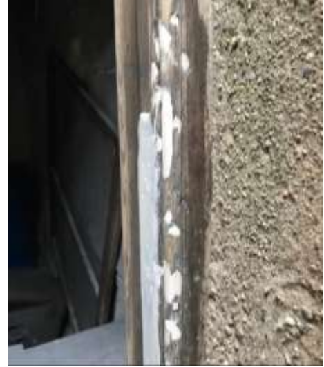
Epoxy fills in window frame at the Woodland's cryptoporticus, 2017
