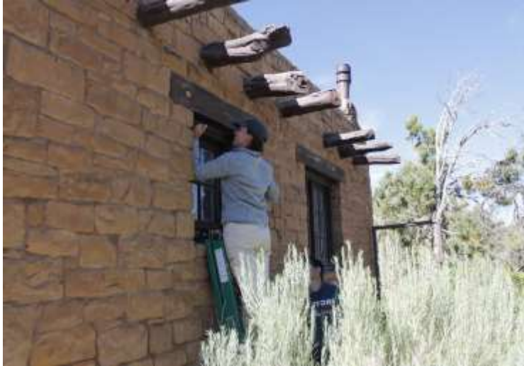
Taking wood samples for testing from an original window to the 1930 addition of Quarters 5 in Mesa Verde National Park, 2017
