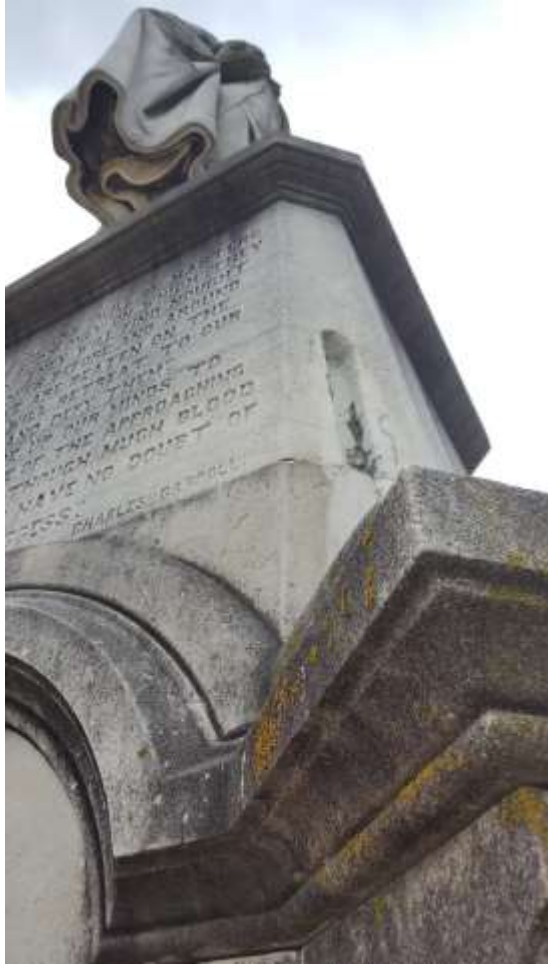
Removal of biogrowth and incorporation of cast replacement pieces at the Catholic Total Abstinence Fountain, 2017
