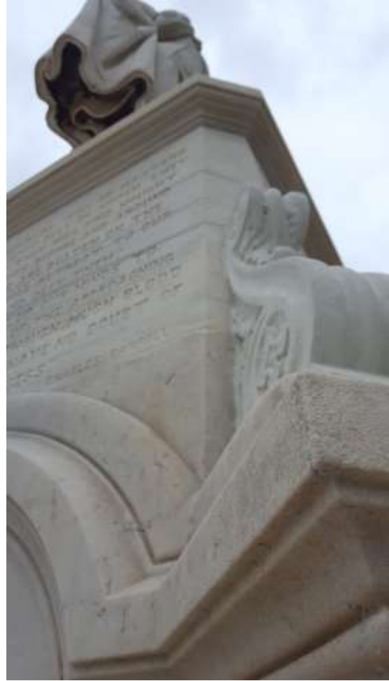
Removal of biogrowth and incorporation of cast replacement pieces at the Catholic Total Abstinence Fountain, 2017
