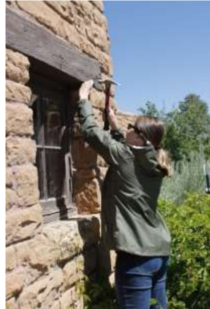
Taking paint samples from a lintel on Quarters 5 at Mesa Verde National Park, 2017
