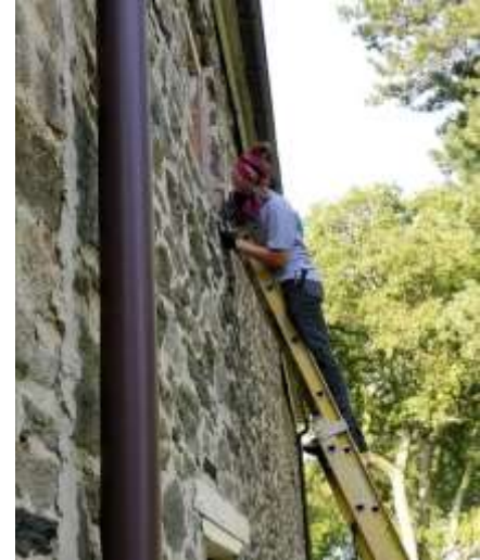
Stripping paint from a window of the Carriage House in Woodlands Cemetery, 2017
