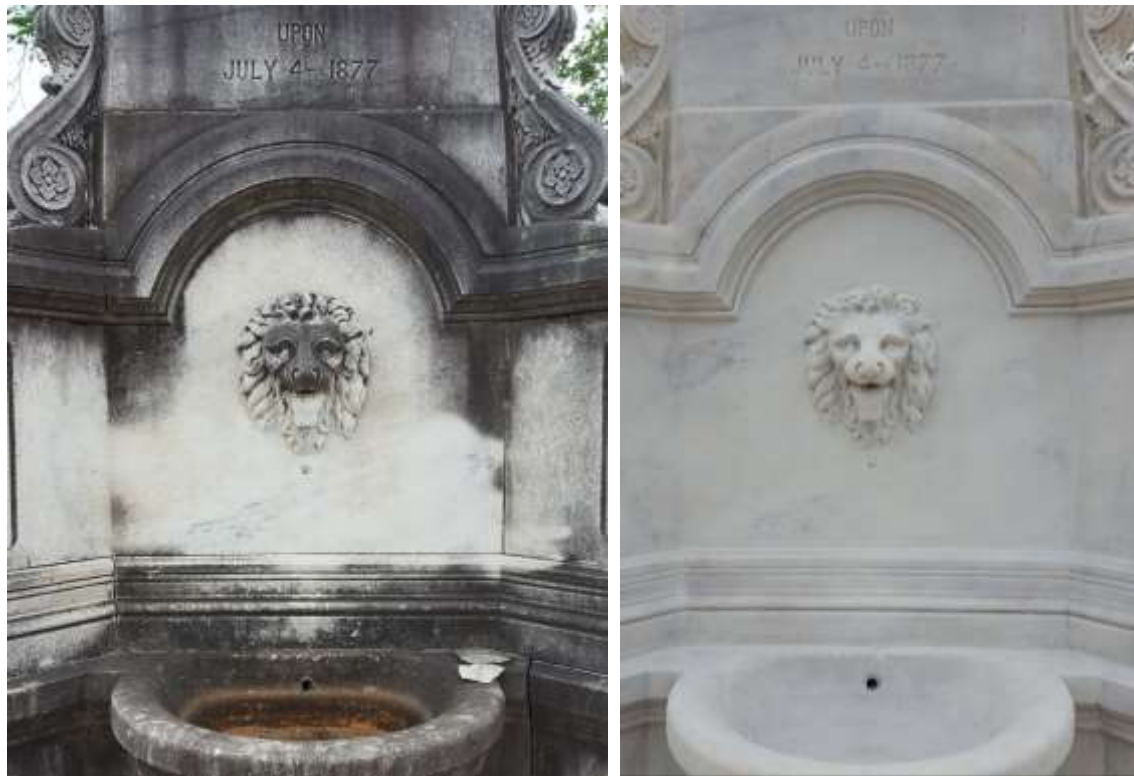
Removal of biogrowth at the Catholic Total Abstinence Fountain, 2017
