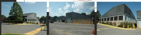
Planned demolition of the service complex required entry into the Virginia Cultural Resource Information System
