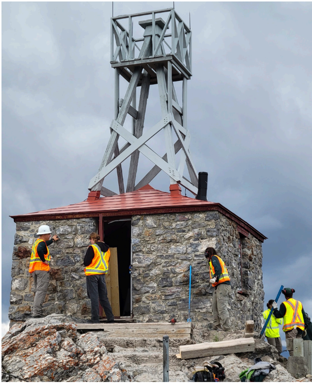
Image: Parks Canada workers conducting a condition assessment and window and deck removal on the observatory.
