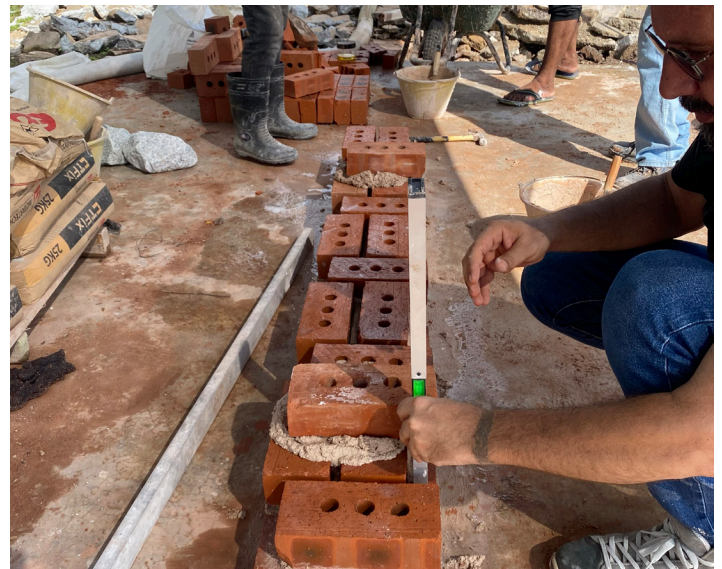
Image 2: Giovanni Santo demonstrating how to ensure all bricks are level in the mockup section wall
