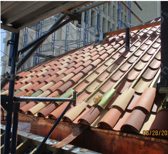
Image 1: Documentation of replacement clay tile installation progress at the west elevation of Casa Italiana.
