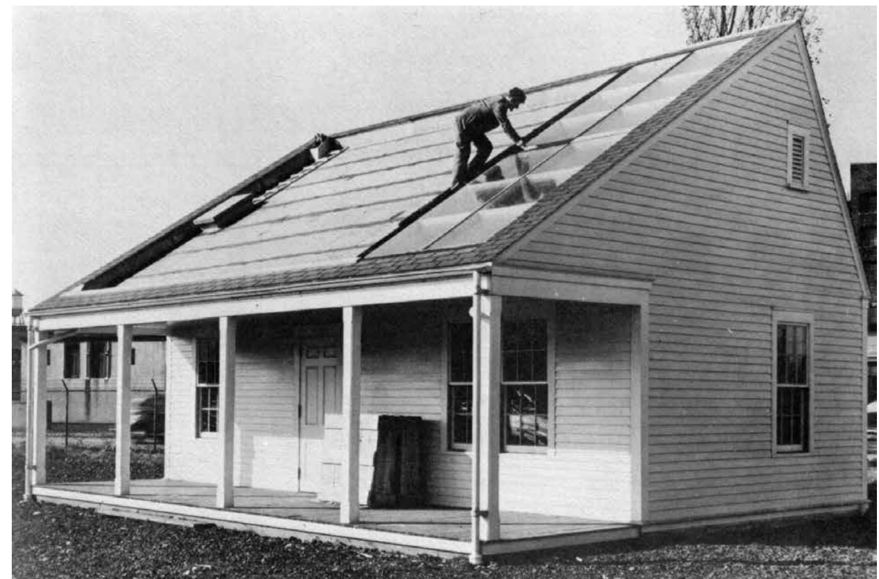
2. MIT Solar Energy Fund, Building 34, Cambridge, MA, 1939. Installation of solar panels. Hottel papers.
