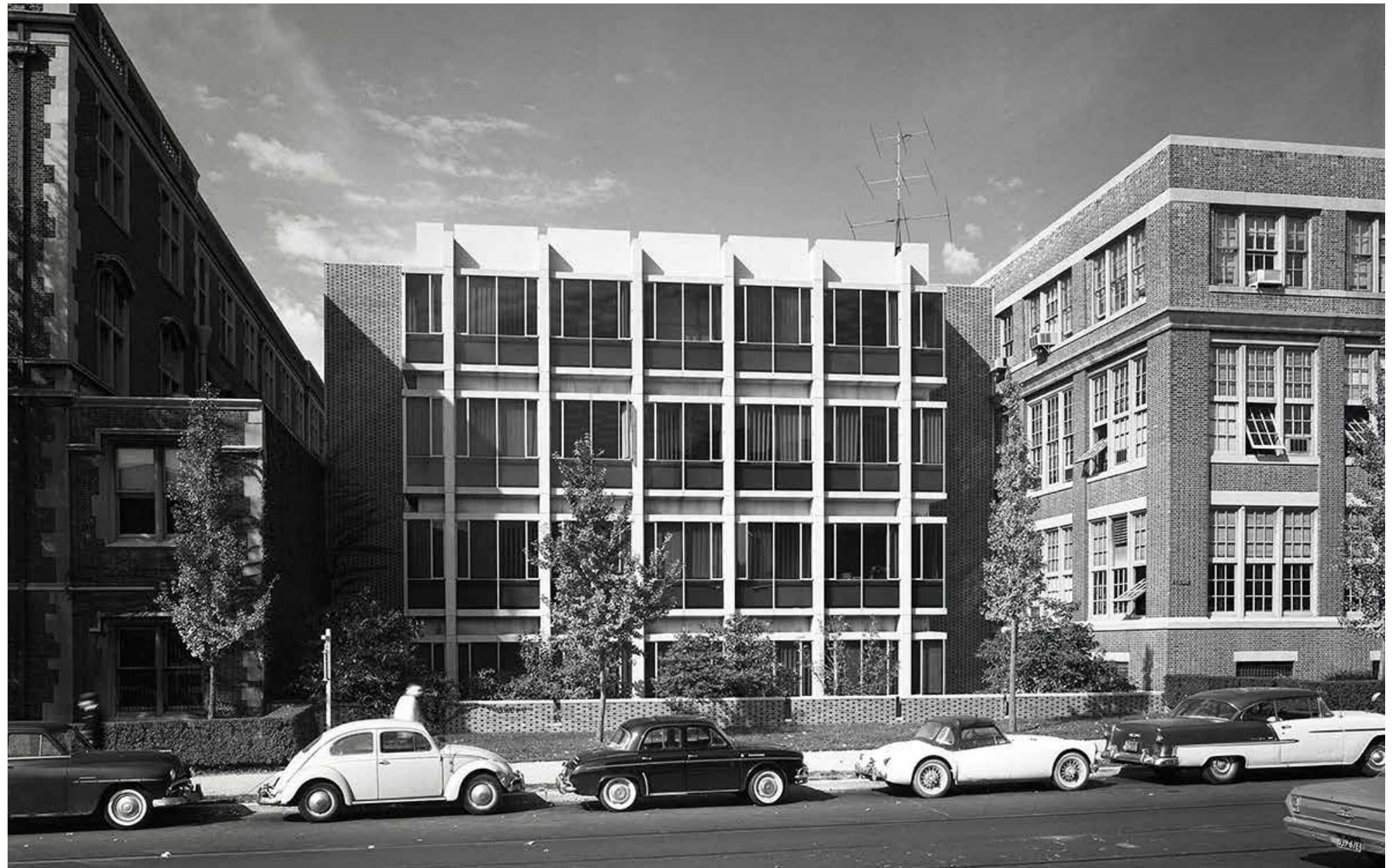
Figure 1. Pender Labs, Moore School of Engineering, University of Pennsylvania. (Source: Photo Credit: Athenaeum of Philadelphia, Lawrence Williams Inc. Collection, Local ID#:77133-A). Demolished.
