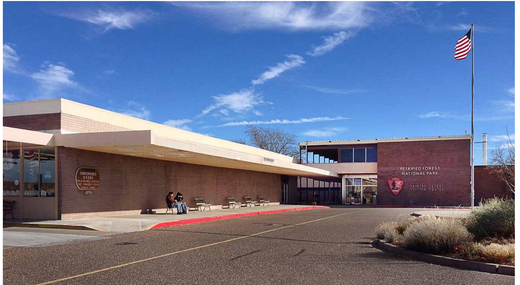
Figure 1. View of the Painted Desert Community Complex from the Main Visitor Parking Lot. (Source: Modern Phoenix LLC, "Neutra's Last Standing National Park Project Is Right Here in Arizona: Modern Phoenix." Neutra's Last Standing National Park Project is Right Here in Arizona | Modern Phoenix, 2013. Accessed May 3, 2022. https://modernphoenix.net/neutra/painteddesert.htm .)
