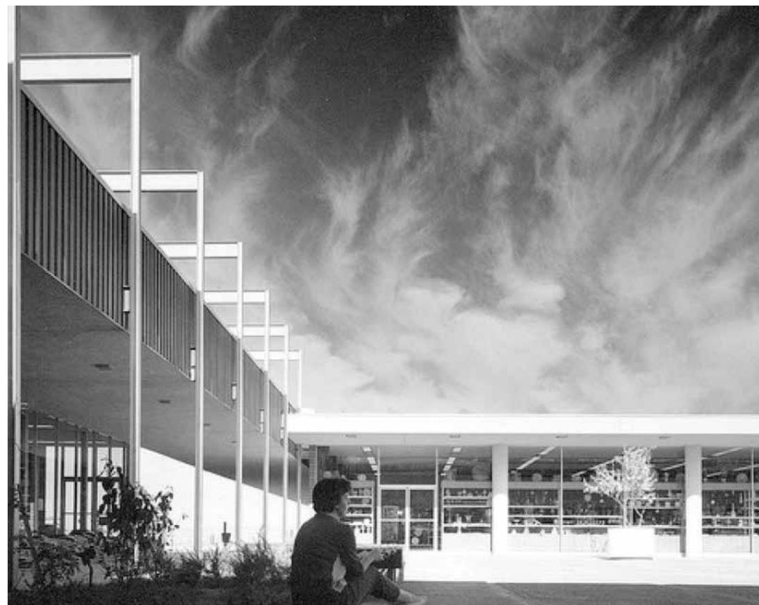
Figure 2. View of the Central Courtyard Facing West during the Construction of the Visitor Center. (Source: Beinlich Studios/ National Park Service, Photograph, 1960s, https://saving-places.org/stories/painted-desert-community-complex-returns-to-modernist-roots#.YnBVB-C1h1p8 , Accessed May 3, 2022).
