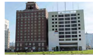
20 - Historic Hotel High rise hotels built in the late 19th and early 20th Century to accommodate for tourists.
