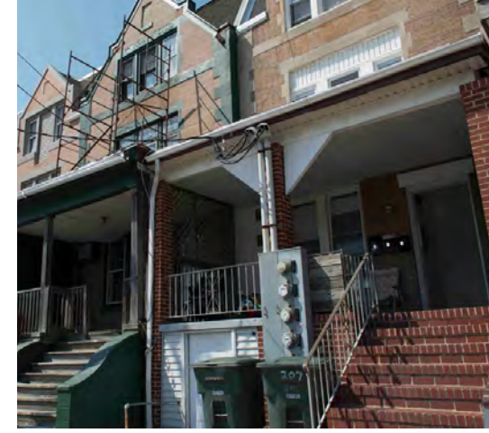
South Inlet // Intact Rowhomes
