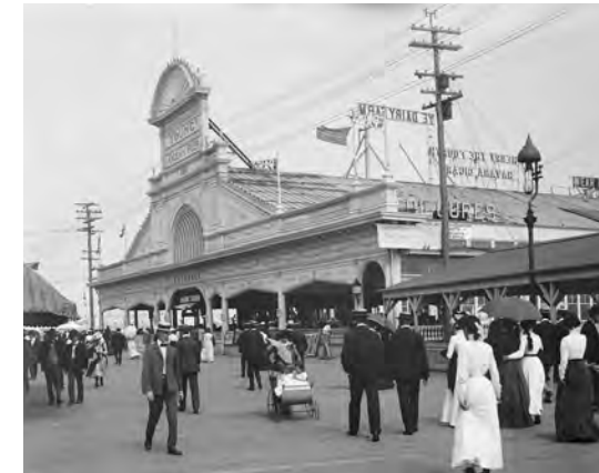
APPLGATE PIER (1884) // Tennessee Avenue
