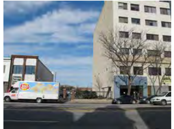
Vacant Lot on Atlantic Avenue near Kentucky, proposed site for new music venue
