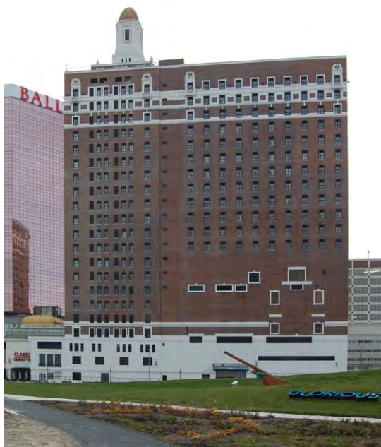
Blank facade left after demolition of the Sands
