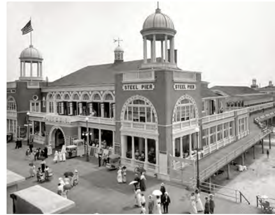
STEEL PIER (1898) // Virginia Avenue
