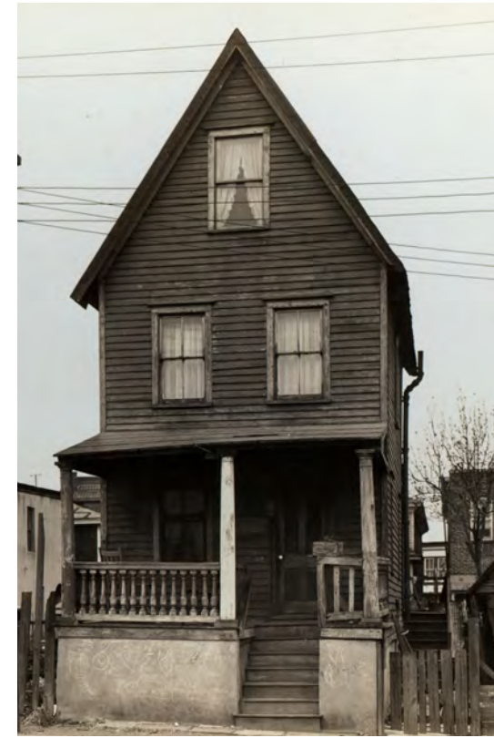
Photo #9 in Project NJ-14-1, December 15, 1939. // Courtesy of Bob Ruffolo, Princeton Antiques.
