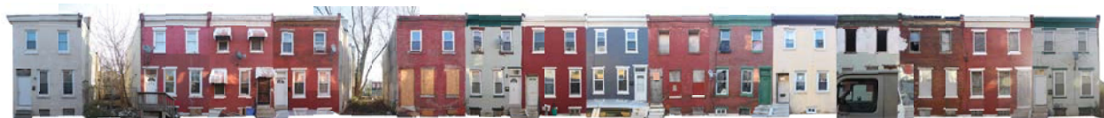
Figure 2. Elevation of east side of N. Brooklyn St.
