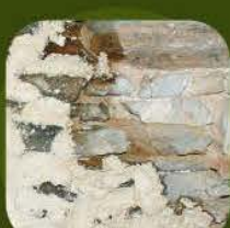
Lime and Mud Mortar
