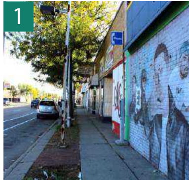
Figure 4.19. Sidewalk on the Strip
