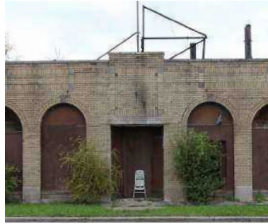
Figure 4.124. Arched, brick facade.
