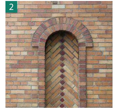
Figure 4.9. Blind Window + Brickwork
