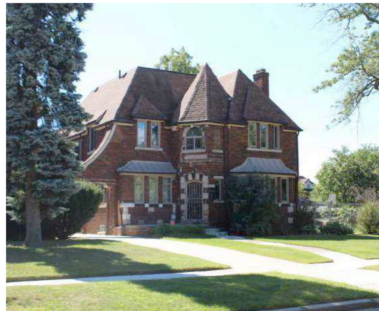
Figure 3.7. "Tudor Revival, Russell Woods". Example of the Tudor Revival Style in Russell Woods.
