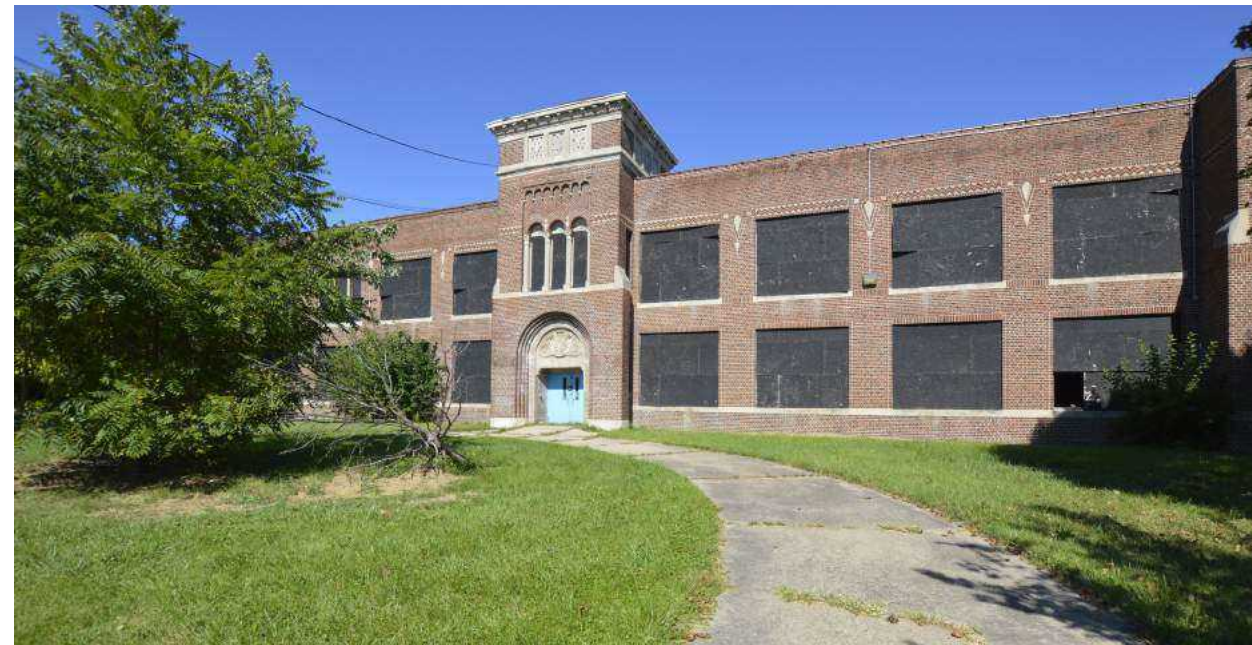
Figure 4.61. Elevation of McKerrrow School.
