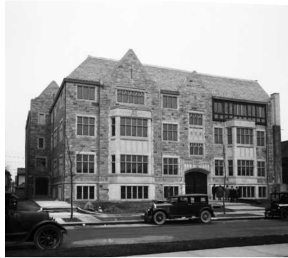
Figure 3.3. Nardin Park Methodist Episcopal Church, now Ebenezer AME Church), in November of 1928.
