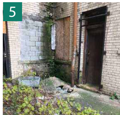
Figure 4.23. Water Damage Vestige
