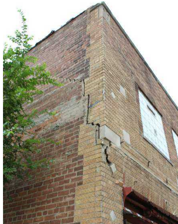
Figure 2.41. After damage that occurred during the 1967 rebellion and subsequent years of vacancy, it is not uncommon to find commercial properties with deteriorating storefronts.
