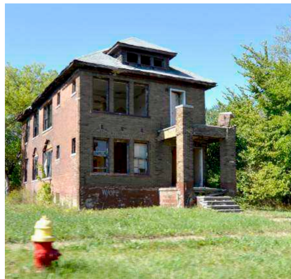
Figure 3.11. Two-story Nardin Park residence featuring a front porch and dormer, typical of multi-family housing in Nardin Park.
