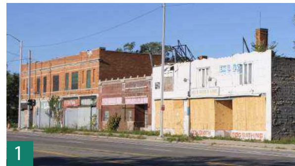
Figure 4.28. View of front looking north.
