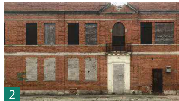
Figure 4.29. North side of 12546.
