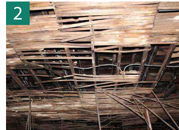
Figure 4.91. Roof of Vaughn's Bookstore building, 2018.
