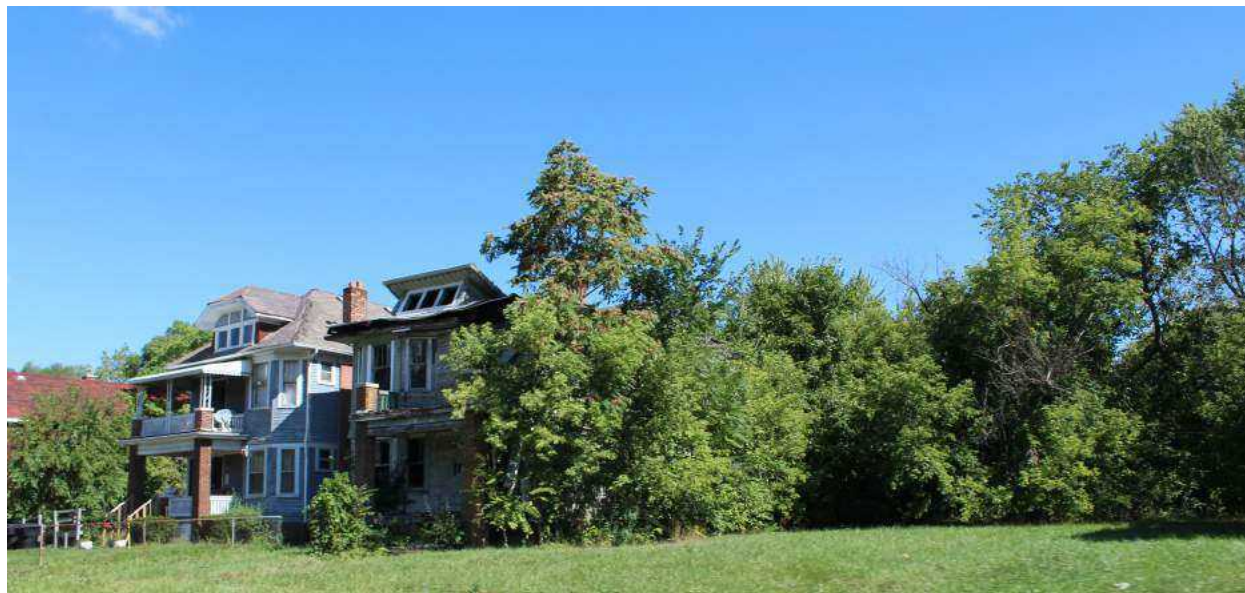
Figure 2.30. A typical street in Nardin Park, showing vacant land and buildings, more closely placed houses, several being multifamily, and significant overgrowth. Note the collapsed dormer and the surrounding empty lots, which are former house sites.
