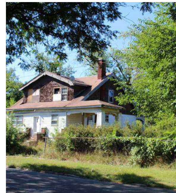
Figure 2.12: A vacant and derelict house in Nardin Park, with overgrowth around it.
