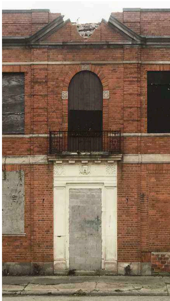
Figure 4.41. Side entrance of 12546 with decorative balcony and missing parapet detail along Fullerton Avenue.
