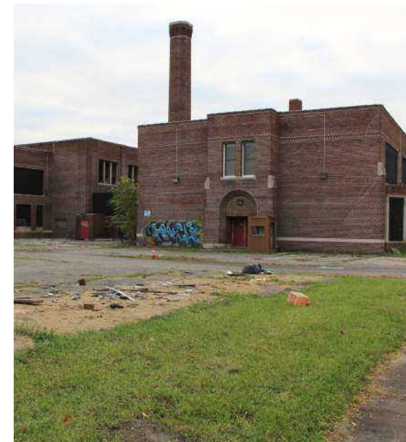
Figure 4.62. Rear of McKerrrow School.
