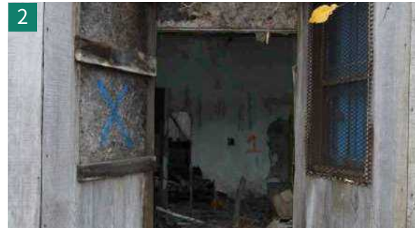
Figure 4.138. Exterior, Building B.
