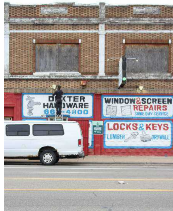
Figure 2.40. The Dexter Hardware Store is one of the few active businesses along Dexter Avenue. The building has recently undergone repairs and maintenance.
