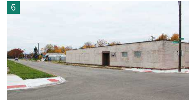
Figure 4.142. Exterior, Building G.
