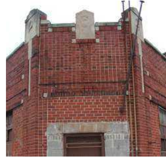
Figure 4.125. Chamfered corner and parapet detail.
