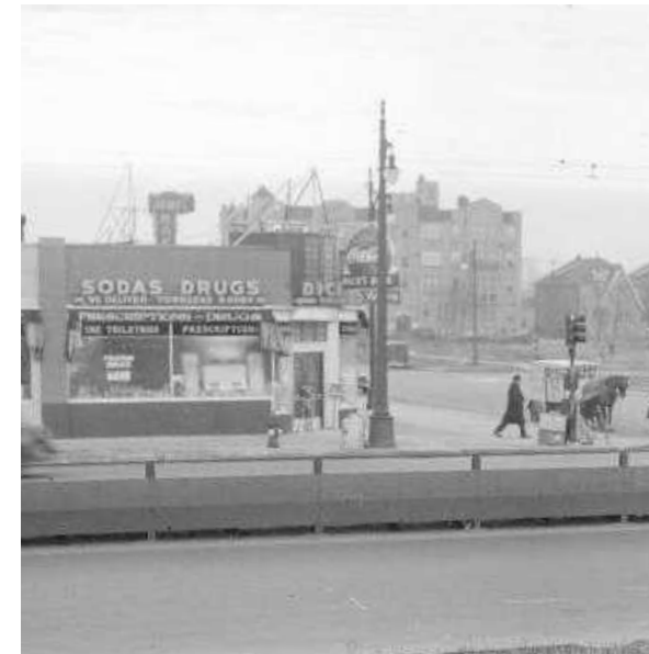
Figure 4.15. Circa 1940 image of the Tyler Apartments and no commercial strip, looking south from Davison and Dexter intersection.
