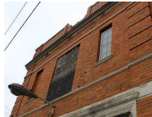
Figure 4.46. Parapet details and stone cornices on 12546.
