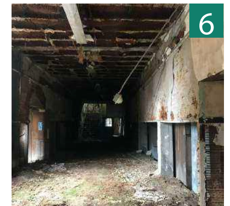
Figure 4.71. Hallway deterioration in McKerrrow School.
