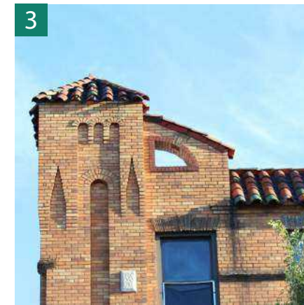
Figure 4.10. Parapet + Clay Tile Roof
