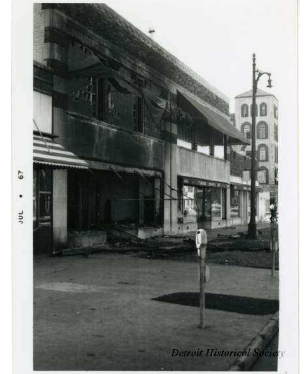
Figure 2.25. A 1967 image of a destroyed storefront along Dexter Avenue after the rebellion.
