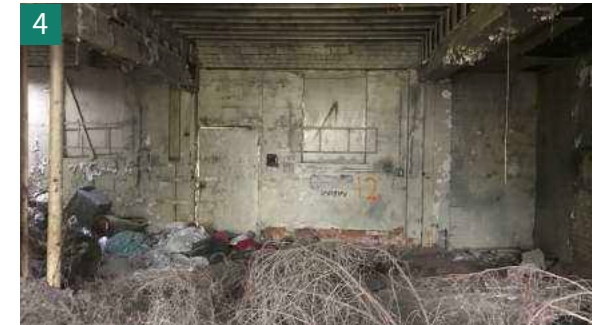
Figure 4.140. Interior, Building D.
