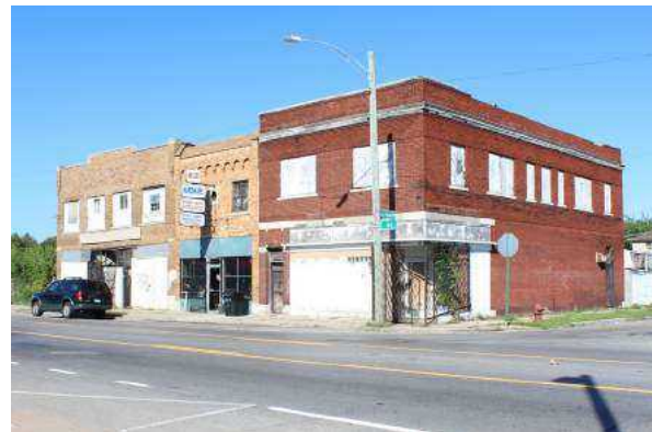
Figure 3.10. Small cluster of commercial properties along Joy Avenue
