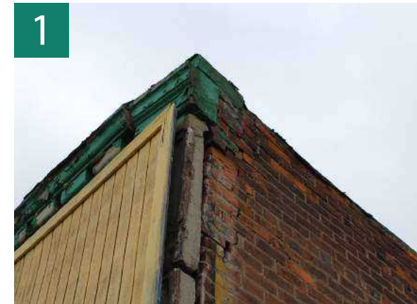
Figure 4.90. Cracking facade of Vaughn's Bookstore, 2018.
