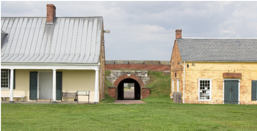
View northeast toward the Soldier's Barracks (left) and the Commissary (right) from the parade ground. Photo by A. Hita, 2017.
