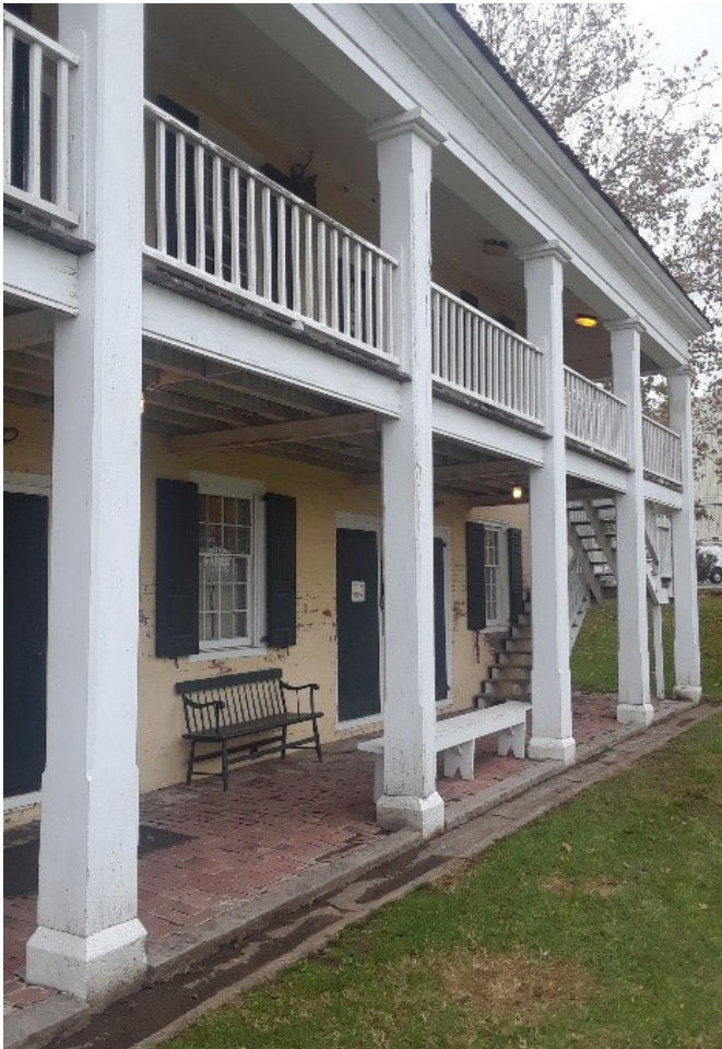
View northeast toward the colonnade of streamlined wood columns and covered porches on the Fort Mifflin Hospital building's facade. Photo by J. Giganti, 2017.
