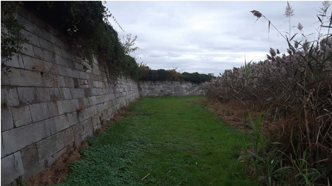
View northeast toward the exterior face of the fort's battered walls, which are primarily clad in ashlar gneiss here. Photo by J. Giganti, 2017.
