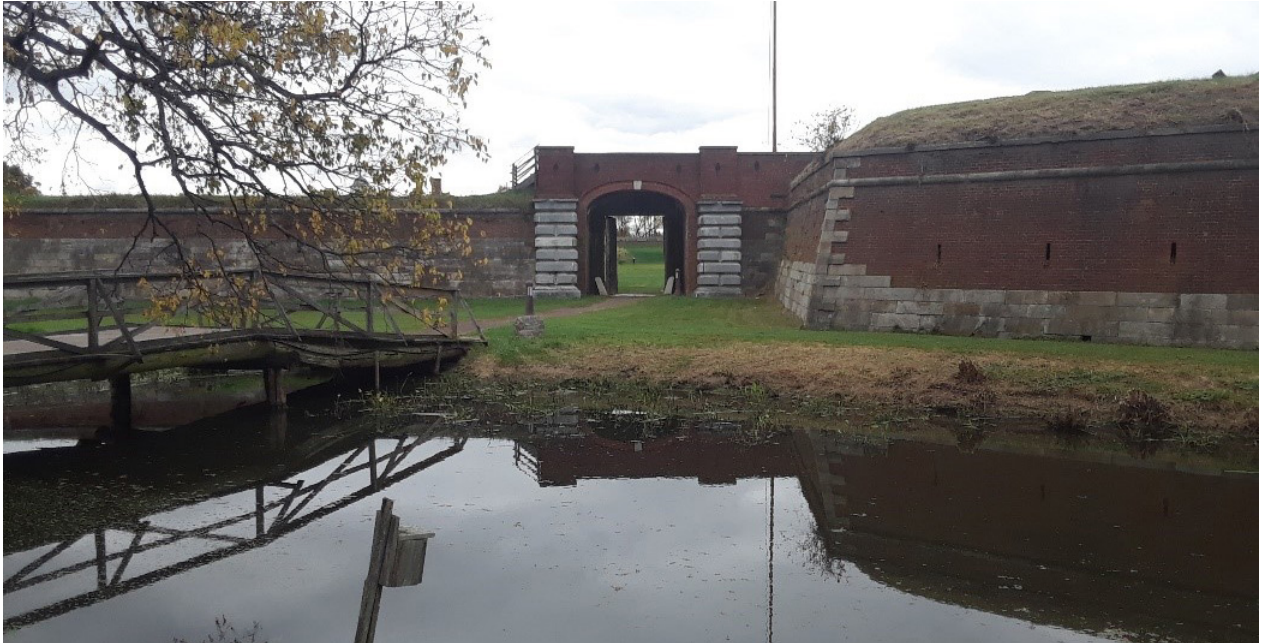
View across Fort Mifflin's moat, which is spanned by a footbridge, toward the East Sally Port. Photo by K. Britt, 2017.
