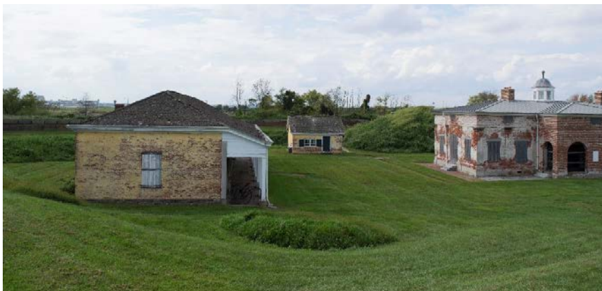
View northwest toward the Artillery Shed (left), Blacksmith Shop (center), Commandant's House (right) from the terreplein. Photo by J. Giganti, 2017.
