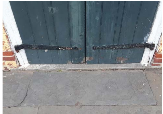
Below, wrought iron strap hinges on the Commissary's board-and-batten door, the doorway's gneiss sill, and slate tiles at the ground. Photos by K. Britt, 2017.
