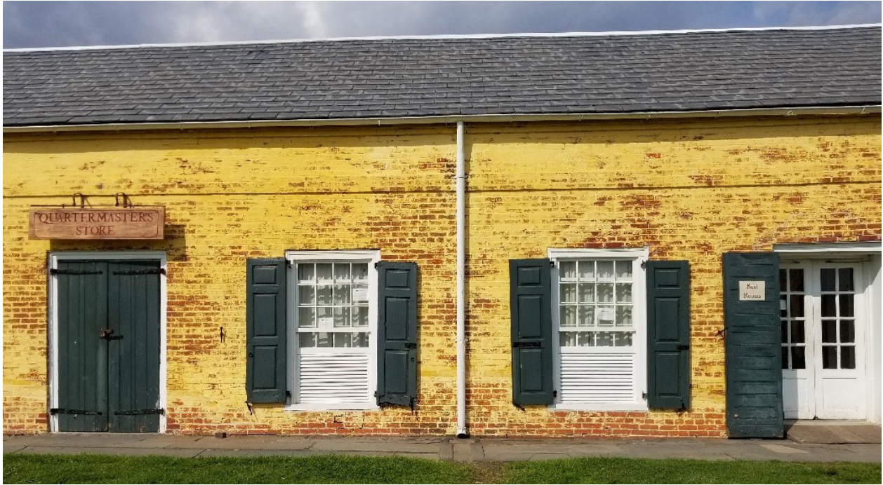
View northeast toward the Commissary. Note the common-bond brickwork, paneled, wooden shutters on the windows and doors, the small, multiple lights on both windows and doors, and the board-and-batten doors (left). Photo by J. Giganti, 2017.
