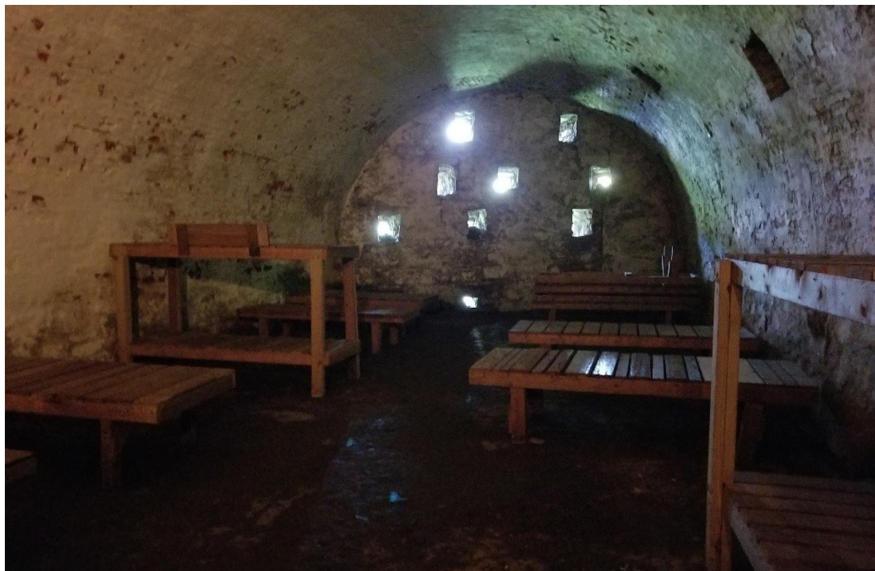
Interior of barrel-vaulted Casemate 5, located within the fort's walls. Note embrasures that provide natural light and ventilation. Photo by J. Giganti, 2017.
