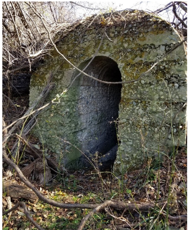
Entrance to a powder magazine on the never completed High Battery, which is located outside of the fort's walls on the southeast end of the property. Photo by S. Gdula, 2017.
