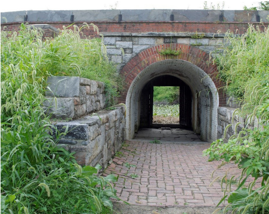
View northwest toward West Sally Port from inside of the fort. Photo by J. Giganti, 2017.
