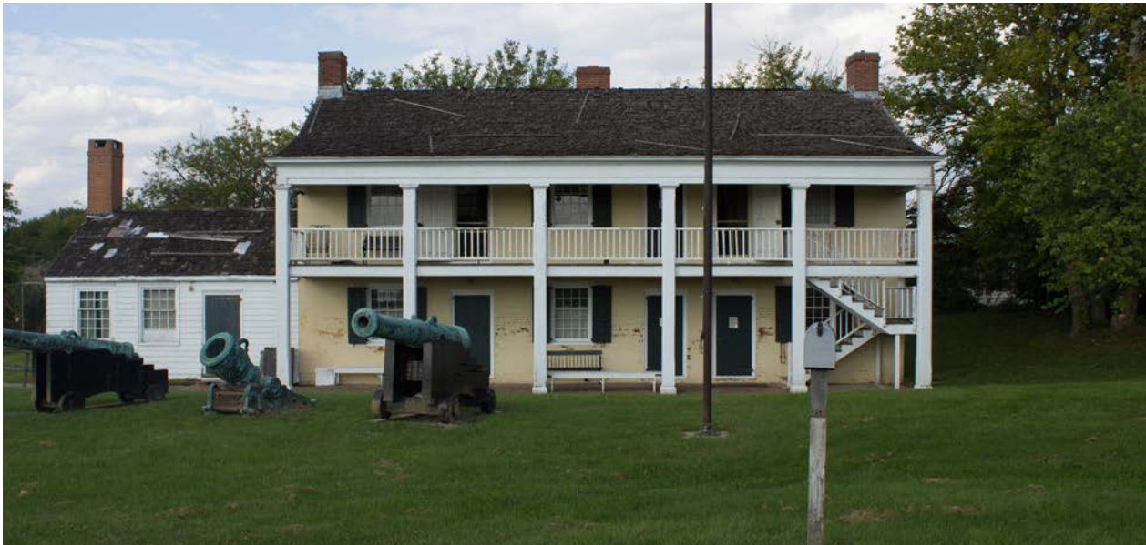
View northeast toward the Hospital Building's facade. Photo by A. Hita, 2017.
