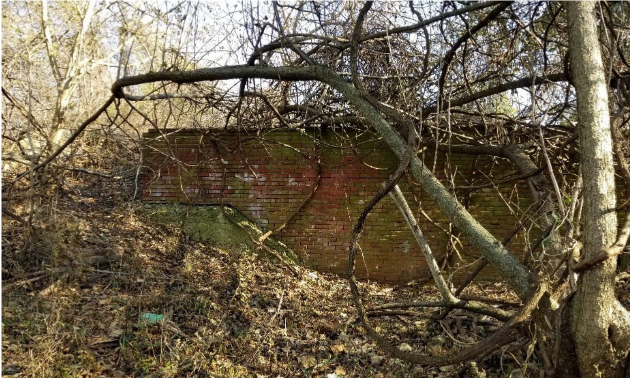
Remnants of a brick wall on the never completed High Battery, which is located outside of the fort's walls on the southeast end of the property. Photo by S. Gdula, 2017.
