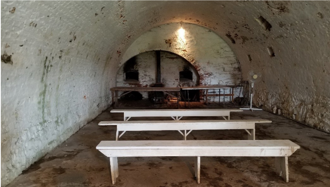
Interior of barrel-vaulted Casemate with built-in ovens and stoves on end wall. Photo by S. Gdula, 2017.
