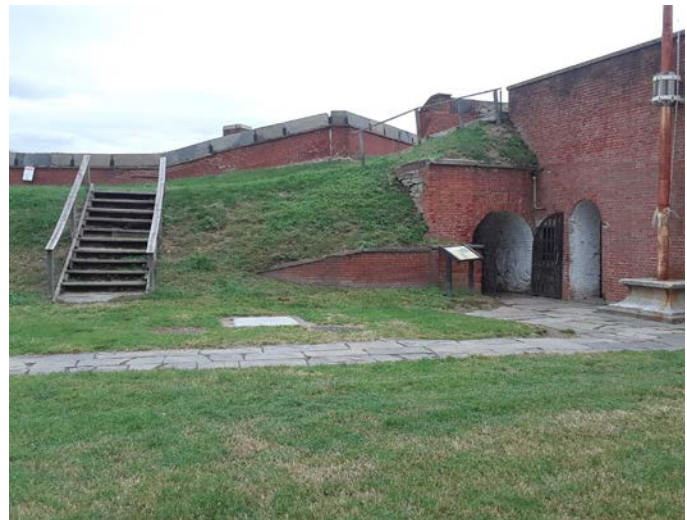
View east toward casemate entrances flanking the East Sally Port and stairs that provide access to the terreplein and the wall's parapet. Photo by J. Giganti, 2017.
