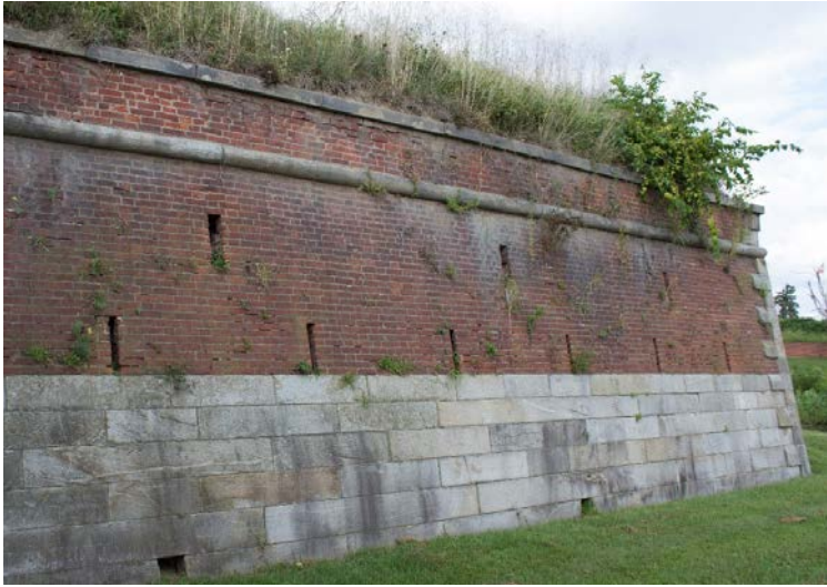
View northwest toward the exterior face of the fort's walls, east corner. Note battered form, Flemish-bond brick, ashlar gneiss base, quoins, and belt courses, embrasures, and overgrowth at parapet. Photo by A. Hita, 2017.
