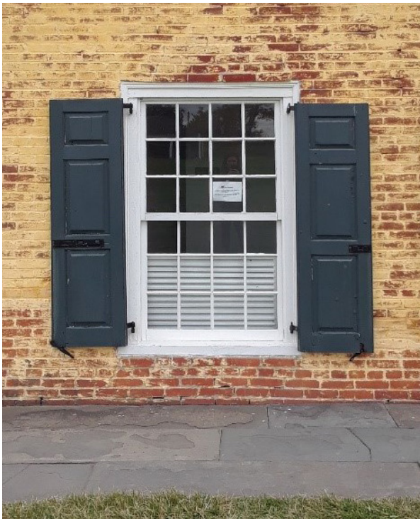
View northeast toward the Commissary. Note the common-bond brickwork, paneled, wooden shutters on the windows and doors, the small, multiple lights on both windows and doors, and the board-and-batten doors (left). Photo by J. Giganti, 2017.
