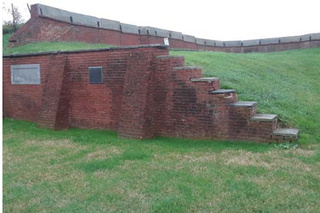
View south toward stepped brick wall with the buttresses and a portion of a terreplein flanking the East Sally Port. Photo by J. Giganti, 2017.
