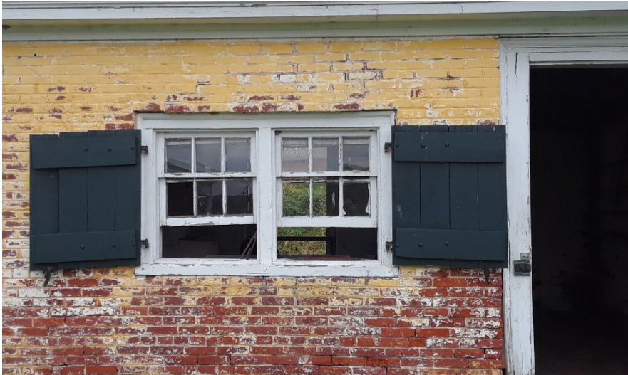
View northwest toward the Blacksmith Shop's paired wood-frame, double-hung, three-over-six light windows flanked by wooden shutters. Photo by J. Giganti, 2017.
