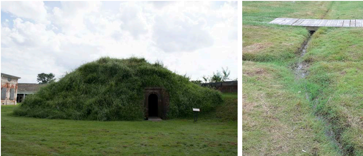
Left, a view southeast toward the earthen covered West Magazine located within the fort. Right, small channels for drainage within the fort. Photo by K. Britt, 2017.
