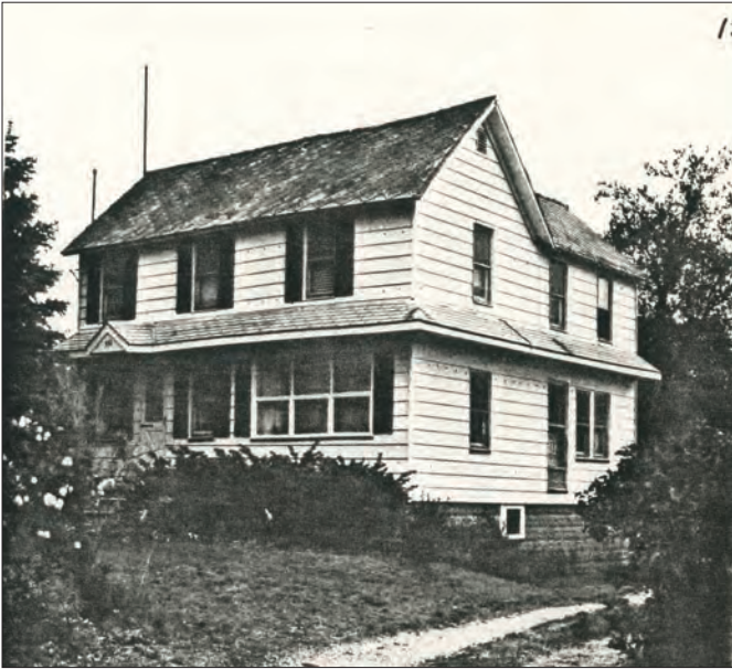
E-7: Alex Manluff House (Boynton, 1986)
