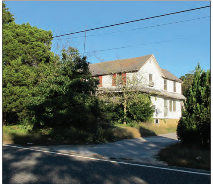
E-8: Alex Manluff House (Greenwich Studio Group)
