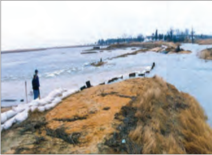
Image H-4: Pine Mount Levee Breach 1989 (South Jersey RC & D Council)
