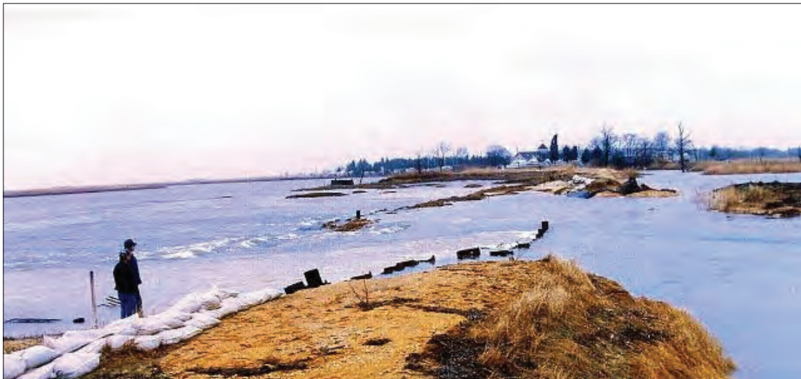
Pine Mount Levee Breach (South Jersey RC&D Council)
