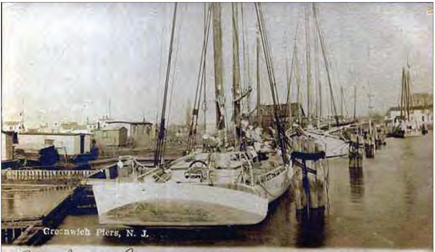
Greenwich Piers (Sustainable Greenwich)
