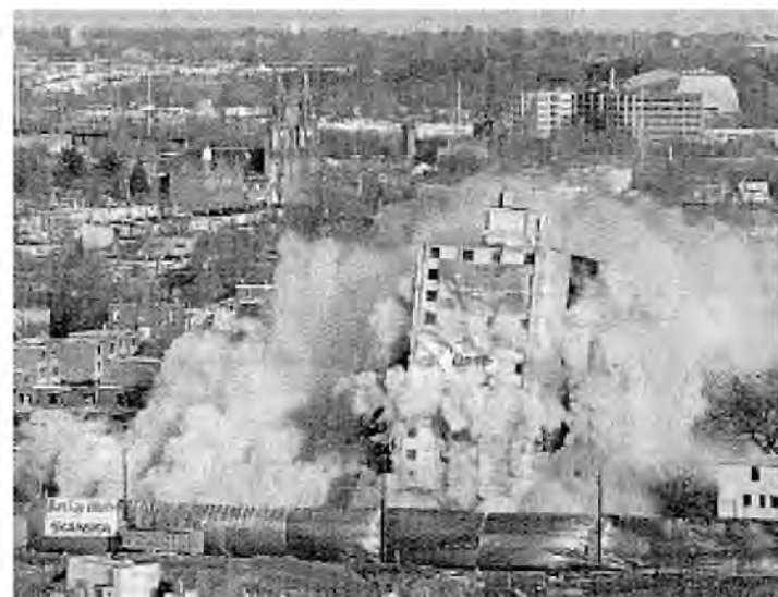
Implosion of Louis Kahn's Mill Creek Project Towers (Philadelphia: 2002.11.24).| Archinnet.com
