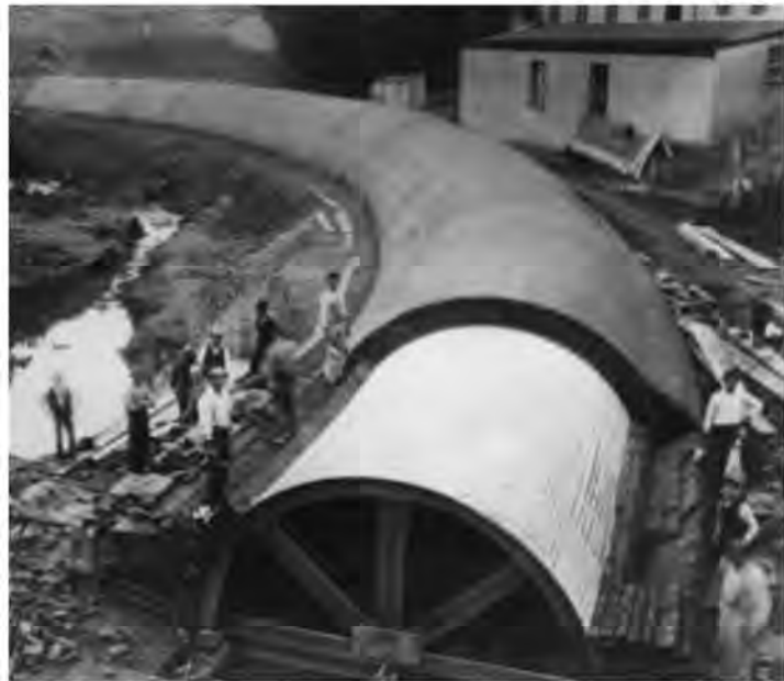
The Mill Creek Sewer is shown under construction at 47th Street and Haverford Avenue in 1883. Mill Creek once drained more than 4,500 acres of West Philadelphia | Courtesy of Philadelphia Water Department.
