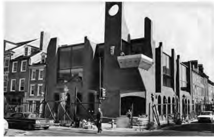
New Society Hill Construction | Special Collections Research Center, Temple University Libraries
