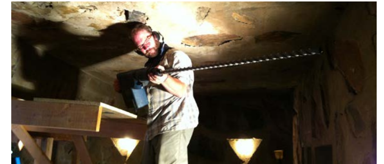
Figure 2.23 2012 structural roof repair Source: Frank Lloyd Wright Foundation Preservation Records
