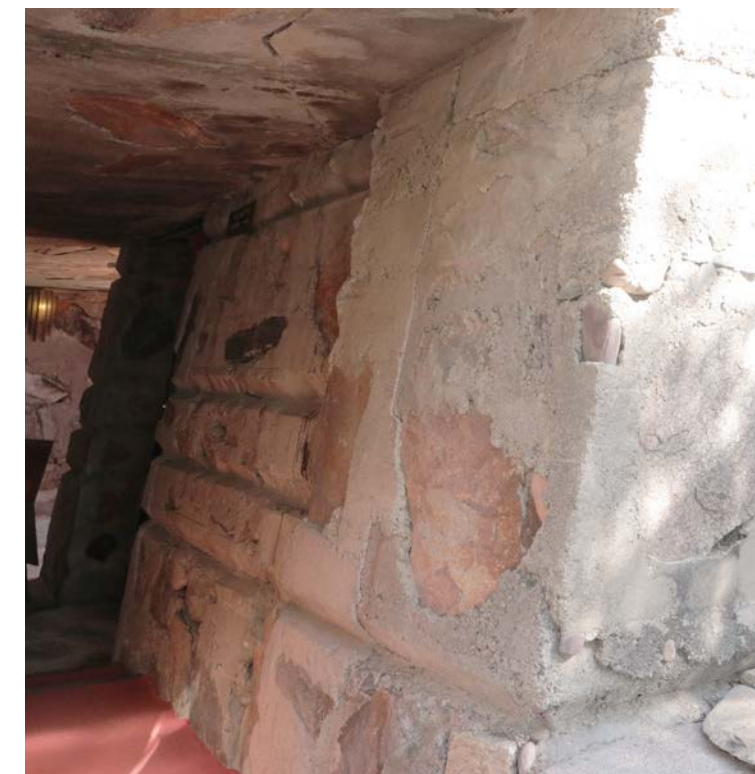
Figure 2.2 View looking South towards the exit, showing the masonry differences between Wright's office and the Cabaret addition. Image credit: Author, March 2023
