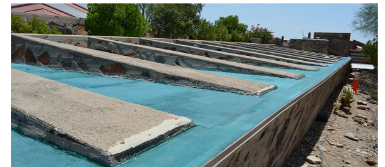
Figure 2.25 2015 roof system replacement Source: Frank Lloyd Wright Foundation Preservation Records
