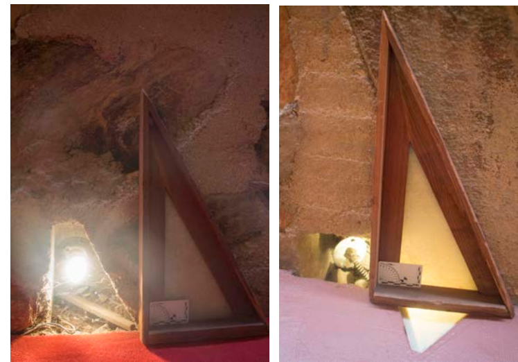
Figure 3.21 Left: Original base light Right: New triangular covers and original lights are blocked by the new ramp Image Credit: Author, March 2023
