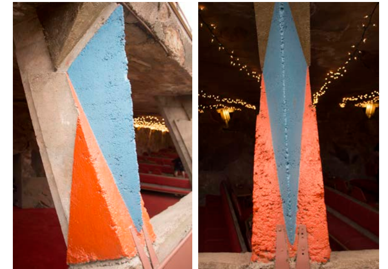
Figure 3.23 Decorative piers along the west side of the corridor Image Credit: Author, March 2023
