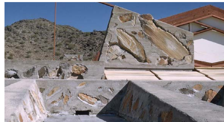
Figure 2.22 Historic photo showing the original drains in the parapet Source: Frank Lloyd Wright Foundation Archives
