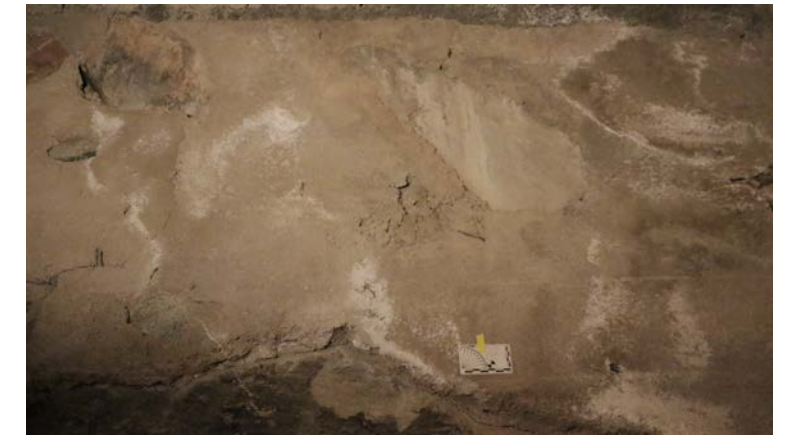
Figure 4.4 Salts found across the entire expanse of the West Wall in the Cabaret interior Image Credit: Authors, March 2023
