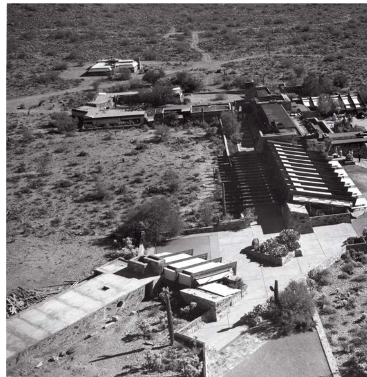
Figure 2.6 Close-up of historic aerial photo, showing the roof of the Cabaret before the beams were added. Source: Frank Lloyd Wright Foundation Archives
