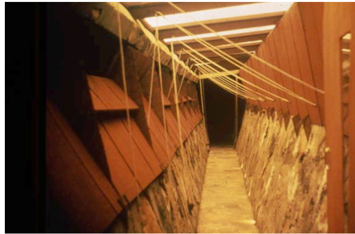
Figure 2.9 Corridor with the operable canvas panels in the Cabaret Source: Frank Lloyd Wright Foundation Archives
