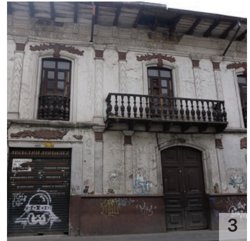
Vacant Building Due to Low Construction Capacity
