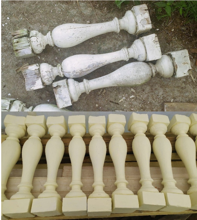
Glen Foerd Balusters, before and after repairs and repainting, 2018
