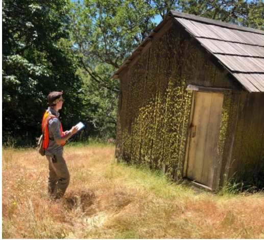
Assessing the condition of a historic shed in the Lyons Ranch Historic District, 2018.
