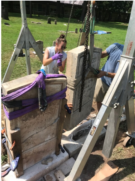
I operated the gantry and to guide headstones back into place for resetting. Pictured here is the dry run to ensure the headstone would sit levelly on its base after it was pinned. (2018)
