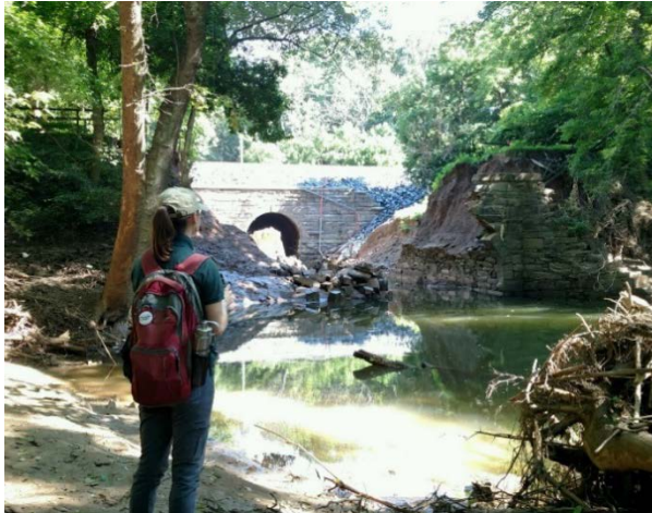
On a site visit to a flood-damaged culvert, 2018
