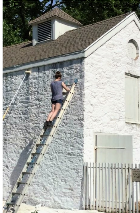
Applying lime wash to a structure at Woodford, 2018
