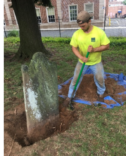
Removing soil to prepare headstone for treatment, 2018
