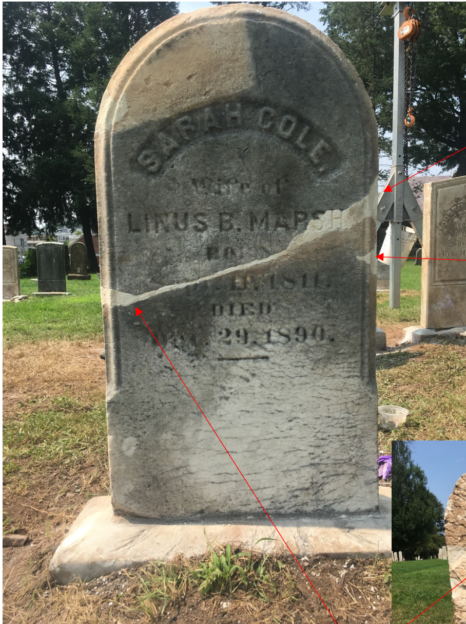
Front and back views of the same headstone and line of failure.
