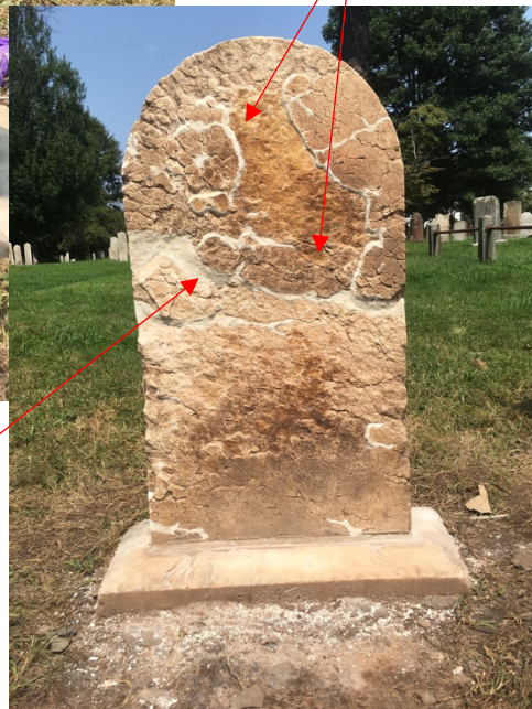
Front and back views of the same headstone and line of failure.
