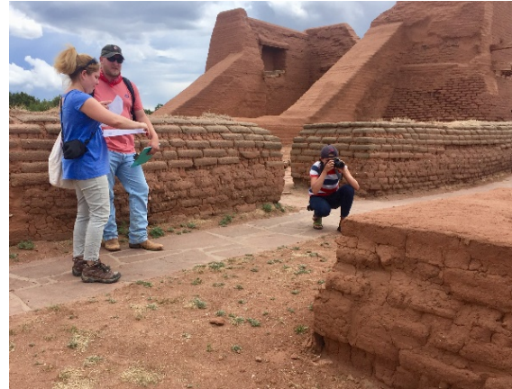
Testing a field survey and documenting various conditions of the convento walls at Pecos, 2018
