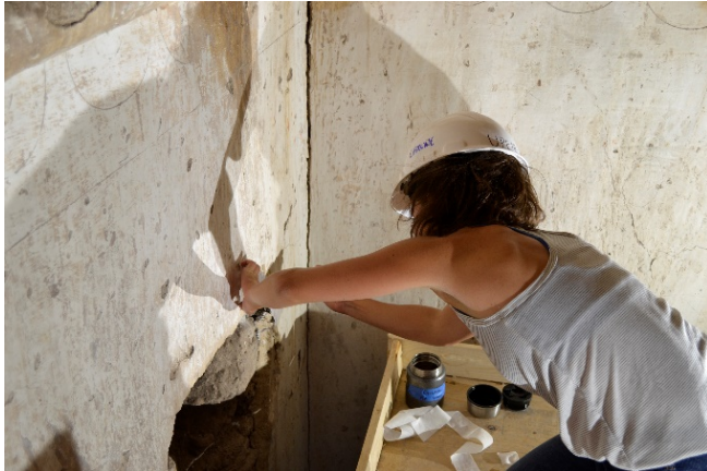
Applying gelatin-soaked bandages to damaged plaster at Mission San Jose de Tumacácori, 2018
