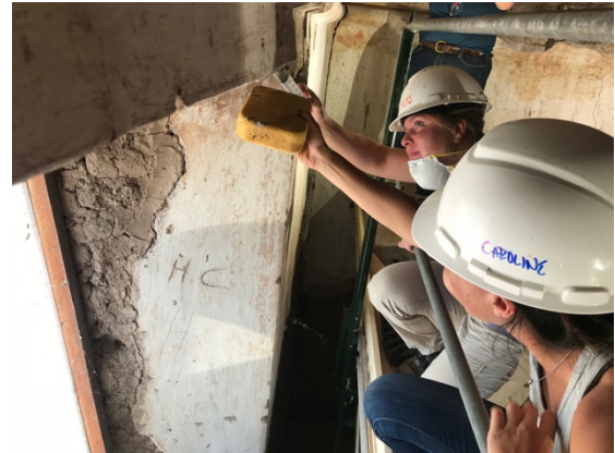
Me and the other intern injecting earthen grout as part of the plaster stabilization process in Tumacácori National Park, Arizona, 2018
