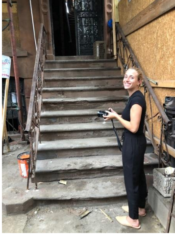
On a site visit to a fire damaged row house in the Bed-Stuy historic district, 2019
