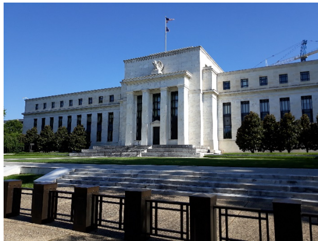
Mariner S. Eccles Building, Federal Reserve System built in 1937, 2019
