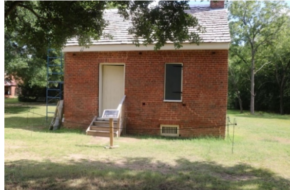
Dairy front elevation following restoration work, 2019
