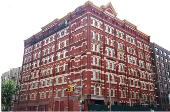
The Windermere, an individual landmark saved from demolition by neglect has been undergoing restoration since 2009, 2019
