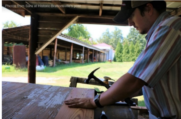
Clenching nails on a replacement board for the door, 2019
