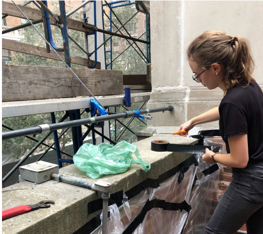
Prep work for water testing, 2019
