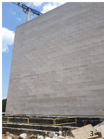
Preservation issues within the Smithsonian Air and Space Museum (built-in 1976) including the whole stone panel replacement from the facades, 2019
