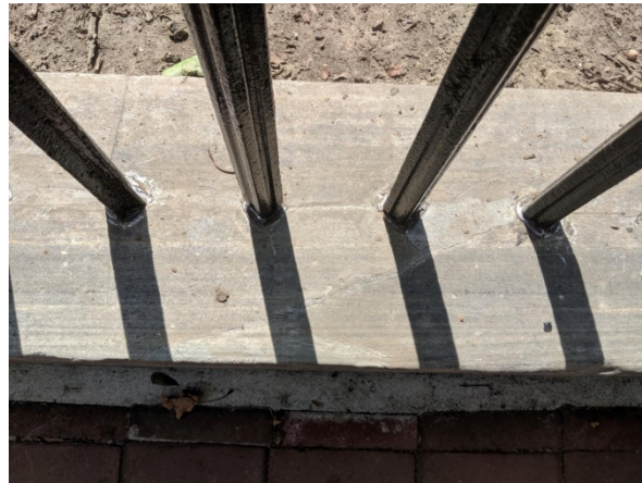
Some composite fills in the cracks of a large stone that had been cleaved in half by a nearby tree root, 2019
