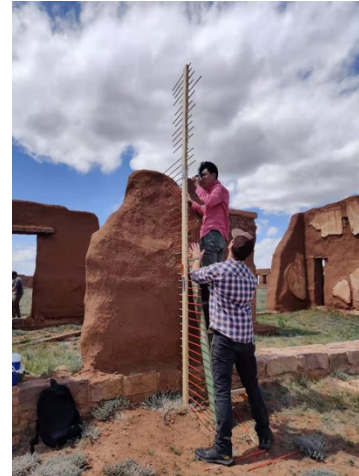
Recording the remains of an adobe wall with a profile gauge at Fort Union, 2019
