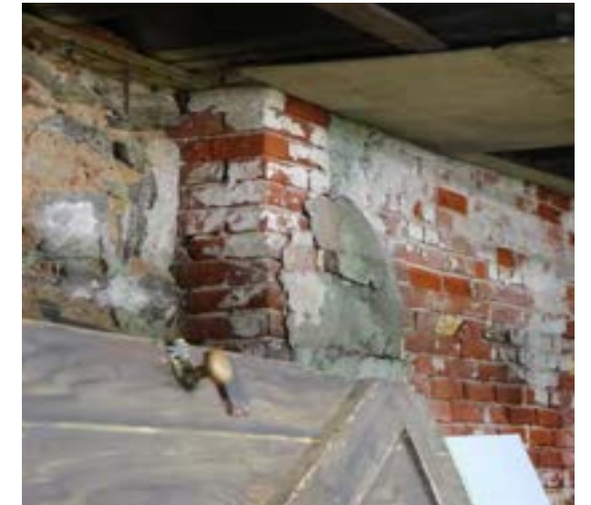
Figure 8: Stone and masonry walls with detached plaster, 2024 (DCT Studio Group)
