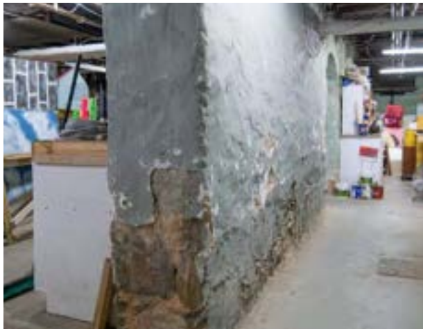
Figure 17: Raising damp impacting 1892-SE-WALL-INT (November 29, 2024)
