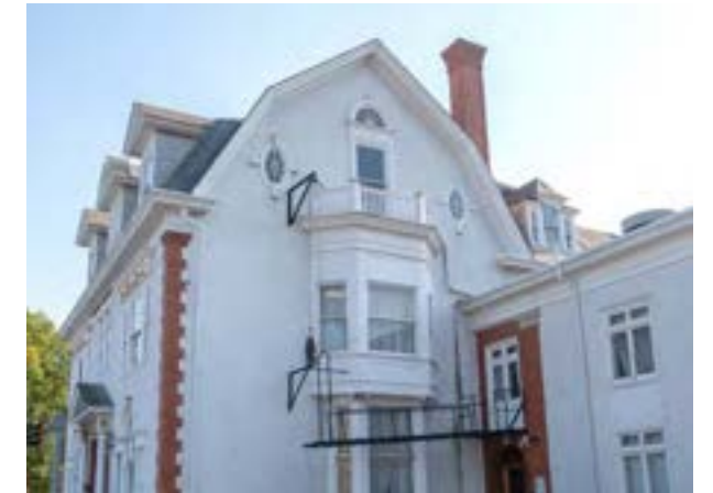
Figure 3: Northwest elevation. Note bay windows, fan light, and oval lights.
