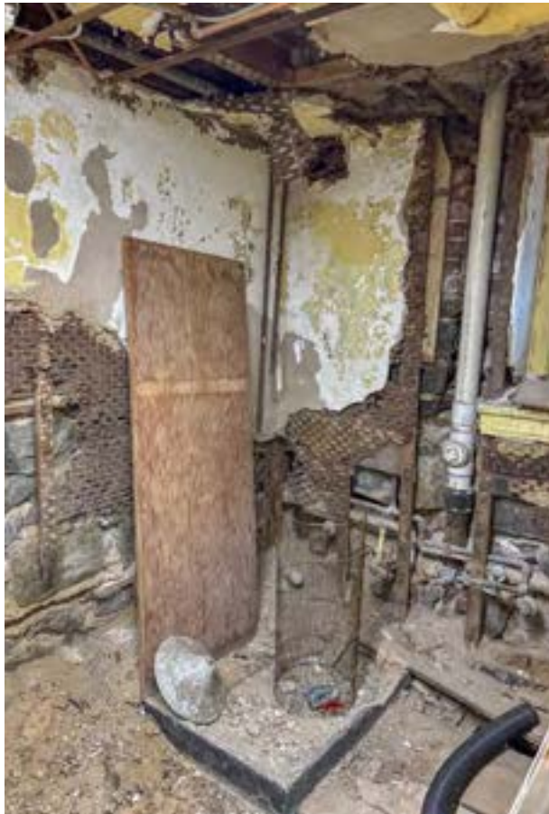
Figure 9: Old machinery room adjacent to exposed perimetral wall and exposed metal mesh. Note the accumulation of material, 2024 (DCT Studio Group)
