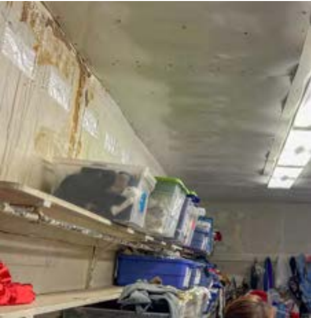
Figure 2: Staining observed on 3 rd floor wall and ceiling, September 5, 2024
