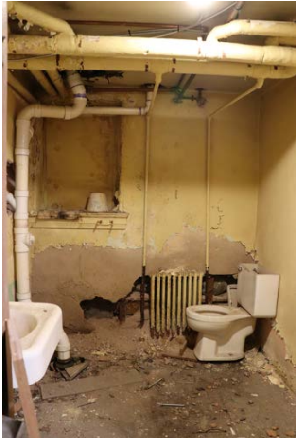
Figure 10: Closed restroom with water infiltration due to rising damp and possible water leakage, 2024 (DCT Studio Group)
