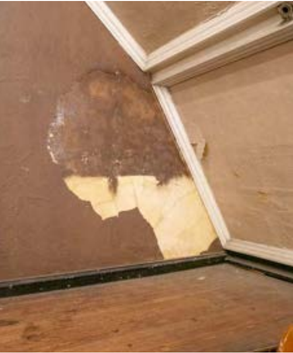
Figure 17: Detachment at auditorium balcony, 2024 (DCT Studio Group)
