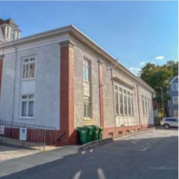
Figure 12: Exterior view of 1922-NW-WALL with concrete and window closures (November 29, 2024)
