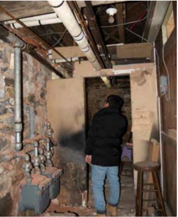
Figure 18: Brick powdering on 1892-NE-WALL (November 29, 2024)
