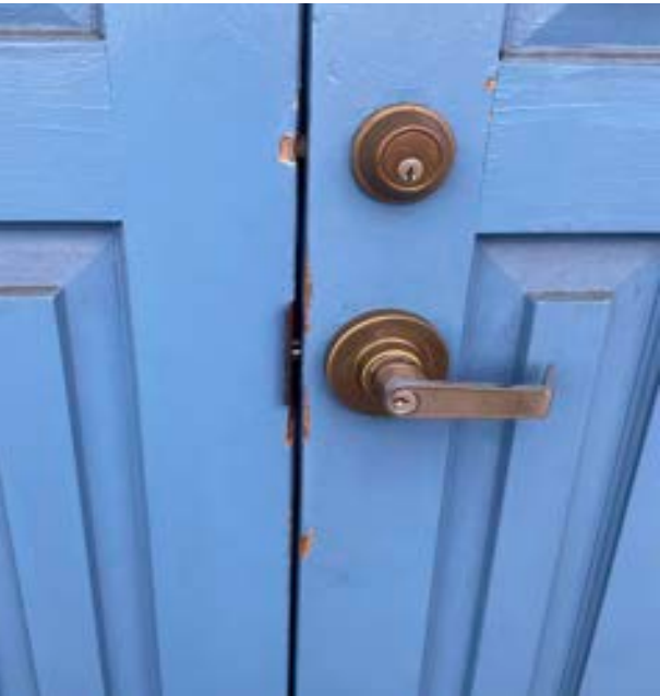
Paint Peeling of Door of D. NFAC.01.1
