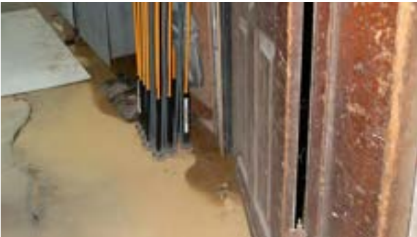
Figure 6: Water pooling around 1892-SE-WALL (November 29, 2024)
