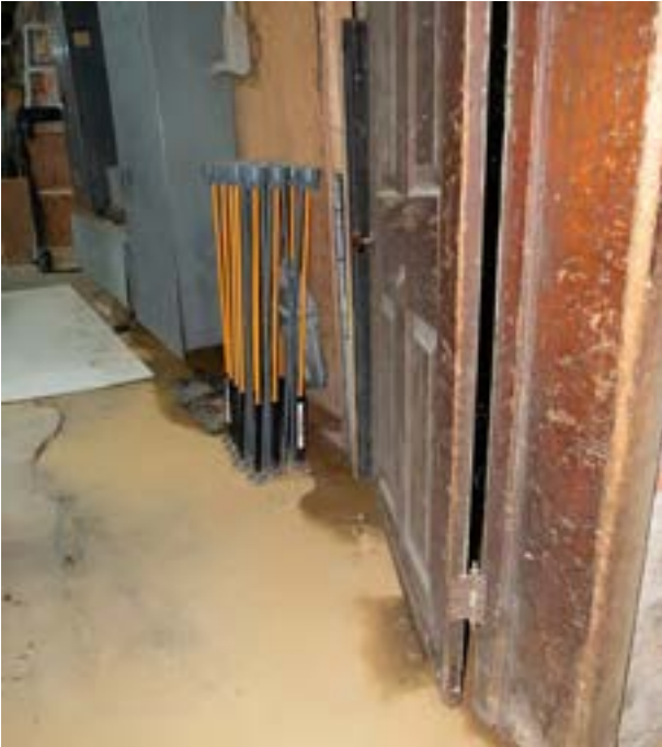
Figure 1: Moisture observed along southeast basement wall beneath electrical units, November 29, 2024
