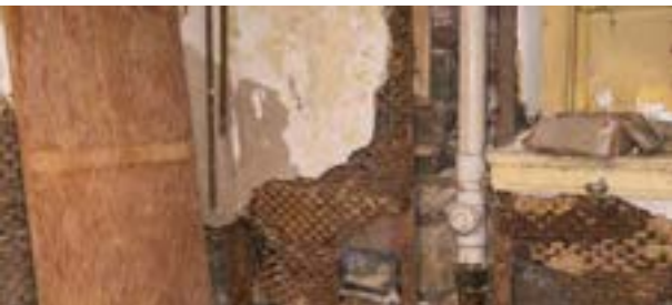
Figure 10: Plaster peeling from furring on 1922-NE-WALL (November 29, 2024)
