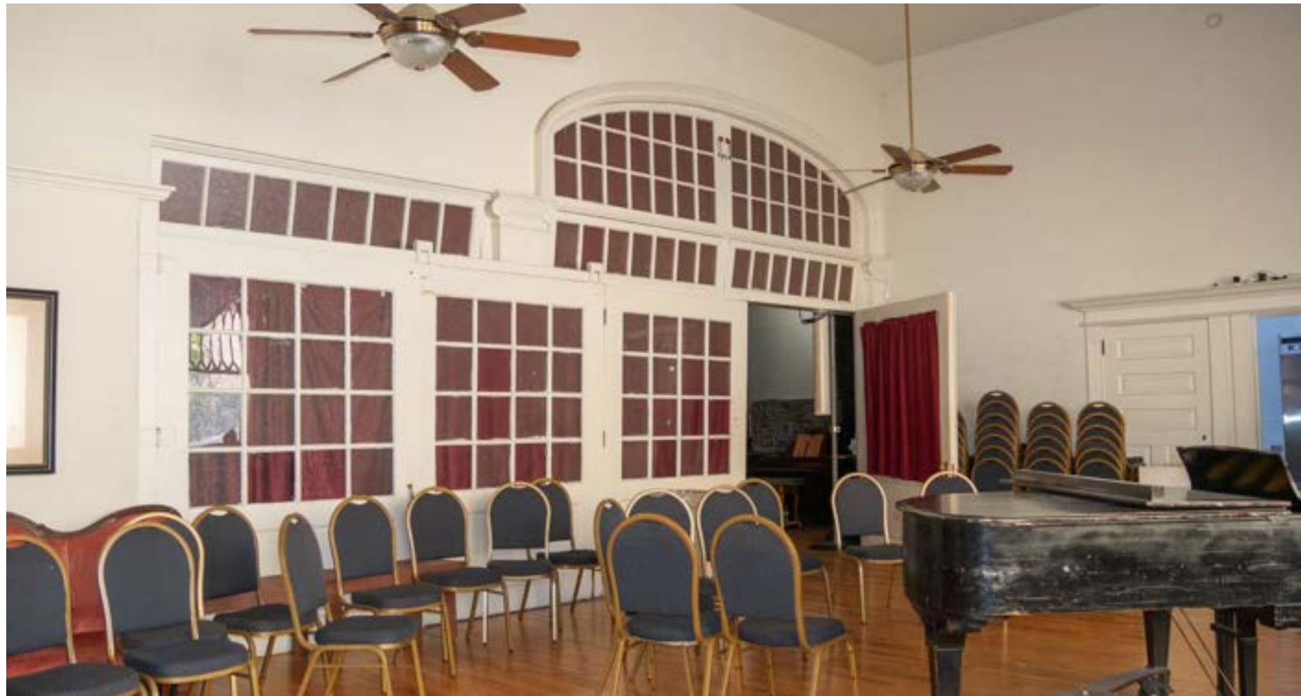
Figure 4: View of southeast elevation, featuring 1922-designed slidable and swingable windows and doors. Note operable transom windows, 2024 (DCT Studio Group)
