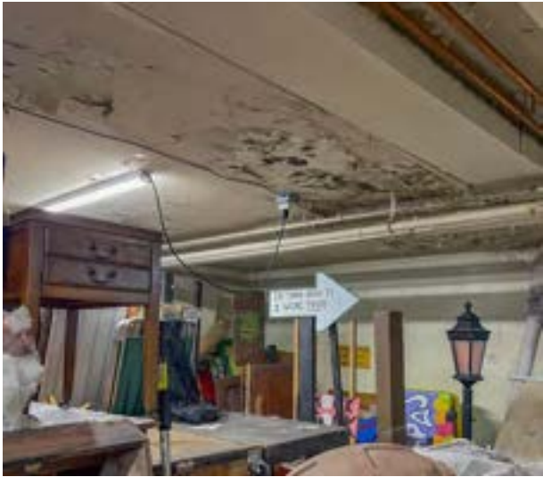
Figure 13 (Left): Plaster detachment on ceiling, 2024 (DCT Studio Group)
