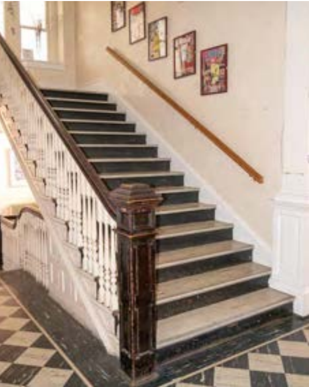
Figure 21: Deteriorated wooden balustrade on stairway, 2024 (DCT Studio Group)
