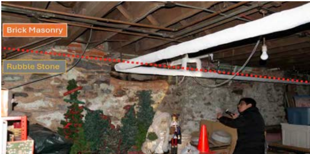
Figure 4: Rubble stone masonry supporting the brick masonry walls and first floor joists on 1892-NW-Wall (November 29, 2024)
