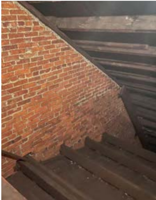
Figure 5: Connection of brick wall, historic roof and auditorium ceiling at the attic, 2024 (DCT Studio Group)
