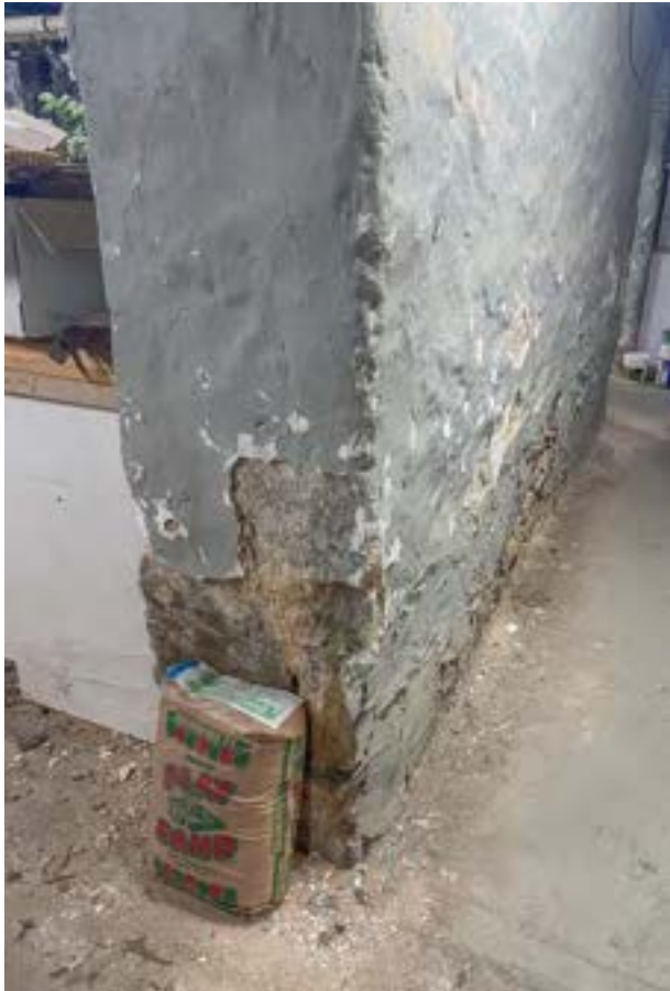
Figure 12: Moisture on wall along hallway due to rising damp, 2024 (DCT Studio Group)
