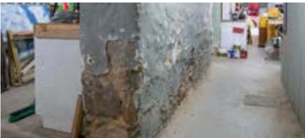
Figure 8: Plaster peeling on stone wall on 1892-SE-WALL-INT. (November 29, 2024)
