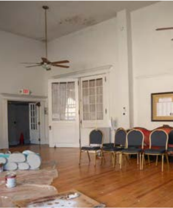
Figure 16: Buffet Room, note moisture on ceiling corner, 2024 (DCT Studio Group)
