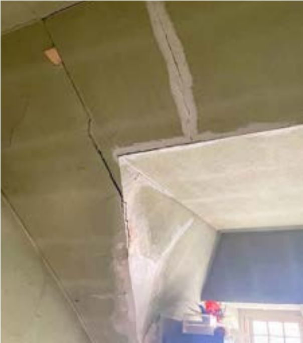
Figure 18: Cracks along patches and repairs, 2024 (DCT Studio Group)
