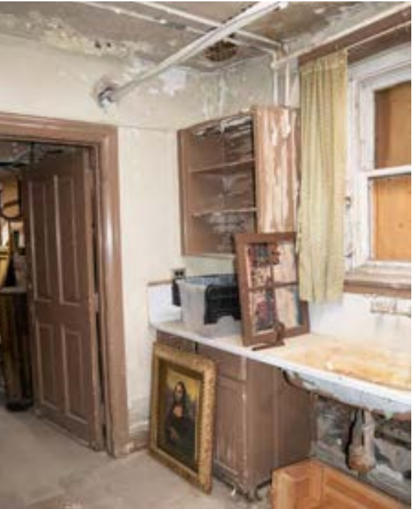
Figure 21. Plaster detachment from ceiling and furring on 1922-NW-WALL (November 29, 2024)
