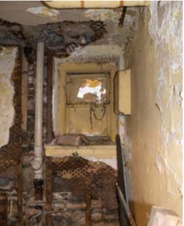
Figure 20. Plaster detachment from furring on 1922-NE-WALL (November 29, 2024)
