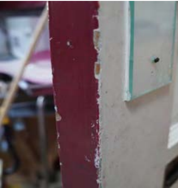
Paint Peeling of Door of D. BUFF.01.23
