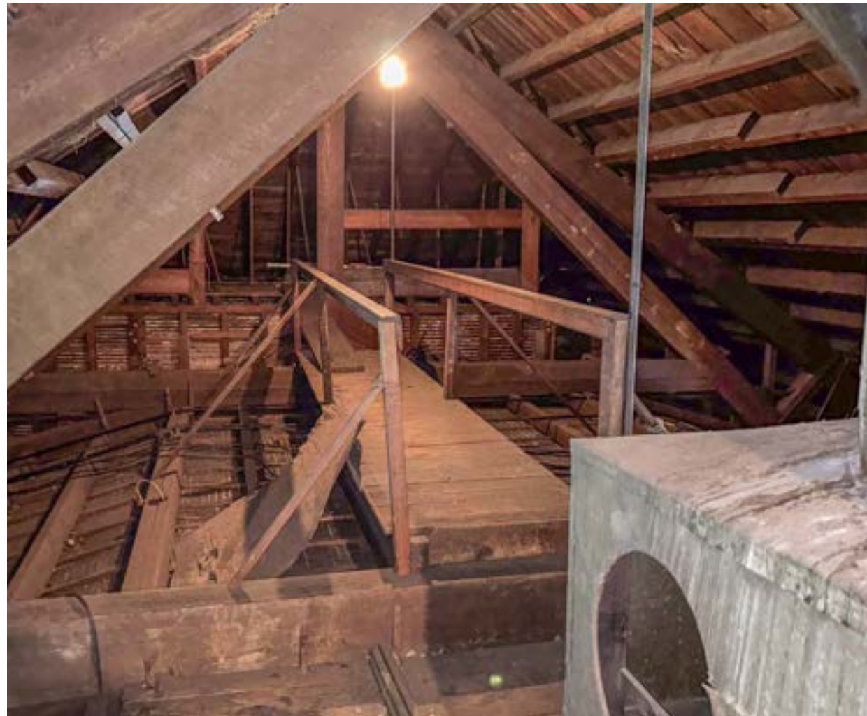
Figure 1. View of attic catwalk and furnace. Note trusses, exposed rafters, and outline of auditorium roof.
