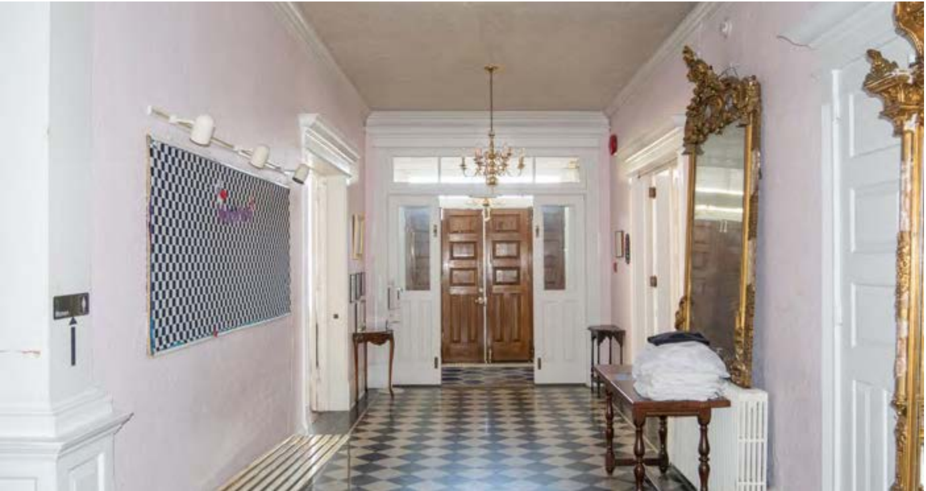
Figure 7: View of lobby, facing towards entry doors on Delaware Avenue. Note cornice molding, transom windows on entry vestibule and paneled doors, 2024 (DCT Studio Group)
