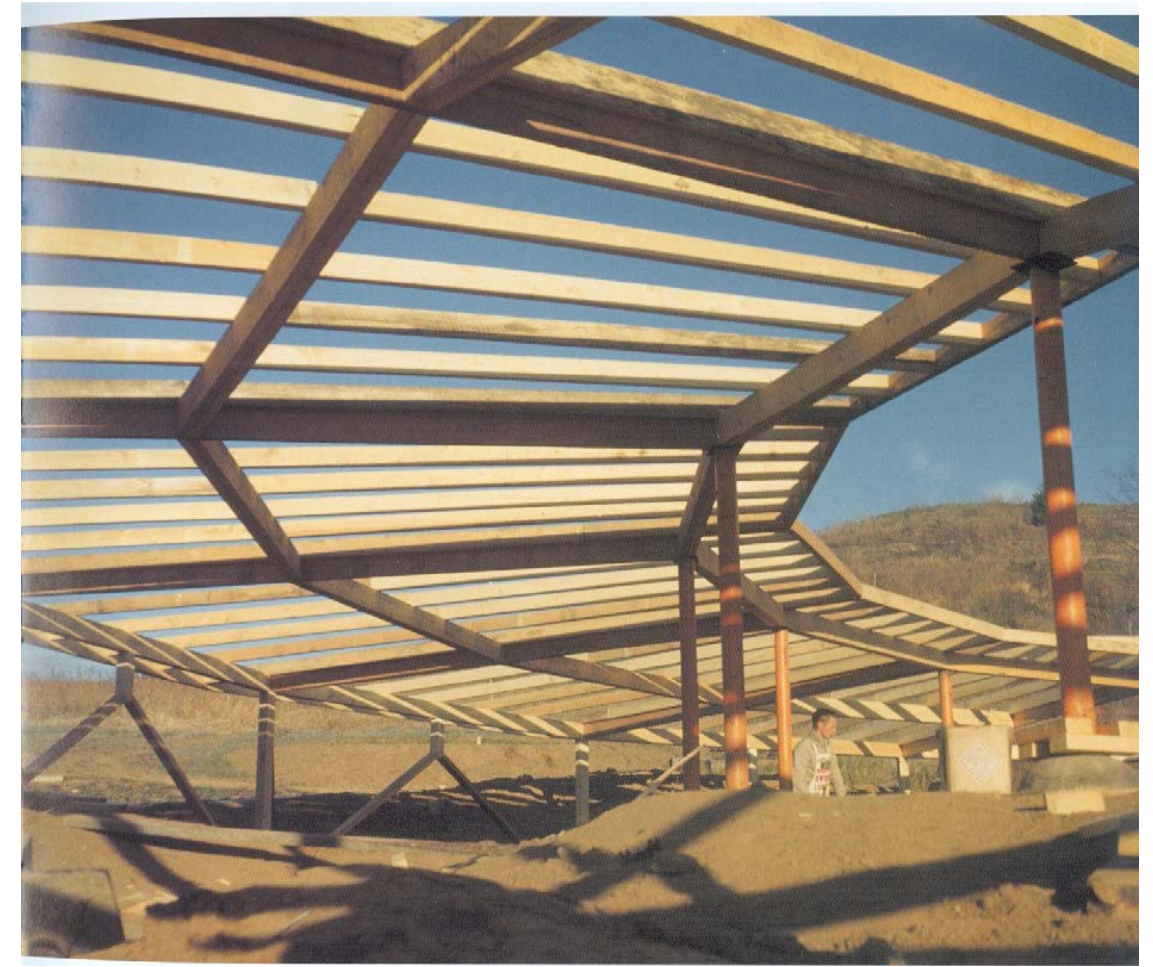
1948 - Machine shed initial construction, looking west TPI #1800. Davidson Gottlieb collection
