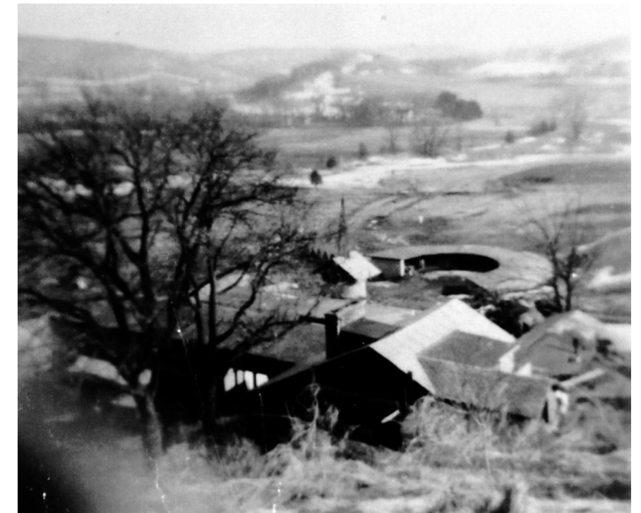
Post 1948 , Shed viewed from above facing east
