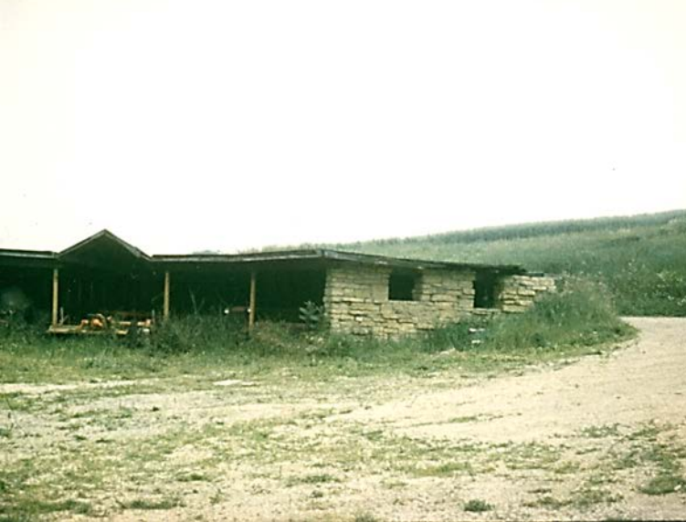
Post 1948 , Shed with roof modification
