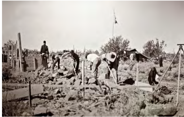
1938 Apprentices clear the desert for sun trap, the first structure on site. (Source: Taliesin West Archive, "Construction Taliesin West" historic photo collection.)
