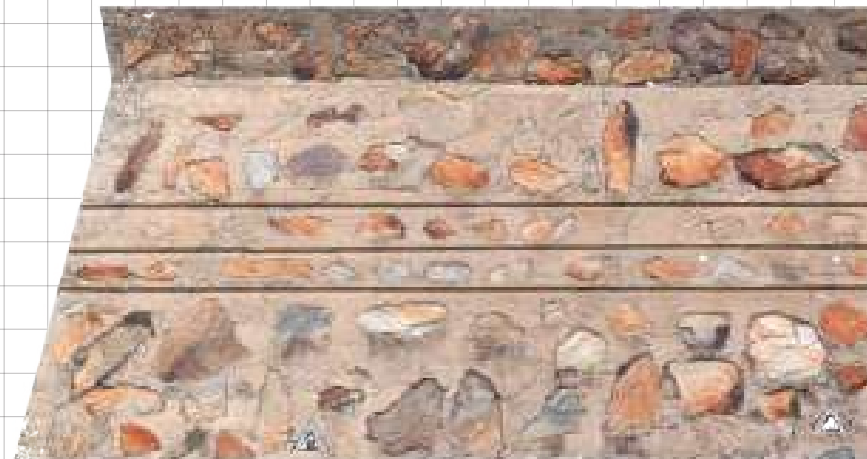
25-c-Admin Office-outer wall
