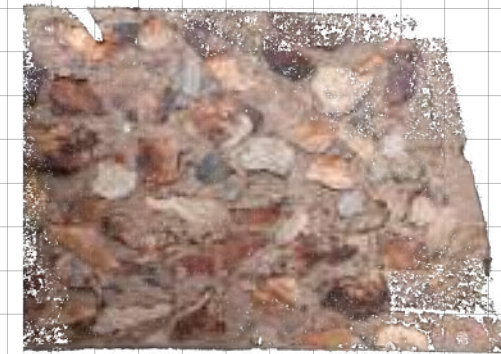
26-c-Admin Office-inner wall
