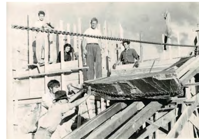
Figure 2.1. Transporting face stone using ramp. (Source: Taliesin West Archive, "Construction Taliesin West" historic photo collection.)
