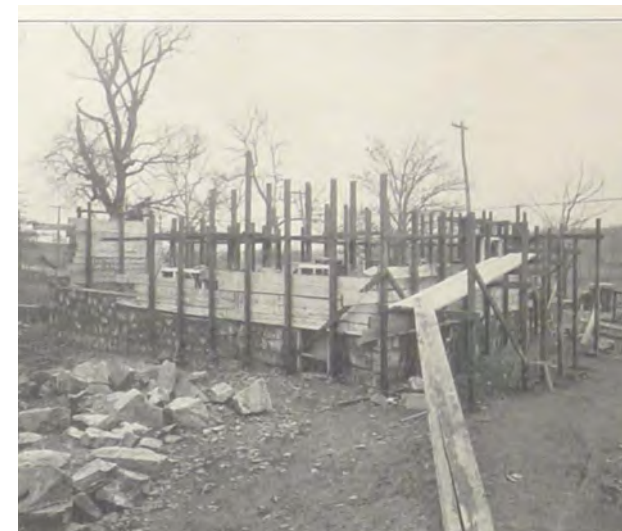
Figure 5.1. Slip-form rubble construction (Source: Ernest Flagg, Small Houses: Their Economic Design and Construction , 1922. Internet Archive)
