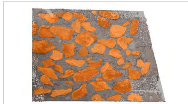
26-c-Admin Office-inner wall
