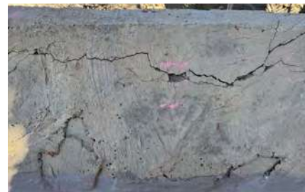
Figure 4.21. West bridge parapet (Source: photos by authors)
