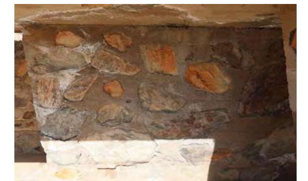
Figure 4.13. Kiva east addition west elevation (Source: photos taken by authors)
