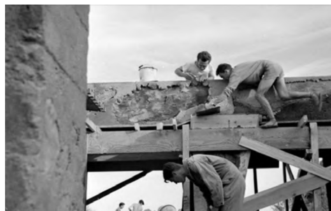
Figure 2.8. Stripping wood forms. (Source: Taliesin Fellowship – Pedro E. Guerrero. https://guerrero-photo.com/portfolio/taliesin-fellowship/ .)
