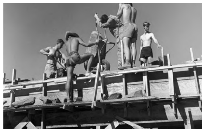
Figure 2.7. Packing concrete into forms. (Source: Taliesin Fellowship – Pedro E. Guerrero. https://guerrero-photo.com/portfolio/taliesin-fellowship/ .)
