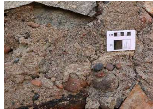
goose egg size concrete texture & aggregate
