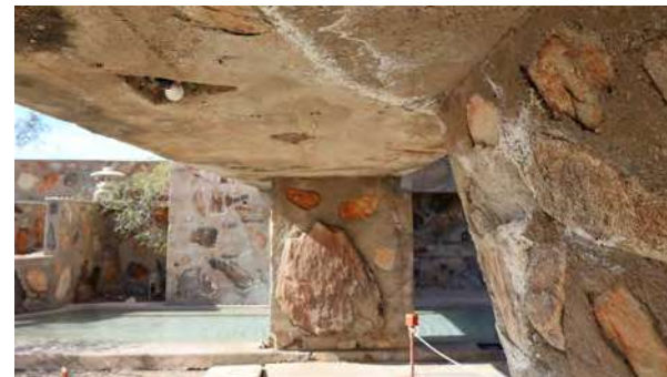
Figure 4.4. Underside of the bridge (Source: photos taken by authors)
