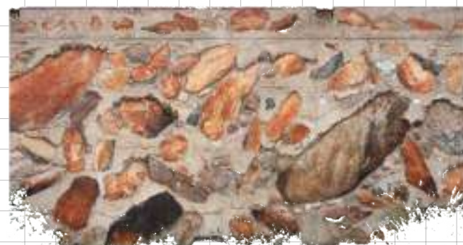
21-b-Men's Locker Room-wall
