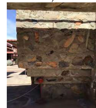
Figure 4.11. Kiva east elevation (Source: photos taken by authors)
