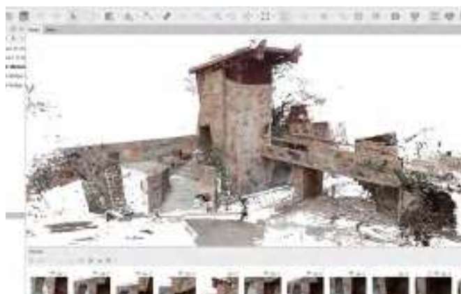
Figure 3.11. Building point cloud models of surveyed desert masonry structures using the photogrammetry software Agisoft. (Source: taken by authors)
