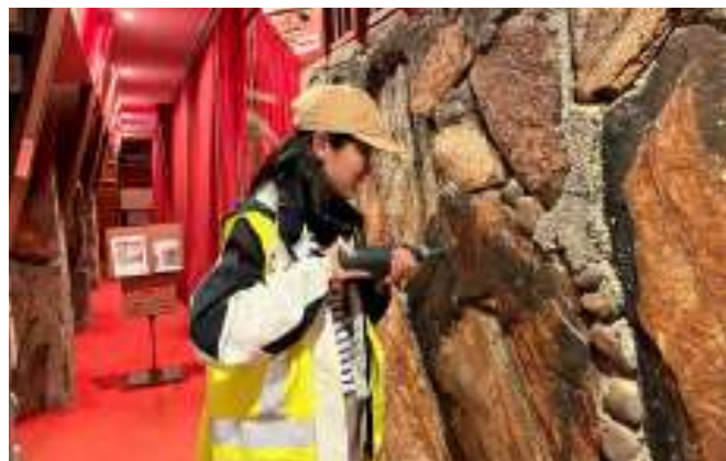
Figure 3.10. Measuring compressive strength of face rocks using Schmidt Hammer. (Source: taken by authors)
