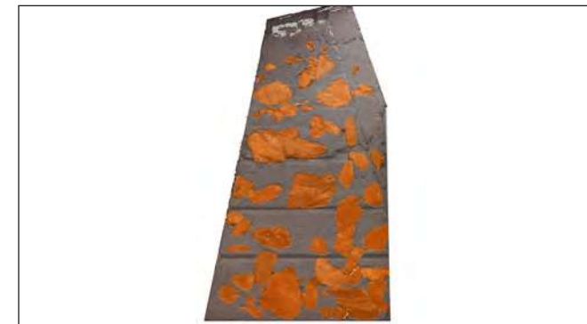
7-a-Drafting Studio- vault interior wall
