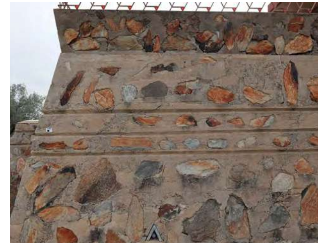
face rock size & density horizontal grooves
