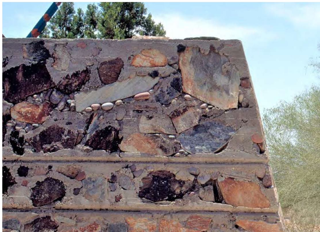
Close-up view of the Drafting Studio Vault, showing face stones, goose eggs and rustications. (Source: Atlas of Place, "Frank Lloyd Wright: Taliesin West, 1937–1959, 659AR")
