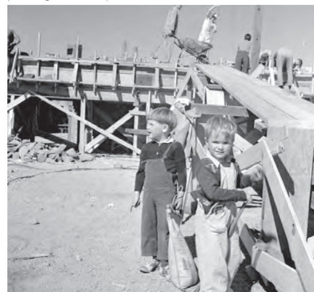
1947 Construction at Taliesin West, Brandoch Peters in the foreground. (Source: Taliesin Fellowship – Pedro E. Guerrero. https://guerreroportfolio.com/portfolio/taliesin-fellowship/ .)
