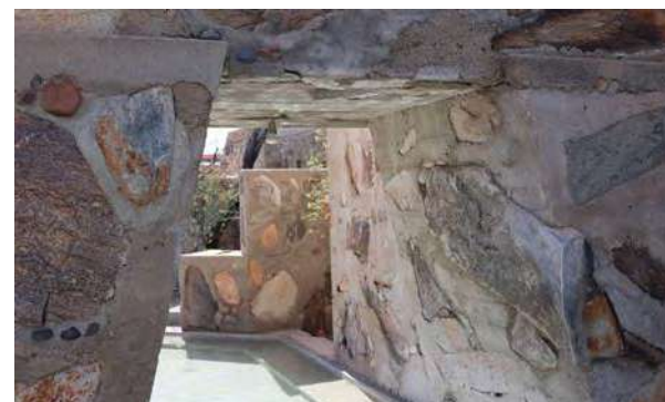
Figure 4.5. Bridge and column (Source: photos taken by authors)
