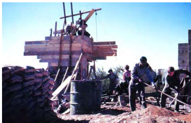
Figure 1.7. Chimney Construction at Taliesin West, 1949. (Source: Gottlieb, Lois Davidson. A Way of Life: an Apprenticeship with Frank Lloyd Wright . Mulgrave, Vic.: Images Publishing Group, 2001.)
