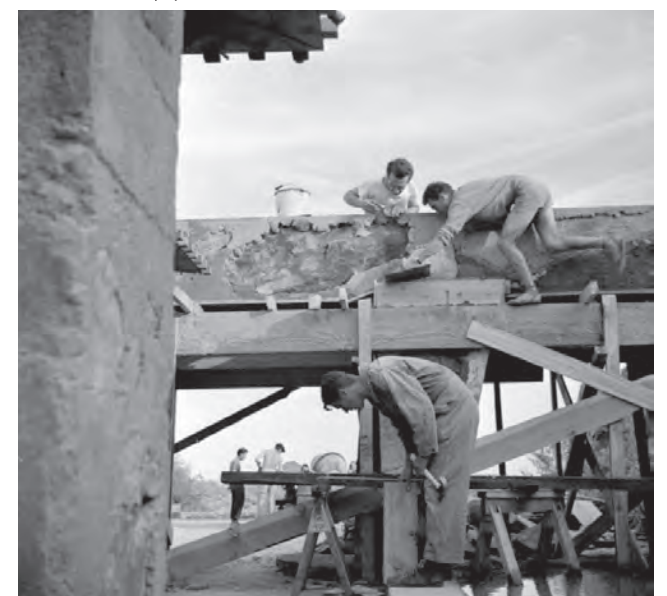
1947 Construction of Kiva bridge. (Source: Taliesin Fellowship – Pedro E. Guerrero. https://guerreroportfolio.com/portfolio/taliesin-fellowship/ .)
