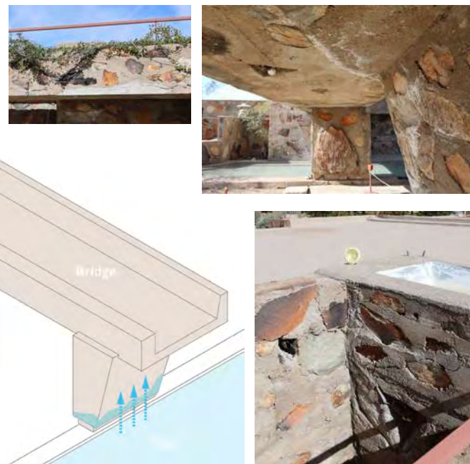
Figure 4.29. Diagram of water infiltration in the Kiva-Bridge area (Source: created by authors)
