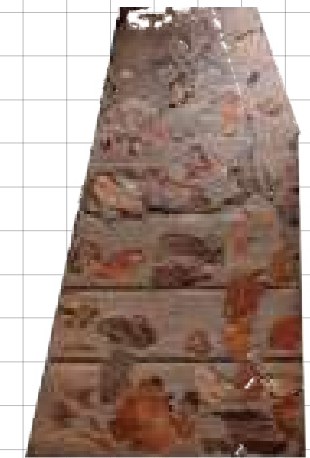
7-a-Drafting Studio- vault interior wall
