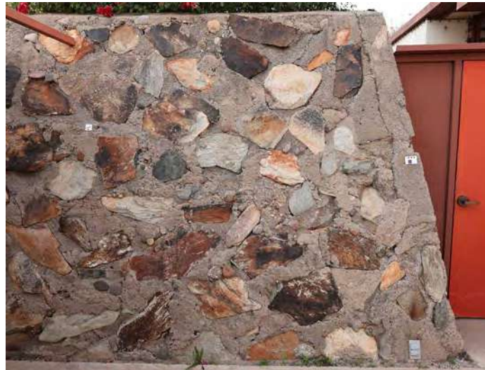
goose egg size concrete texture & aggregate
