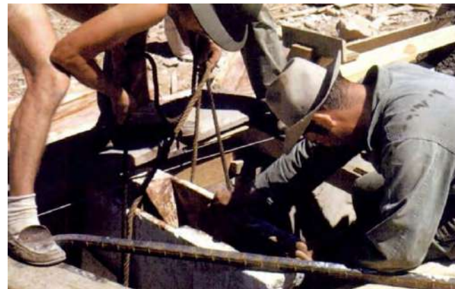
Figure 2.5. Lowering form into place. (Source: Taliesin Fellowship – Pedro E. Guerrero. https://guerrero-photo.com/portfolio/taliesin-fellowship/ .)
