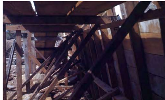
Figure 2.4. Formwork. (Source: Taliesin West Archive, "Construction Taliesin West" historic photo collection.)
