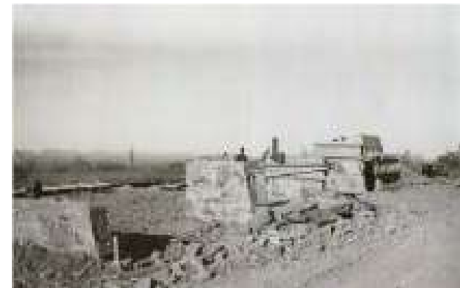
Figure 1.8. Construction of the Drafting Room piers and vault walls, showing the earliest concrete pours using slip forms. (Source: William Blair Scott. “75 Years at Taliesin West.” Journal of Organic Architecture + Design Volume 1, Issue 1, 2013)
