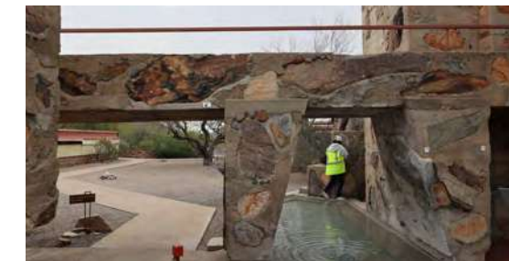
Figure 4.7. Bridge west elevation (Source: photos taken by authors)
