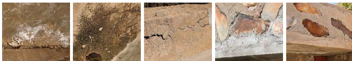
Figure 4.6. Desert Masonry condition glossary reference images (Source: photos taken by authors)
