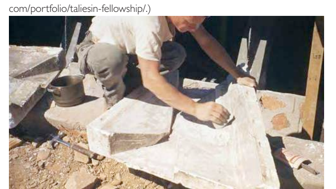
1948-1949 Construction of Cabaret. (Source: Taliesin West Archive, "Construction Taliesin West" historic photo collection.)
