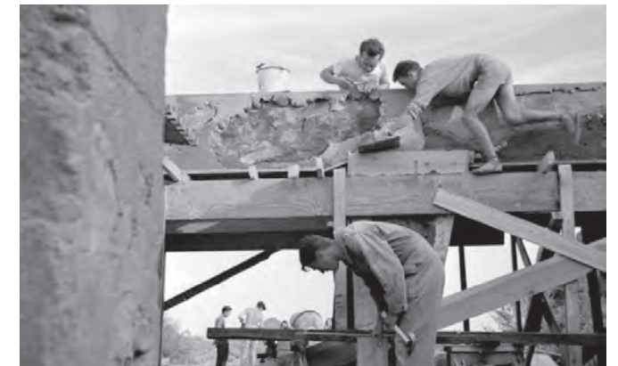
Figure 1.9. Construction of the Kiva Bridge, 1947. (Source: “Construction at Taliesin, 1947”, https://guerrerophoto.com/portfolio/taliesin-fellowship/ )
