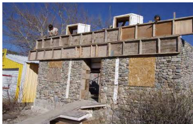
Figure 1.6. Traditional slip-form construction with mainly mortar-filled stones. (Source: “Forms are leap-frogged up the wall”, https://commons.wikimedia.org/wiki/File:Forms_are_leap-frogged_up_the_wall.jpg )
