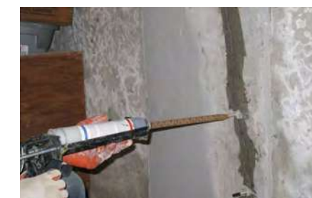
Figure 4.36. Grouting
