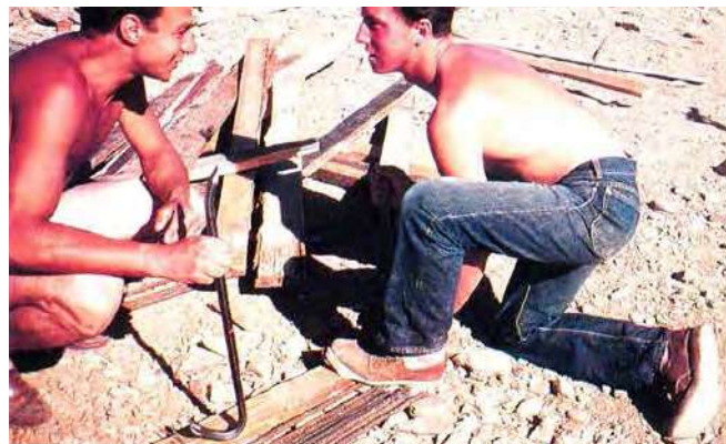
1948-1949 Fende and Paffard Keating-Clay Pulling nails from the boards so they could be used again. (Source: Gottlieb, Lois Davidson. A Way of Life: An Apprenticeship with Frank Lloyd Wright . I. publ, Images Publ, 2001.)
