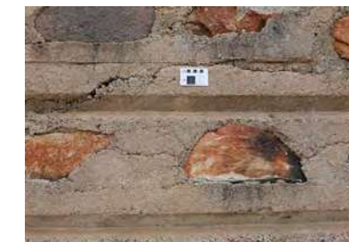
face rock size & density horizontal grooves
