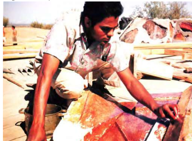
1948-1949 Mansinh Rana applying shellac to the forms for the Cabaret's concrete piers, so the concrete would not stick to them.
