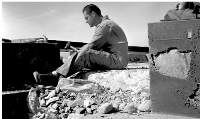
1947 Wes Peter (left) Construction at Taliesin West. (Source: Taliesin Fellowship – Pedro E. Guerrero. https://guerreroportfolio.com/portfolio/taliesin-fellowship/ .)
