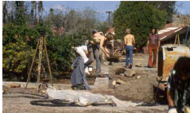
1963 Pavilion construction (Source: Taliesin West Archive, "Construction Taliesin West" historic photo collection.)
