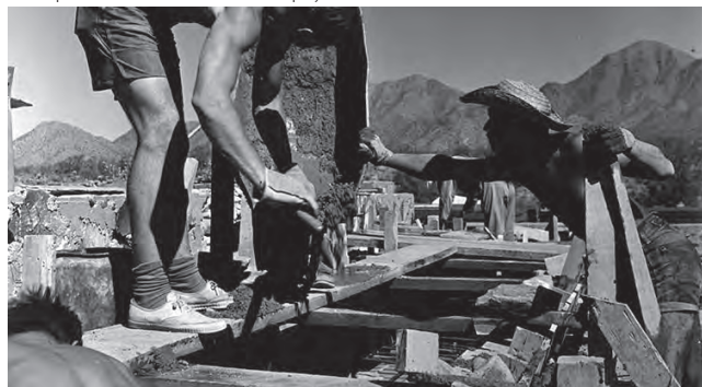
1940 Formwork. (Source: Taliesin Fellowship – Pedro E. Guerrero. https://guerreroportfolio.com/portfolio/taliesin-fellowship/ .)
