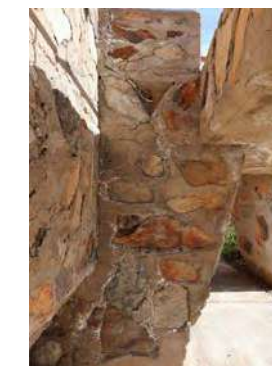
Figure 4.12. Kiva east addition south elevation (Source: photos taken by authors)
