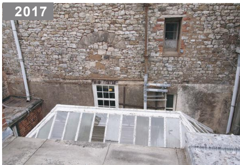
2017 At some point following Fowler's work, the open space between the Kitchen and the southern buildings was enclosed. This likely coincided with the demolition of the back portion of the Grange, labeled on Fowler-era plans as the "Steward's Room." It was replaced by a rectangular addition that now houses the offices. A large skylight was inserted and the room is now called the Scullery. (Photo: Starr Herr-Cardillo)
