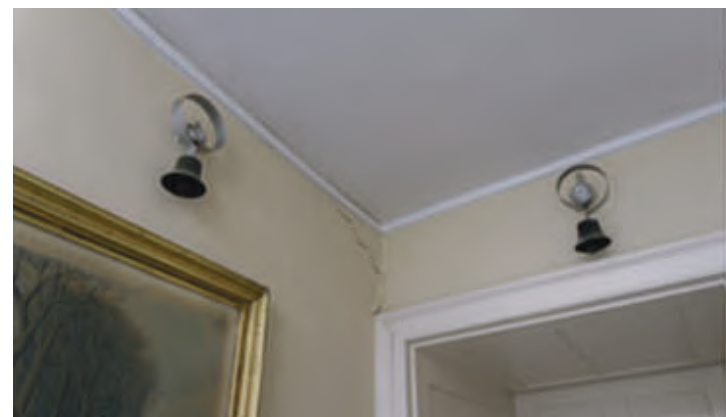
Figures 3 & 4: Bells in the hallway outside of the room correspond with bells in the kitchen of the private quarters. (Photos: Rebecca Clemente)
