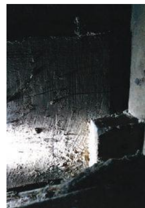
Figure 5: Pit saw marks visible on a floor joist. (Becca Flemer)
