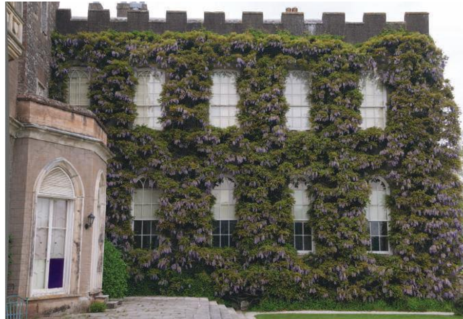
Figure 9: The south wall of the Libraries is covered with massive wisteria vines and render, making examination of the masonry walls impossible. (Photo: Dorcas Corchado)
