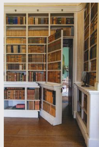
Figure 13: View of the jib door from the Second Library. (Photo: Starr Herr-Cardillo)
