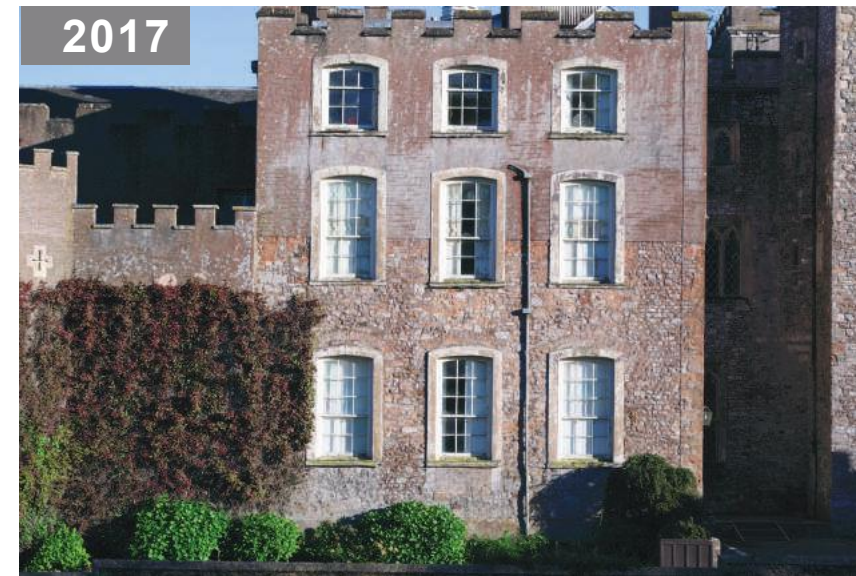
2017 The 30's Block added in the first quarter of the 18th century, retains its Georgian window configuration and window surrounds. The exterior walls of half of the addition are built of stone rubble with a reddish stone mortar and transition to rendered brick. (Photo: Starr Herr-Cardillo)
