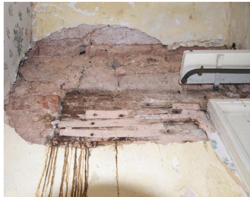
Figure 4: Large exposed wooden lintel in second floor bedchamber. (Image Credit: Allison King)
