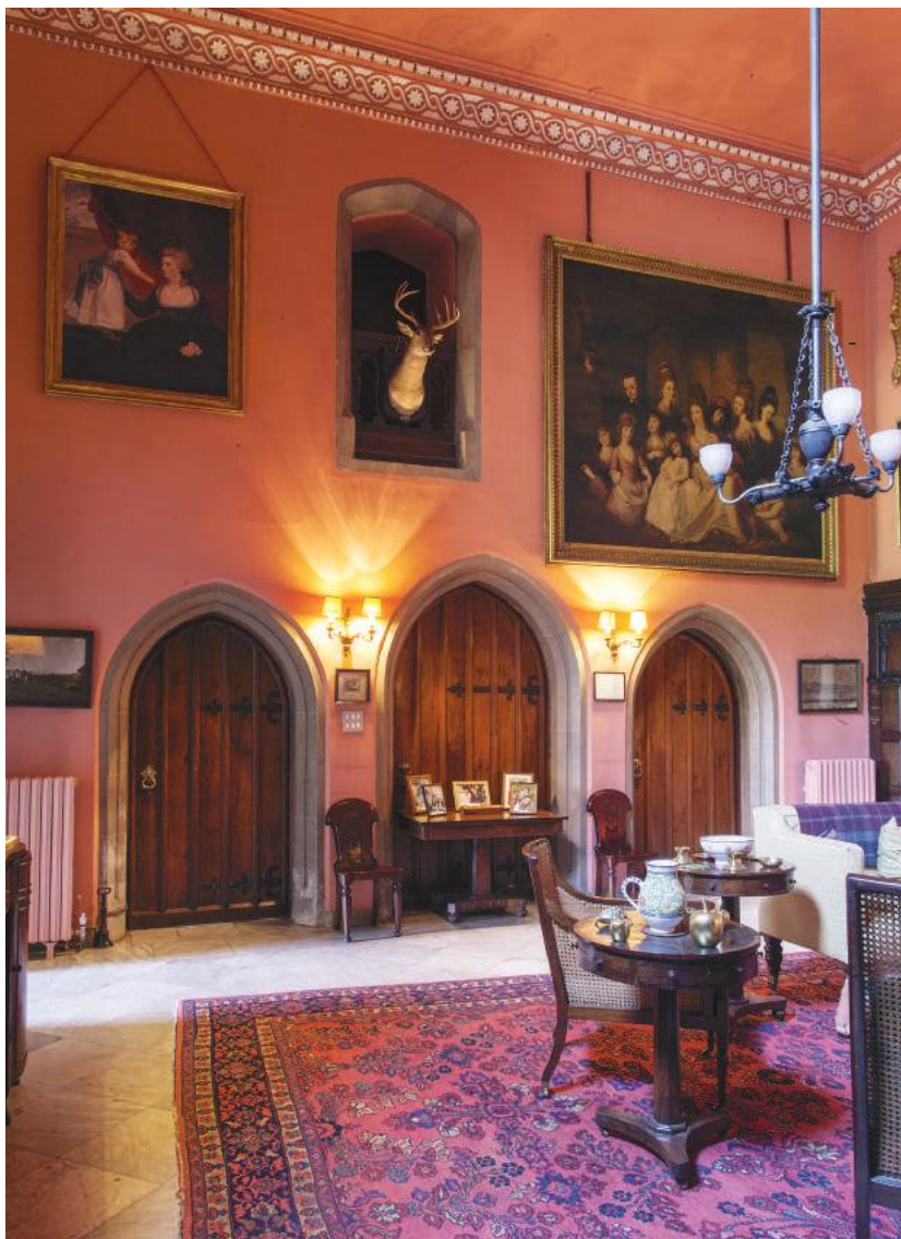
Figure 3: The three medieval arches referenced by Charles Fowler in his Account of Works at Powderham Castle. Fowler re-finished the arches in 1835; the right two doors are not functional due to a reconfiguration of the Kitchen in the private quarters, located on the opposite side. (Starr Herr-Cardillo, 2017)
