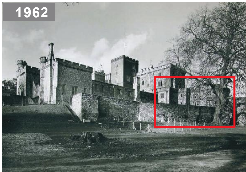
1962 This photograph shows the south side of the west court. Additions to the south end of the castle were made by Charles Fowler; the spaces now function as offices. (Historic England Archives)
