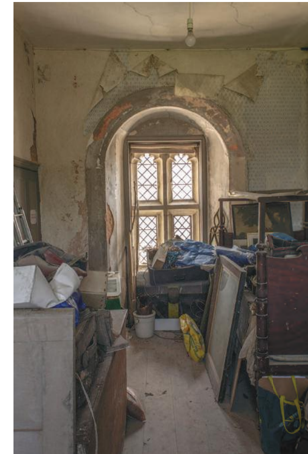
Figure 13: Two phases of paint visible in the third story of the North Tower's south side. The coloration of these phases matches the color scheme of the two layers of wallpaper also visible in the room. (Photo by Rebekah Yousaf)
