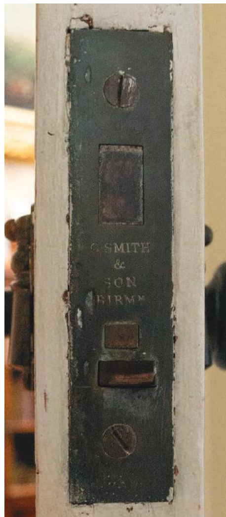
Figure 17: Mortise lock on the door between the Ante-Room and Rose Room (Photo by Mia Maloney).
