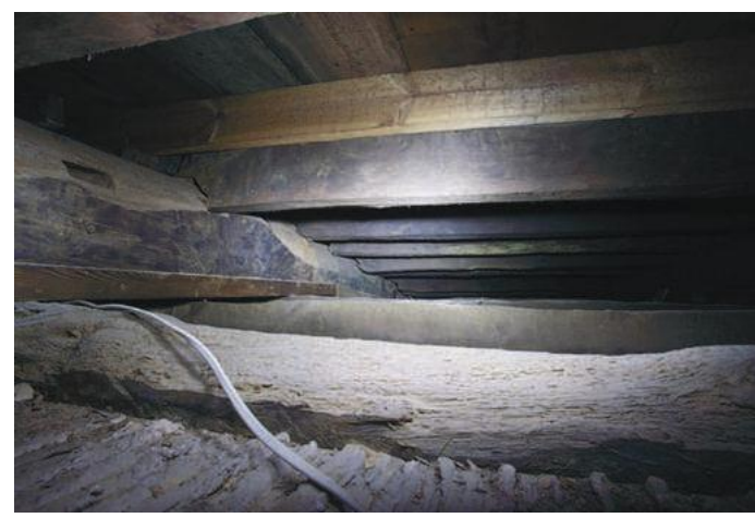
Figures 7: Ceiling beams visible through an access panel in the ceiling. (Photo: Starr Herr-Cardillo)
