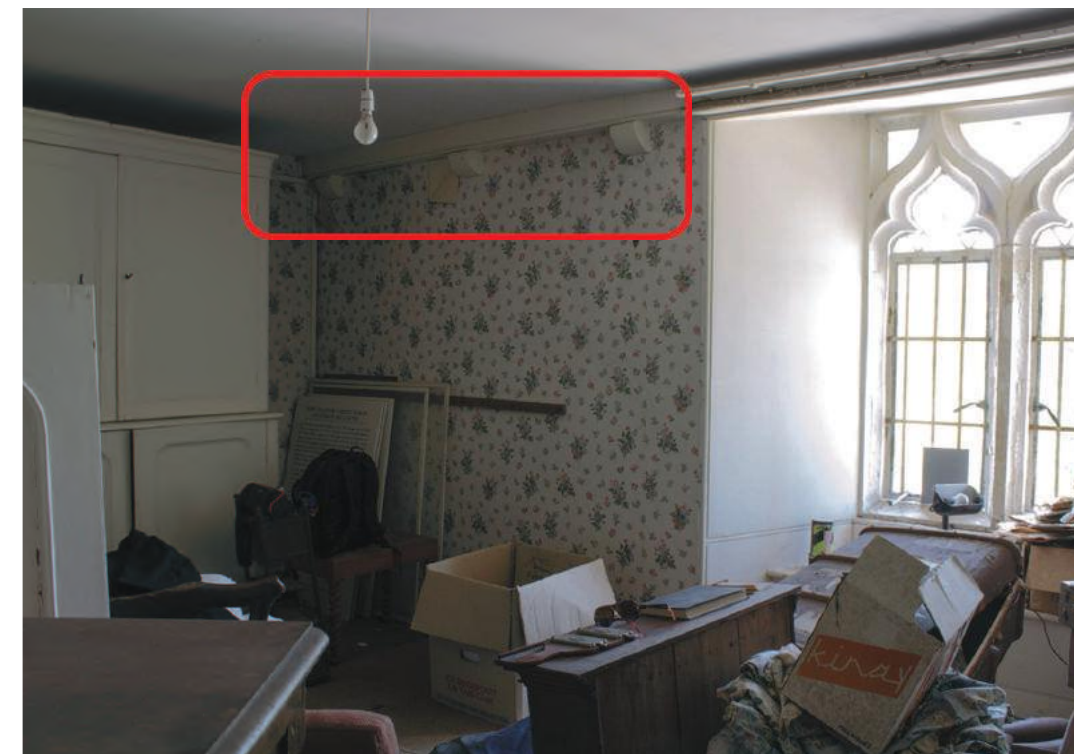
Figure 10: Corbels in the North Tower's second level, southwest corner, possibly hinting at an original pre-Fowler third story that was gone by Fowler's time. (Photo by Anthony Hita)
