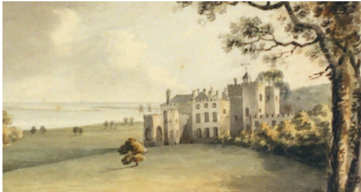
Figure 9: The central window and upper floor openings have not changed significantly since 1798. (Swete, 1798.)
