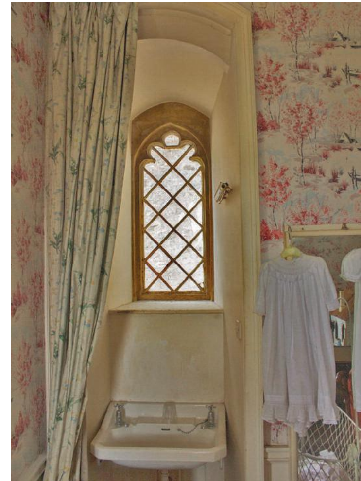
Figure 9: The possible location of a medieval privy in the northeast corner of the first level, now occupied by a modern sink. Fowler mentions removing an old privy and installing new water pipes in this room (IPhoto by Anthony Hita)
