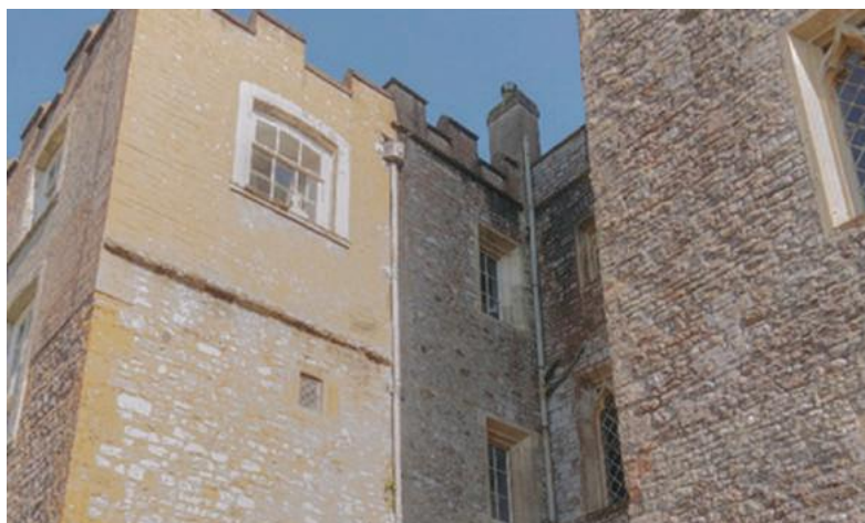
Figure 4: Exterior of the floors above the Hall (right of drainpipe), showing different masonry pattern, lack of string course, and higher crenellations. Also shows change in masonry between upper and lower floors to the right of the drainpipe, marked by string course. (Photo by Katherine Randall.)
