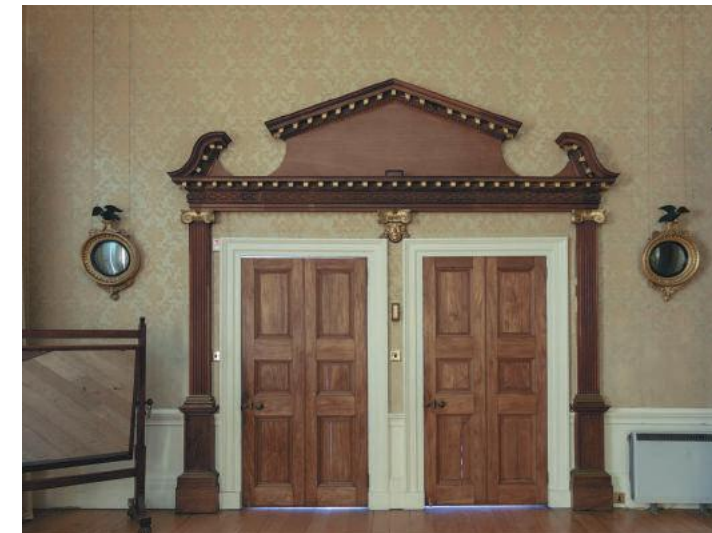
Figure 9: The door surround on the west wall was installed by Fowler to match the elaborate fireplace and provide access to rework rooms to either side. (Photo by Mia Maloney)
