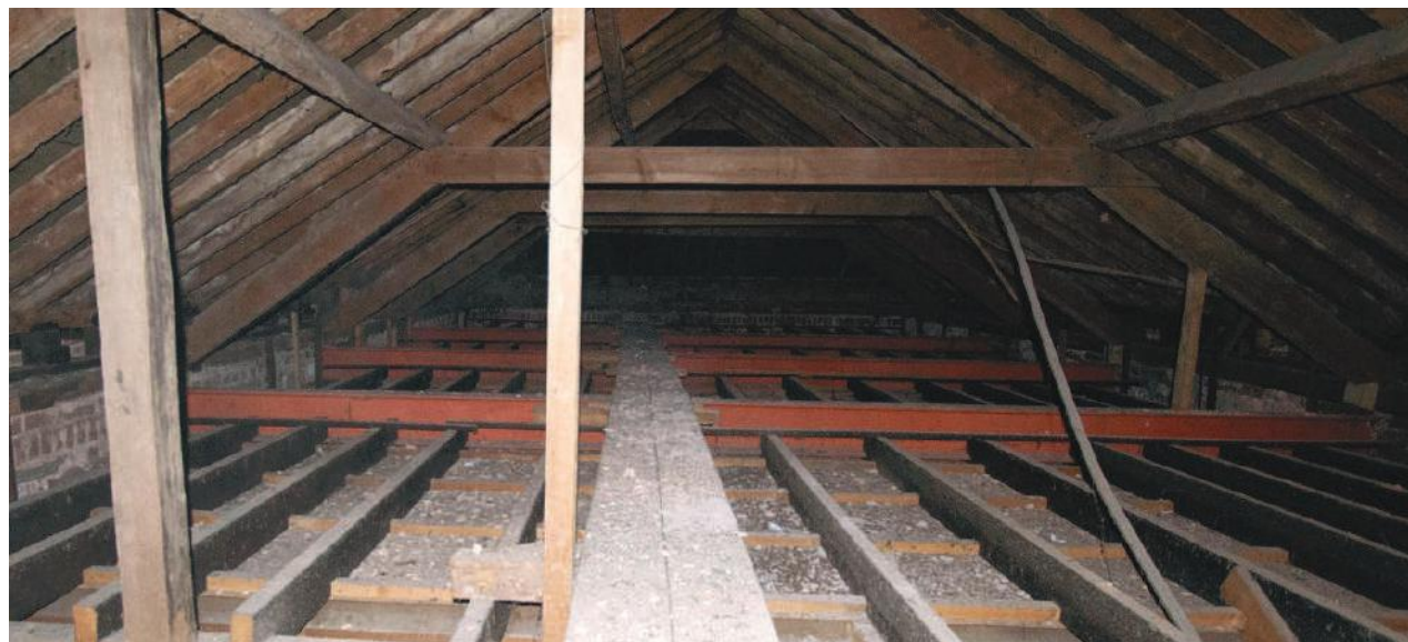
Figure 20: Steel beams over the State Bedroom (Photo by Mia Maloney).
