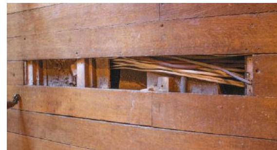
Figure 11: By removing some of the floorboards in the sitting room, we could discern that they were pit-sawn and observe the structure underneath. (Photos: Alberto Calderón-González)
