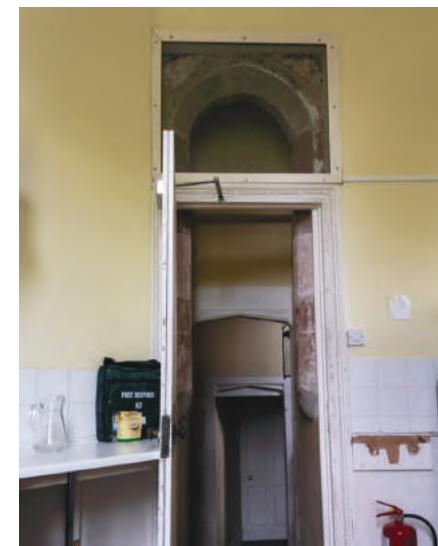
Figure 5: Red sandstone arch in wall between Hall and Kitchen. (Photo by Margaret Back.)
