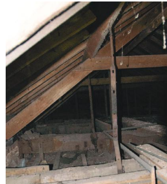
Figure 11: Metal straps connecting ceiling beams to trusses. (Photo by Mia Maloney)
