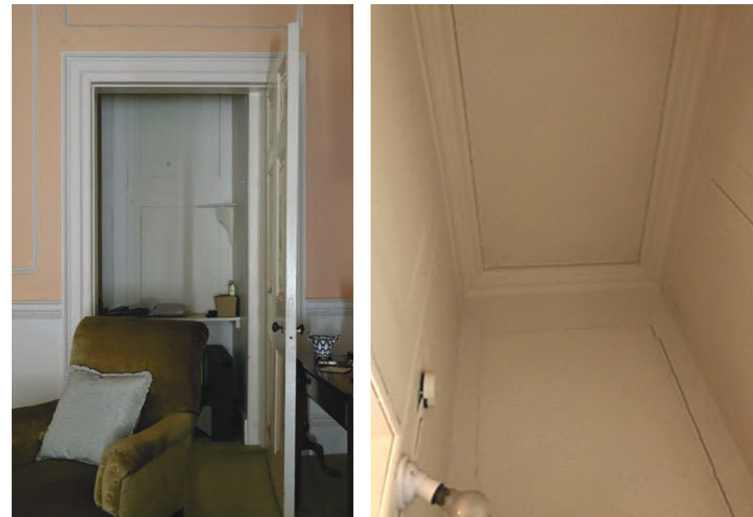
Figure 12: Inside the White Drawing Room there is a closet built into the stone wall of the medieval structure. The closet is not aligned with its door, and is much taller than is necessary (Figure 12); this strongly suggests that the closet was inserted into a major opening in the wall – it is the tallest opening encountered in our investigations thus far. Given that this was originally the main façade of the castle, we speculate that it may have possibly been an entrance to the Great Hall. (Photo: Alberto Calderón-González)
