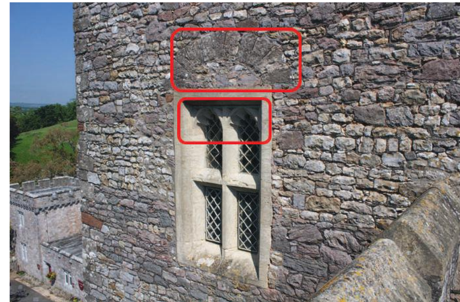
Figure 3: The exterior of the North Tower's third level southern wall showing a medieval arch above the window that Harding claims was uncovered and restored during Fowler's renovations. The trefoil caps appear to be a separate stone from the Fowler-added framing. A similar situation appears in-situ on the exterior west wall of the Stair Hall (Photo by Anthony Hita)
