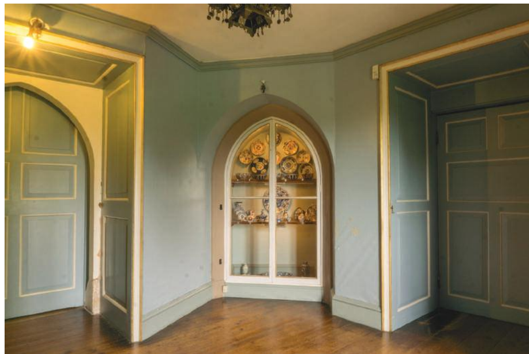
Figure 4: View of the tower stair entry-turned china cabinet at the northwest corner of the China Room. It is unknown whether or not the remnants of the Medieval newell stair remain behind the cabinet. (Photo: Zara Bhatti)
