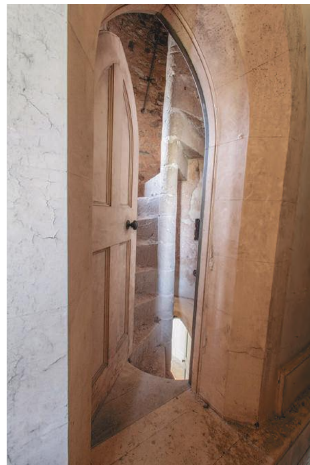
Figure 11: The opening to the spiral staircase on the east side of the North Tower connecting levels one through three. Fowler claims to have retained these openings to allow private access throughout the tower. (Photo by Starr Herr-Cardillo)
