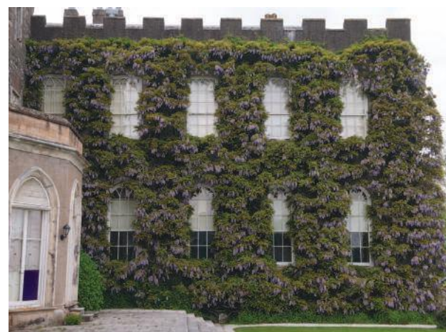
Figure 14: The exterior of the libraries is covered in an old-growth wisteria vine, making examination of the physical fabric a challenge. The walls have also been covered with a render, which obscures physical indications of building campaigns. (Dorcas Corchado)
