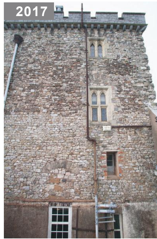
2017 A distinct change in stone rubble is visible on the south wall of the former medieval hall approximately 1/3 up the wall. A red sandstone arch indicates the presence of a medieval opening above a window in the Victorian Kitchen. Various arch campaigns are visible above the second and third story windows. The incongruous battlement, made of grey chert stone, was added by Fowler. (Photo: Starr Herr-Cardillo)
