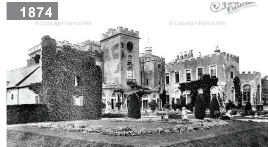
This photograph, taken from the southeast corner of the garden, shows a new, formal garden space off the east terrace. Some wear and patching are visible in the surface render on the tower and sections of dark brick are revealed in some of the patches. The overall window style and configuration appear to match earlier depictions of the central (East) tower, indicating that there was a later campaign that changed a number of the windows after Fowler's remodeling. (Francis Frith Collection)
