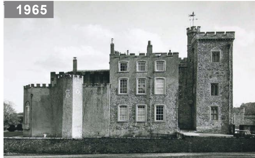
1965 This photograph shows the north wall of the Music Room with no indication of former windows. The crosses on the attached tower appear to have been modified, perhaps from the quatrefoils depicted earlier. A distinct line is visible on the 30's Block where the material transitions from rubble stone to rendered brick. Remnants of an elongated door surround are visible below the middle window in the first row. (Historic England Archives)
