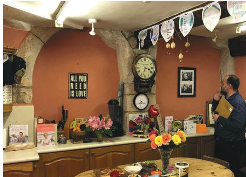
Figure 4: View of the same arches from the Private Kitchen reveals that they were constructed of rough hewn light red sandstone. (Alberto Calderón-González, 2017)
