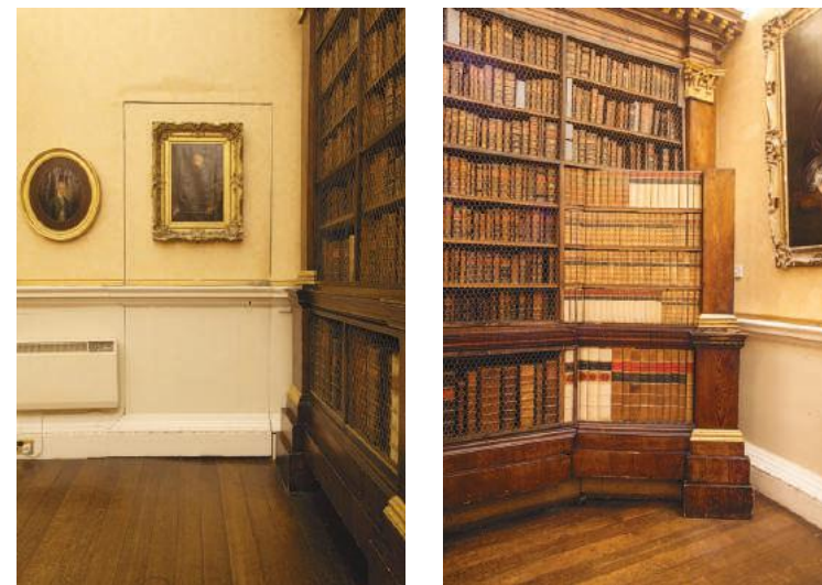
Figures 1 & 2: Jib doors lead to the first floor in the North Tower and to the Prep Kitchen. (Photos: Starr Herr-Cardillo)
