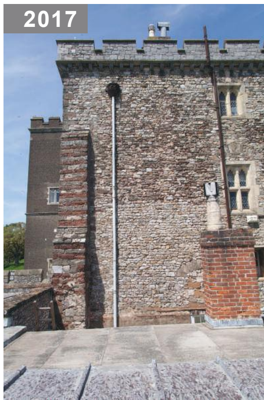
2017 This buttress, made of alternating bands of red breccia and light sandstone, was pointed out by Charles Fowler in his Account of Works as a "very important support" for the castle. He repaired and re-stabilized the buttress while working on the office buildings to the southwest. (Fowler, 5-6) (Photo: Starr Herr-Cardillo)
