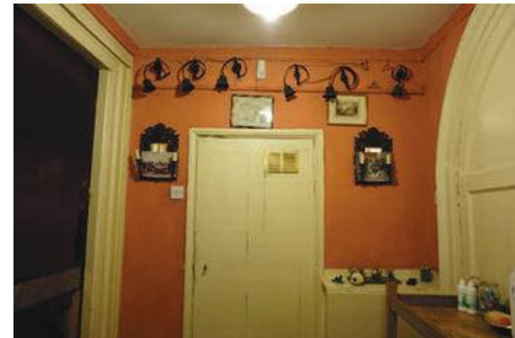
Figures 3 & 4: Bells in the hallway outside of the room correspond with bells in the kitchen of the private quarters. (Photos: Rebecca Clemente)
