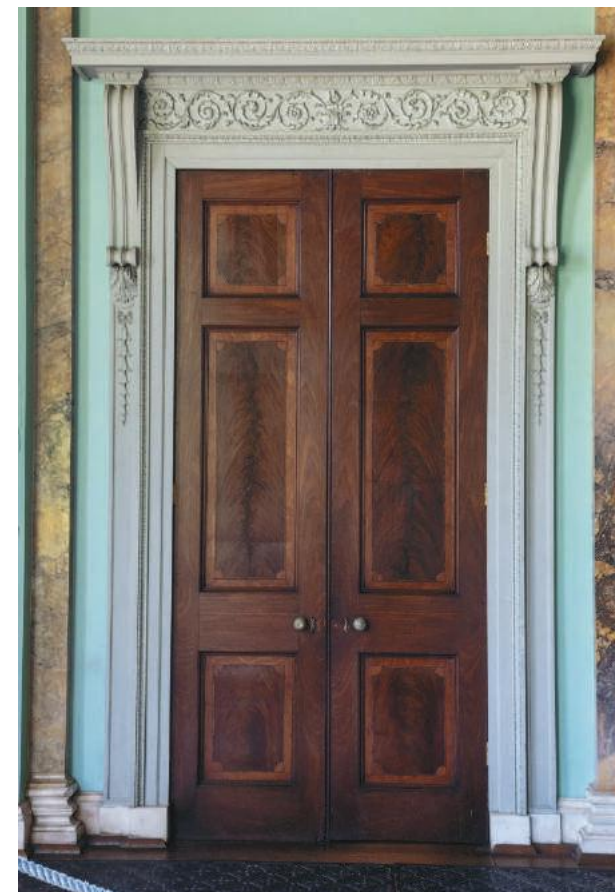
Figure 7: The easternmost door was likely a blind door, added to provide symmetry when Wyatt designed the room. It was later made functional by Charles Fowler. (Photo: Margaret Back)
