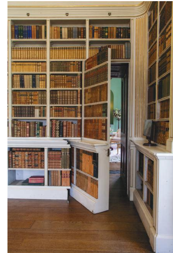
Figure 10: A jib door in the northeast corner bookcase, added by Charles Fowler, leads into the Music Room to the north. (Photo: Starr Herr-Cardillo)
