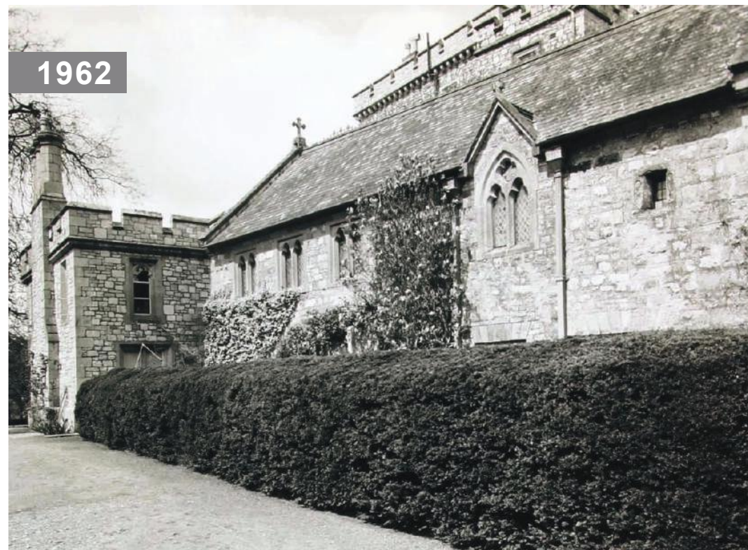
1962 The south wall of the Chapel (formerly the Grange) is constructed of the same irregular stone rubble as the medieval portion of the castle including the red sandstone quoining seen on other medieval portions of the castle. Lieutenant Colonel Harding suspected that the Grange and the original Chapel (in the location of the First and Second Libraries) were both built in the 1450s. (Harding, 176-177) A small and likely very early window framed in red breccia is visible on the right. The Grange was refitted into a family Chapel in 1861. (Historic England Archives)
