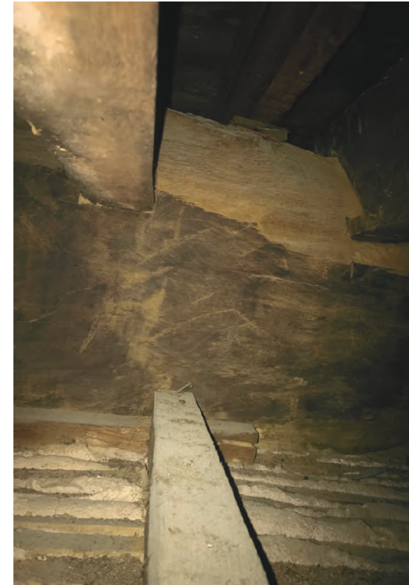
Figure 7: Mortise and tenon joinery from the ceiling of the medieval core above Room 17 (Image Credit: Allison King)
