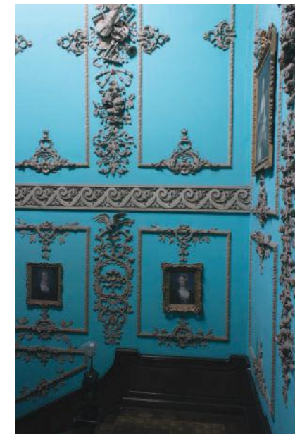
Figure 6: The "Vitruvian scroll" that runs along the south wall of the Stair Hall, ending abruptly at the west wall was mentioned in the original receipt of work. (Starr Herr-Cardillo, 2017)
