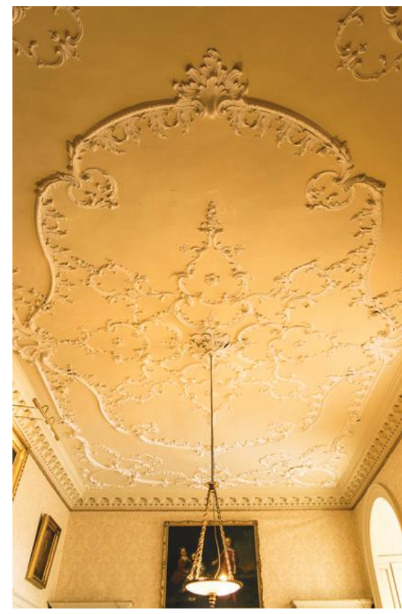
Figure 4: The fine rococo style ceiling found in the First Library. The ceiling experienced water damage and portions were replaced in the early 2000s. (Photo: Dorcas Corchado)
