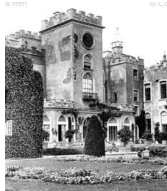
Figure 4: In this circa 1874 photograph of the East Tower, loss in the surface render on the tower reveals dark brick. The window style and configuration appears to match earlier depictions, indicating that there was a post-1874 renovation. (Francis Frith Collection)
