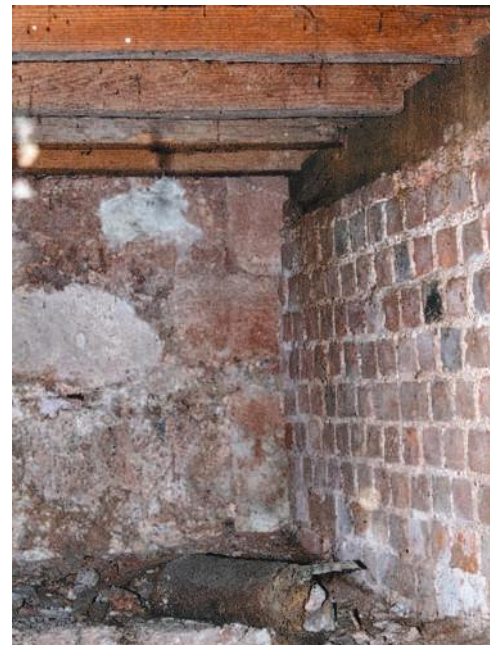
Figure 13: Image of the stone foundations found below the Second Library with indications of quoins. (Caroline Dickensheets)
