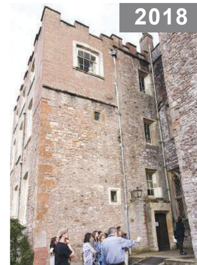
2018 On the west side of the 30's block a light stone belt course is visible at the juncture between the stone masonry and brick portion of the addition. A medieval tower, visible where the masonry extends to the roof to the right of the rain hopper, is embedded in the addition. (Photo: Starr Herr-Cardillo)
