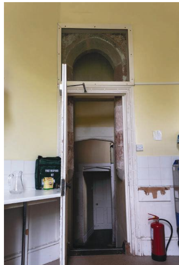
Figure 5: Remnants of a medieval door opening made of red sandstone are visible leading from the prep kitchen to the entryway. (Photo: Margaret Back)
