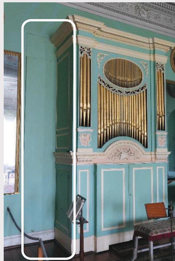
Figure 10: Closer inspection of the wall on either side of the Brice Seede organ reveals that an open space has been infilled by canvas panels. (Photo: Margaret Back)
