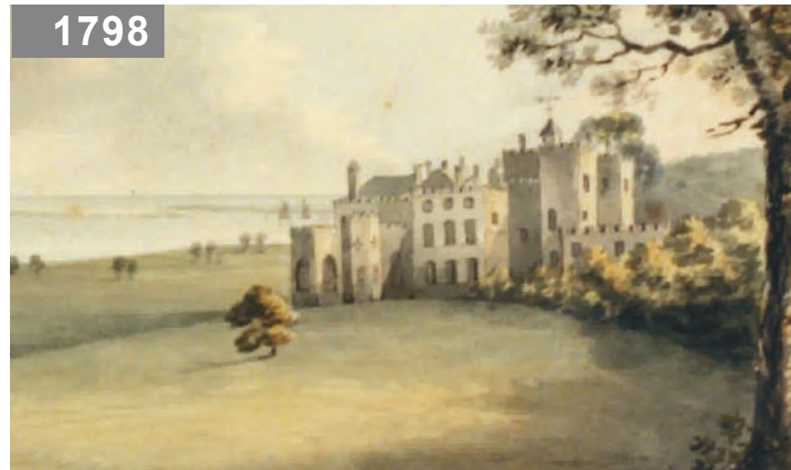
1798 Another view by Rev. John Swete provides a closer look. Large, arched windows along the north wall of the Music Room are clearly visible, flanking the three-sided attached tower, which also appears to have three small arched windows and decorative quatrefoils. There is no visible entrance on the north facade and there no longer appear to be formal gardens to the north of the castle, shown in the Whittlesby map from 1732. Powderham Estate Archives)
