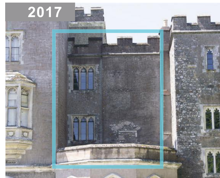
Figure 4: East elevation of Grand Staircase showing window infill. (Julia Cohen, 2017)
