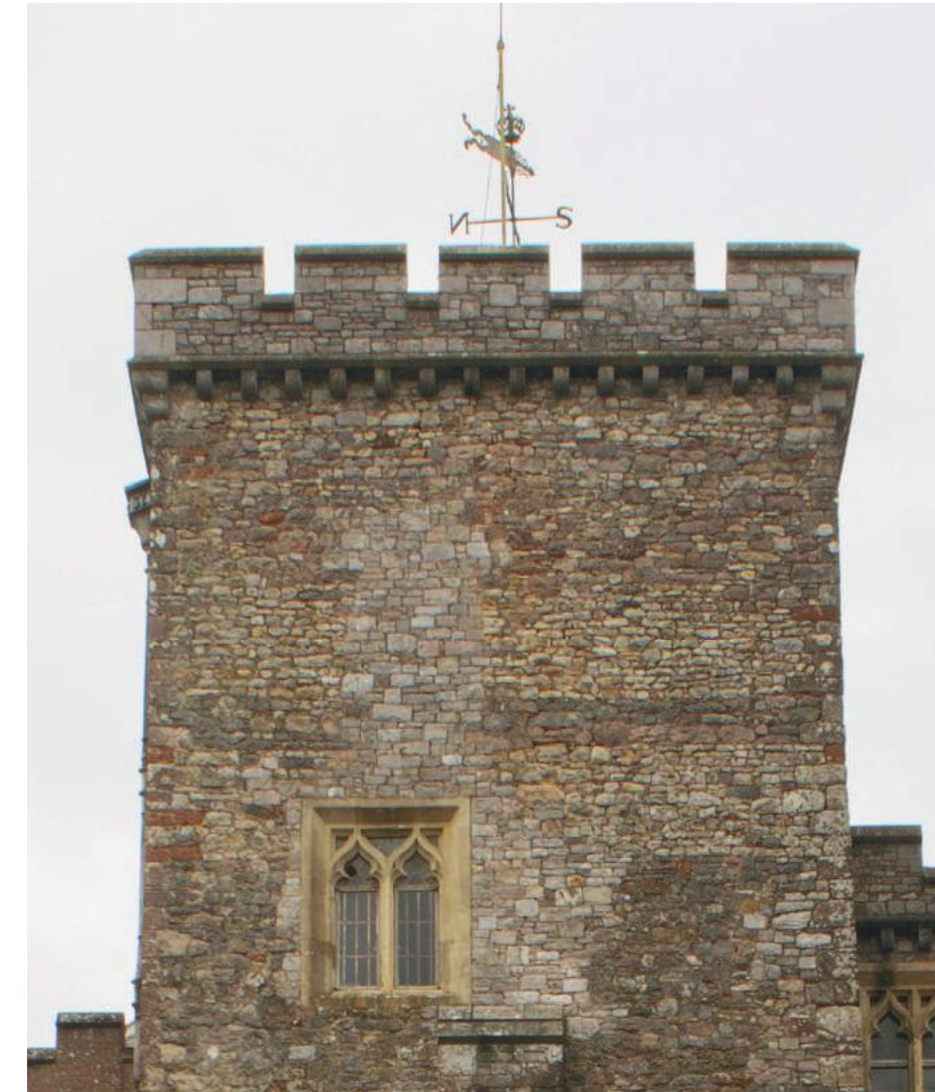
Figure 4: Evidence of a removed opening on the west side of the North Tower's third floor. Fowler placed a fireplace here, moving the window to the north side instead. (Photo by Rebekah Yousaf)
