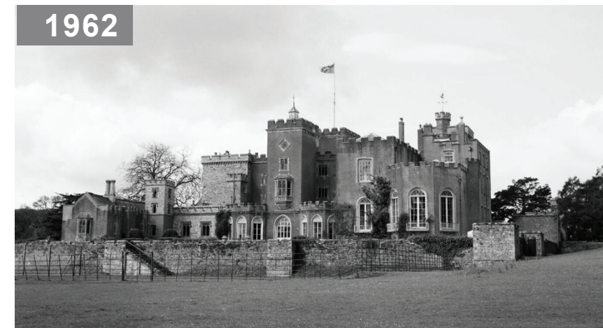
This view shows the terrace wall surrounding the garden east of the castle. The windows and clock on the East Tower and gable end of the chapel have been replaced with Gothic style windows and two oriels. The render on the East Tower's exterior also seems to have been repaired or replaced. (Historic England Archives)
