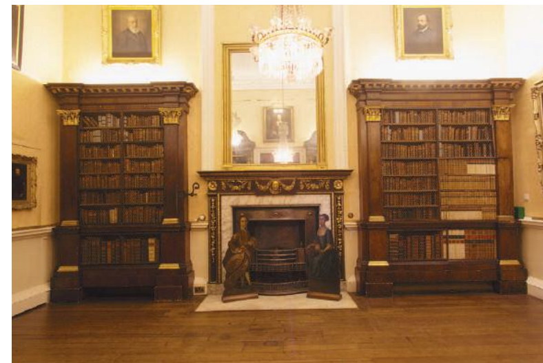
Figure 3: After adding the State Dining Room to the west of the space, a new window was needed to provide natural light. Fowler devised a sliding mirror above the fireplace which, when open, reveals a window. Photo: Zara Bhatti
