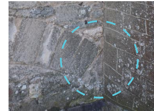
Figure 11: The very last stone in the relieving arch of the full Phase II arch is partially concealed by the west tower (shown intersecting in the photo), suggesting that the tower was a later addition that followed the second window campaign.
