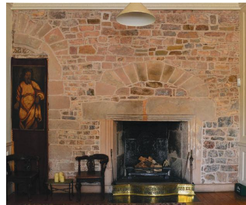
Figure 4: The exposed stone wall reveals the construction behind the Medieval-era hearth and a door opening to the left. (Photo: Zara Bhatti)
