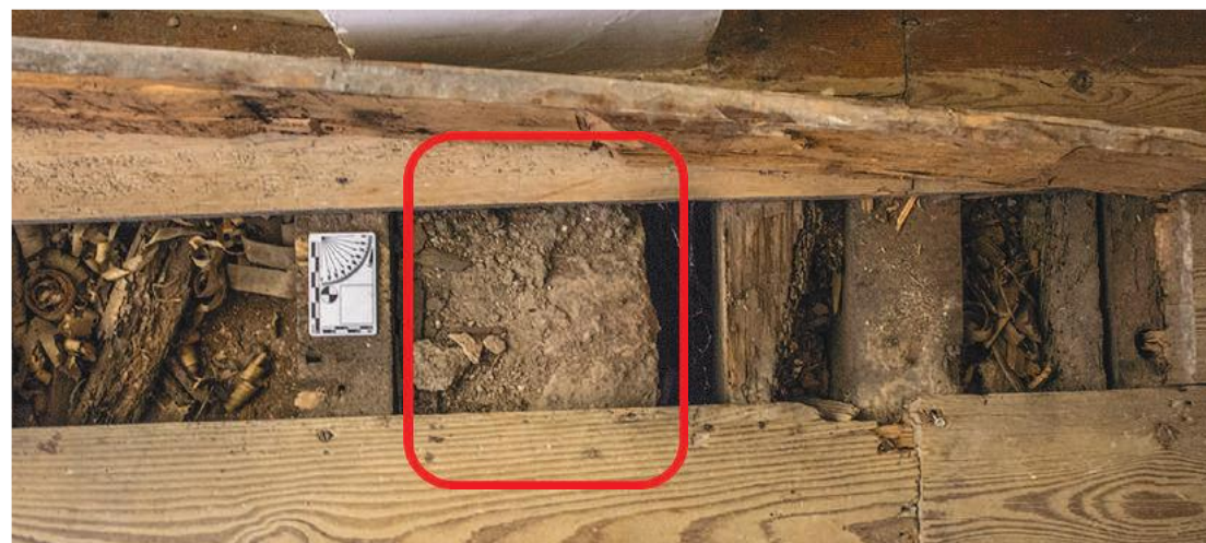
Figures 7-8: Evidence of Fowler's modification and medieval fabric under the floorboards in the hallway connecting the Dressing Chamber to the Solar on the southeast side of the North Tower's first floor. Top left: context for location. Top right: A possible medieval hewn timber cut by Fowler's floor joists. Bottom: A stone threshold, likely the medieval entrance to the tower. (Photos by Anthony Hita.)
