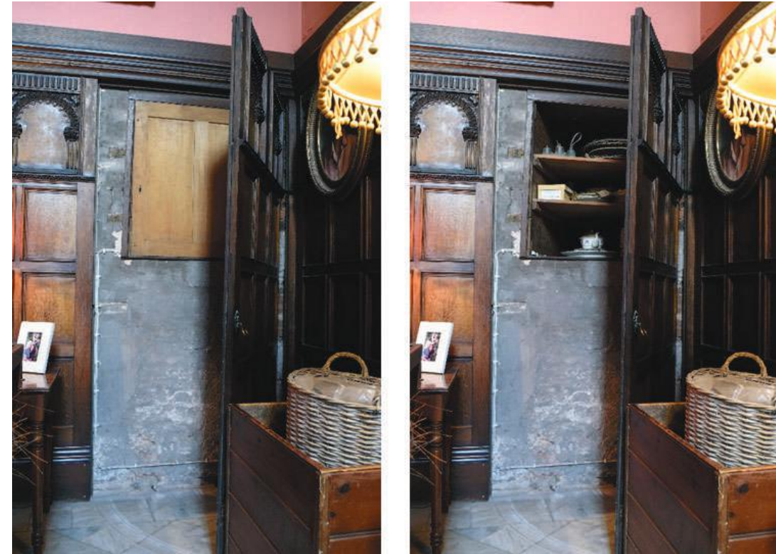
Figure 10: When the door leading to the cupboard on the west side is opened, a section of the medieval wall is exposed. This is a rubble wall covered in plaster, except the framing for the cupboard opening which is made of brick. On the right side of the opening there is a carved stone with cavetto moldings on both sides, which cannot be seen completely. This stone could have been part of an architectural feature such as a window or a fireplace, though it may not be in its original position. (Photo: Alberto Calderón-González)
