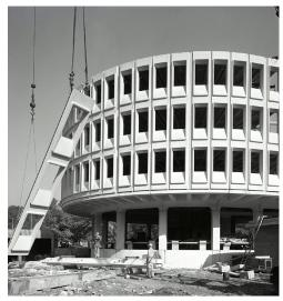
ARCHITECT Geddes, Brecher, Qualls, Cunningham ADDRESS 750 Race St, Philadelphia CONSTRUCTION TYPE Cast in Place, Pre-fabricated
