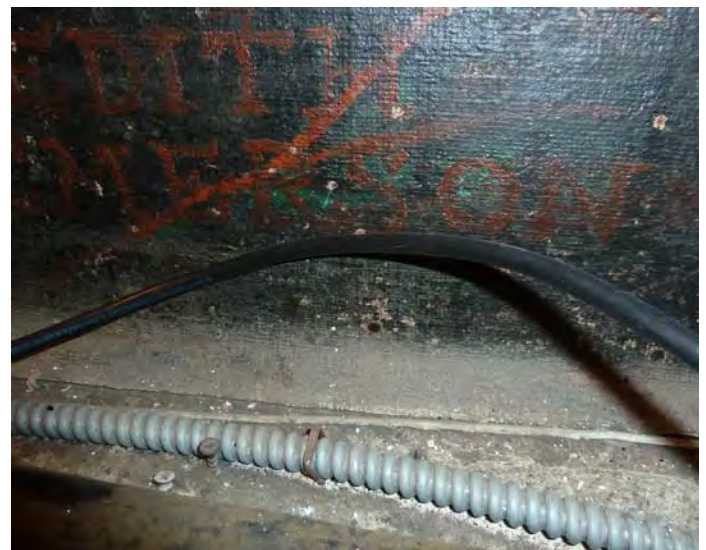
Photo. 3 Scratches on murals due to lighting wires (Photo taken by Jason Cantu)
