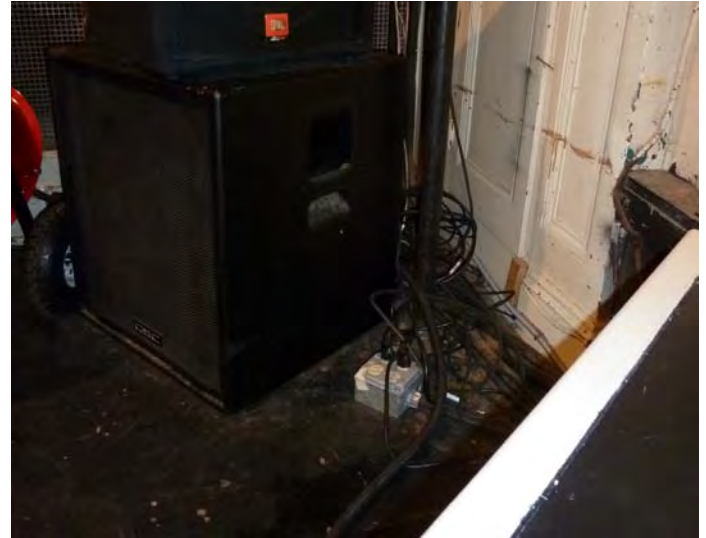
Photo. 2 Wires coming from below stage (Photo taken by Jason Cantu)
