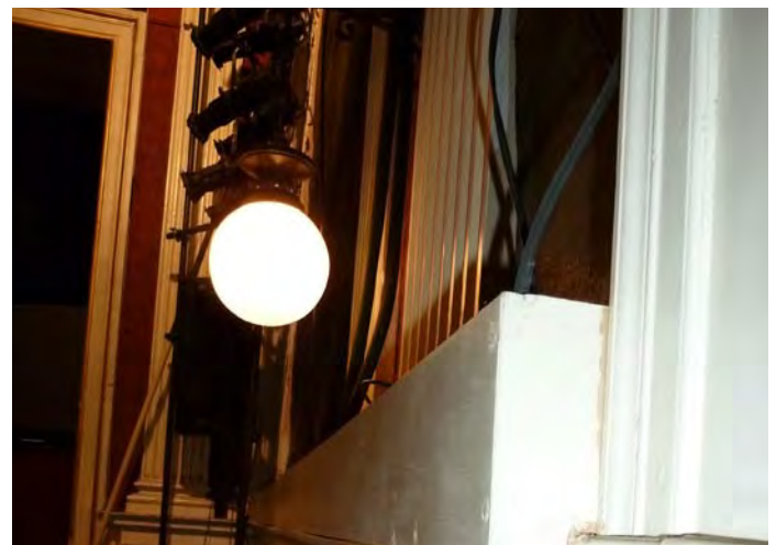
Photo. 4 Attempt to cover wires (Photo taken by Jason Cantu)
