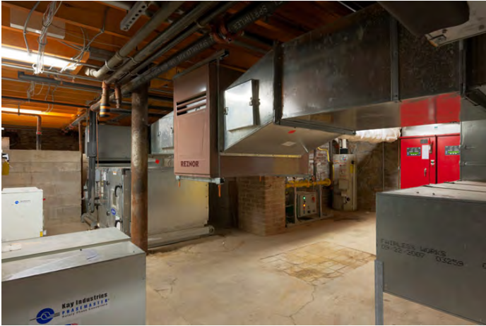
New HVAC System Source: Matthew Millan Architects, Inc.
