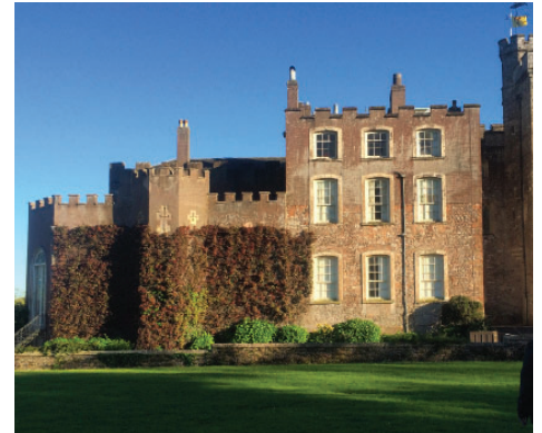
The addition to the North Wing is referred to as the 30's Wing. It is partially built of rubble stone (first floor) and rendered brick (second and third floors).
