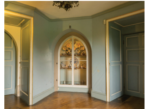
Past modifications, such as converting a medieval newel stair leading from the China Room to the Solar to a china cabinet, have altered historic fabric.
