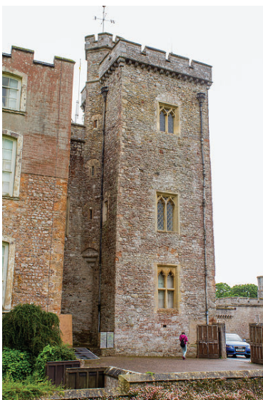
The northwest tower retains medieval-era window openings in the winding newel stair.
