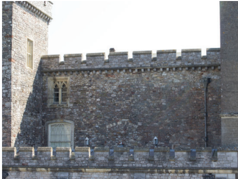
The walls of the original Medieval Hall were built with a distinctive rubble stone that can be differentiated from later additions made in brick and gray chert.
