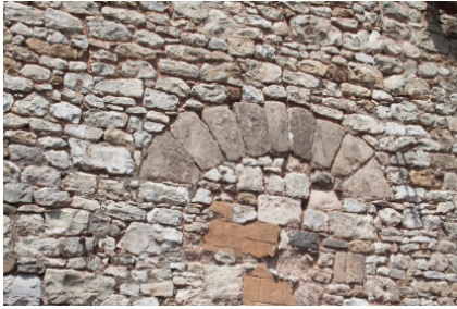
Evidential value relates mostly to physical fabric and its ability to yield scientific information. Pictured: an embedded sandstone arch indicates where original medieval openings were located.
