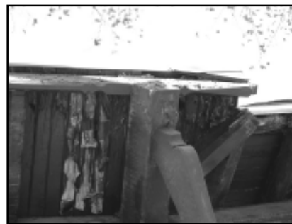
The underside of a porch roof, showing paint failure and wood rot.
