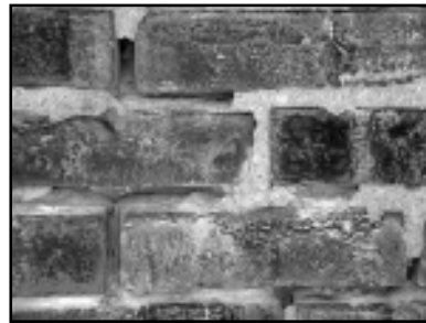
Mortar failure and spalling are results of water penetration.
