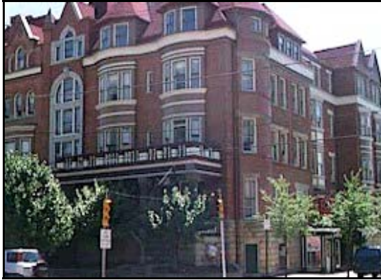
Powelton / The Courts Apartments
