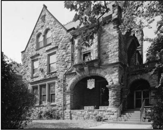
Burnham Mansion, architect T.P. Chandler, ca. 1890 (Philadelphia City Archives)
