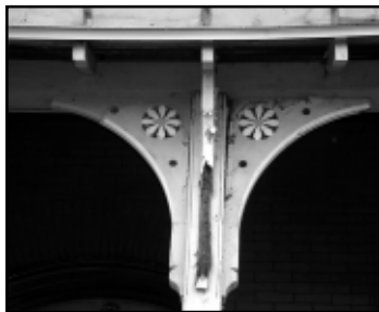
Deterioration of original wood decorative features.
