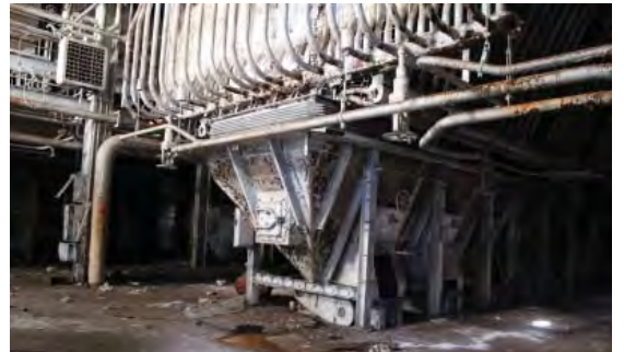
Firing aisle; skylights
