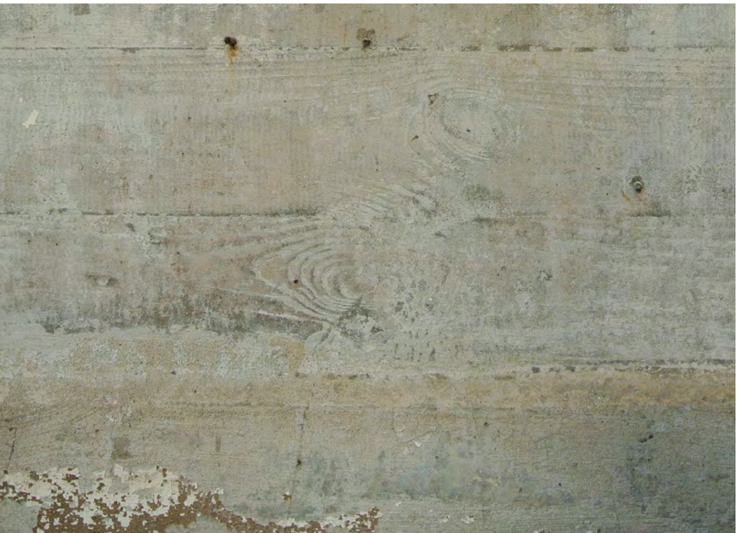
Image 2.8 - Detail of poured-in-place concrete, D. Pape, 2016.
