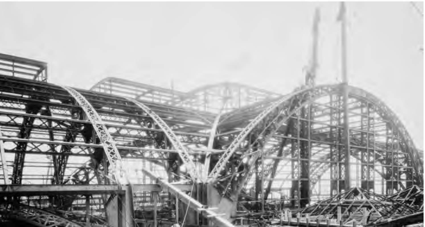
Image 10.2.3 - Historic view of the construction of the Turbine Hall roof, showing the steel structure, still intact today. (PECO Archives)
