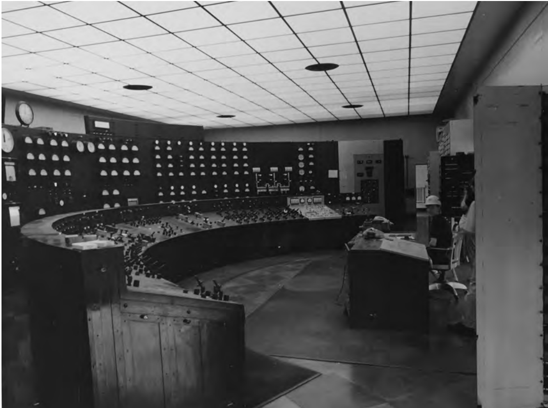
Shortly after the plant opened (c. 1927)
