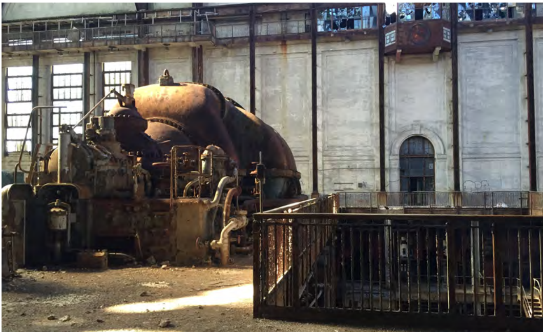
Image 9.8 - Interior of the Turbine Hall, Group Site Visit, Emily Gruendel
