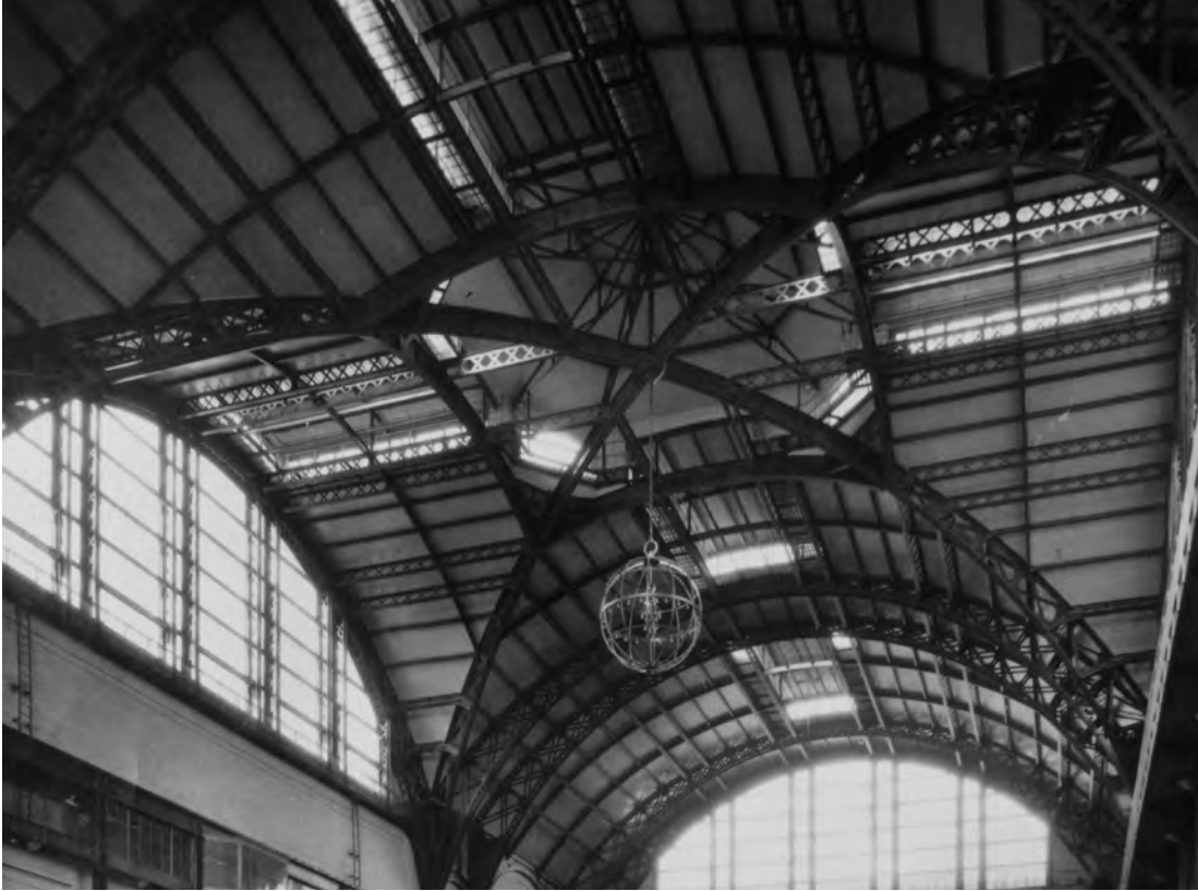
Shortly after the plant opened (c. 1927)
