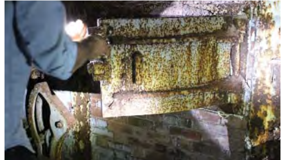
Boiler base, steam pipes
