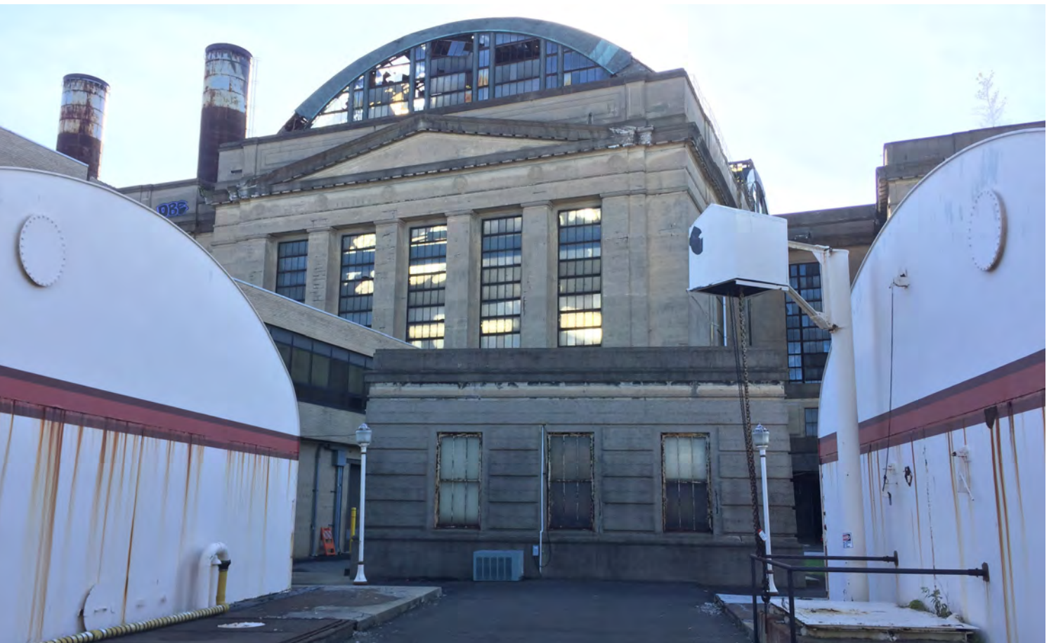
Image 1.2 - Turbine Hall exterior - E. Gruedel, site visit (2016)
