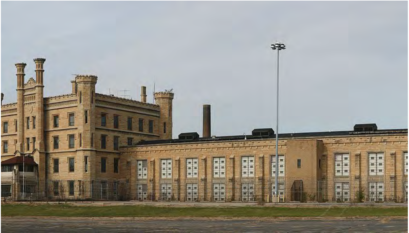
Image 7.6 - Joliet Correctional Center in Joliet, Illinois, Wikicommons.
