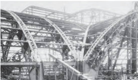
Image 5.20 - Detail, Richmond Power Station Folder at the Philadelphia Historical Commission
