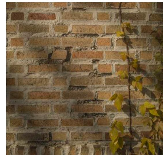
Figure 75. A darker, more granular mortar is revealed where the white repair mortar is deteriorating (Luo, 2018.)
