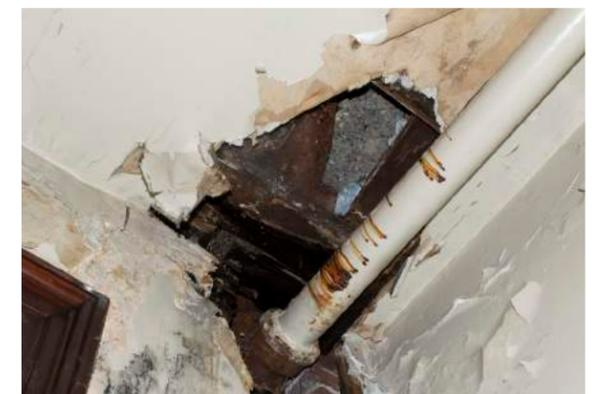
Figure 78. The interior finishwork will only be repaired once the envelope is watertight and survives at least one winter without leaks. (Luo, 2018.)
