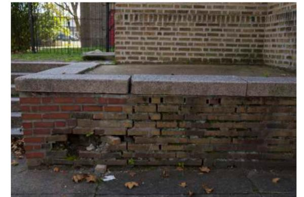
Figure 77. The deteriorated brickwork near the main entrance to the sanctuary will be a high priority. (Luo, 2018.)
