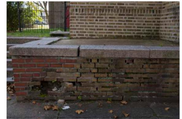
Figure 77. The deteriorated brickwork near the main entrance to the sanctuary will be a high priority. (Luo, 2018.)
