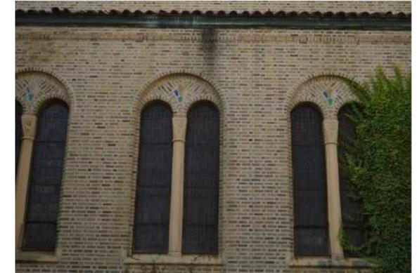
Figure 76. Staining shows where pipes blockages are. The ivy will be removed to prevent mortar deterioration. (
