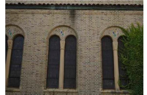
Figure 76. Staining shows where pipes blockages are. The ivy will be removed to prevent mortar deterioration. (
