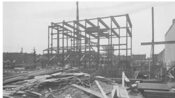
Figure 98. The steel frame at the structure’s base, covered by concrete and a brick envelope. Shown in 1926. (Philadelphia Department of Records.)
