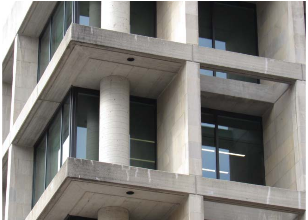
Concrete patina soiling and cleaning. Photo credit: Amy Lamb Woods
