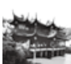
豫园修缮工程 Renovation of Yu Garden
