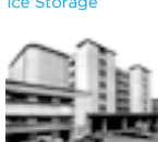
上海外贸冷冻厂万吨冷库 Shanghai Foreign Ice Storage
