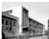
同济大学文远楼 Wenyuan Building at Tongji University
