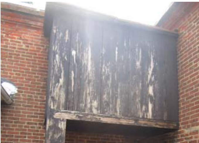
Outside view of the shadow box addition
