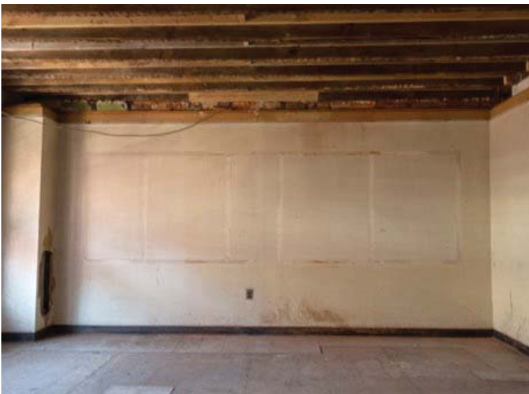
Most rooms have been stripped, with the floor joists now left exposed
