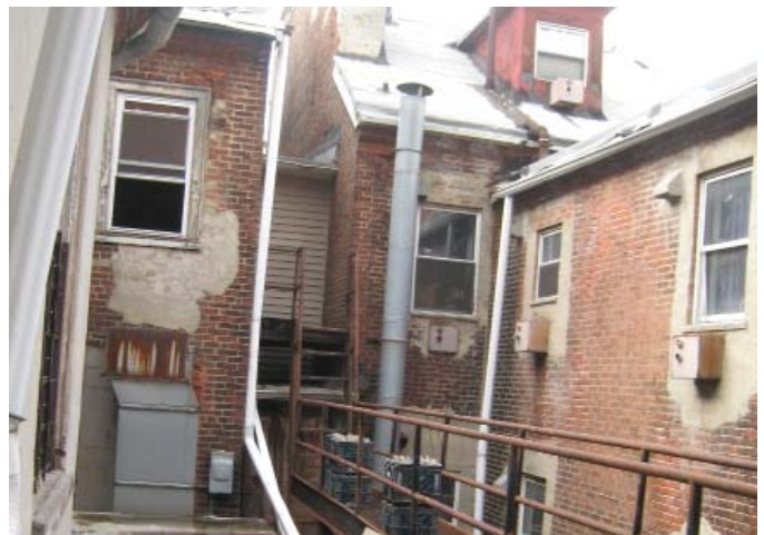
Fire escape and HVAC duct work outside the back portion
