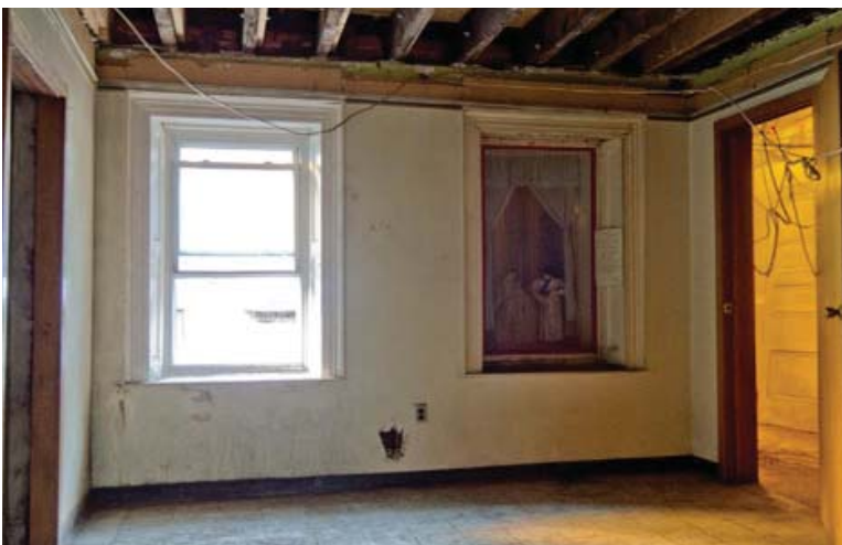
Most rooms have been stripped, with the floor joists now left exposed
