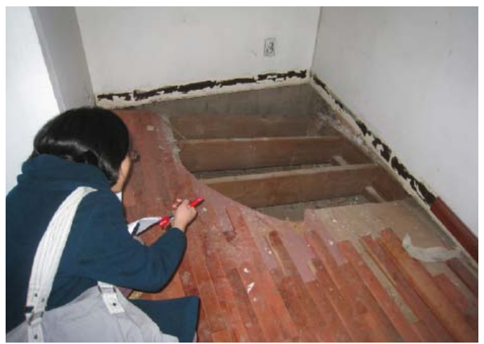
Collapsed floor boards in northwest corner on the first floor
