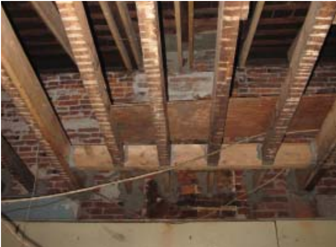
Vestiges of a chimney in the rear of the building
