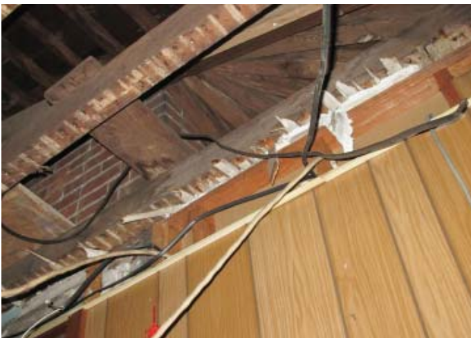
Roof framing over the curved wall
