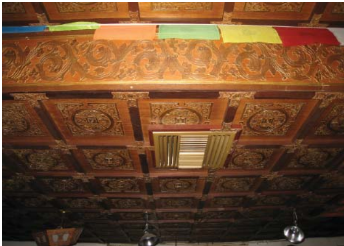
Coffered ceiling on the first floor
