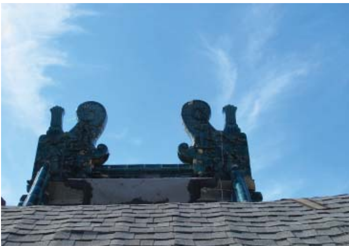
Dragon decorations on the ridge of penthouse roof
