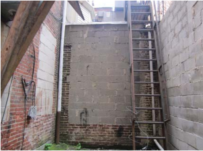
Blockage of an opening at the back of side addition
