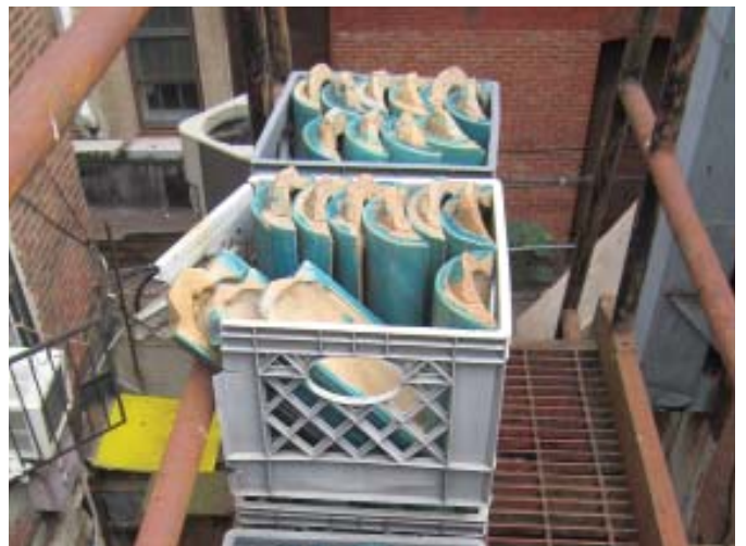
Glazed roof tiles stored on the fire escape deck
