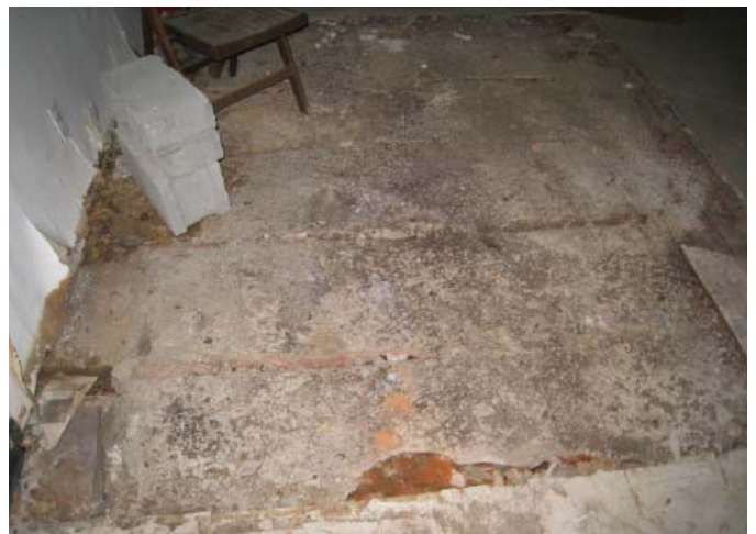
Exposed brick and concrete under floor boards on the first floor
