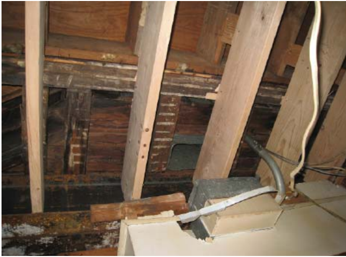
Timber frame supporting bay window on the second floor
