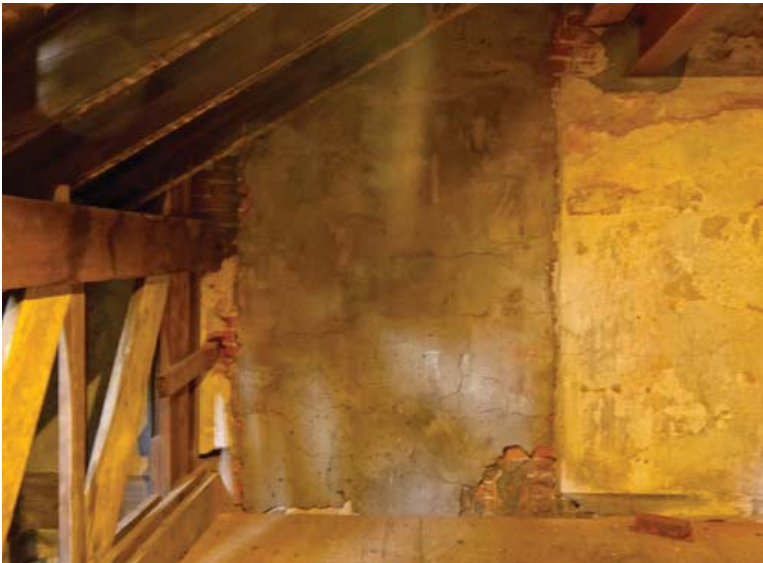
The building's original pitched roof framing is still intact
