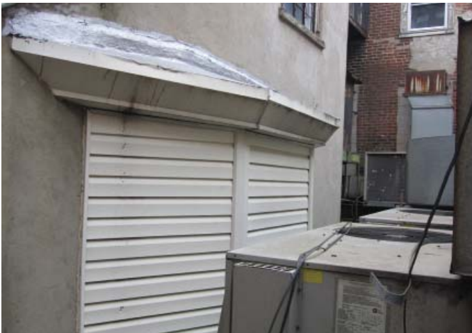
Bay window blinded with vinyl siding
