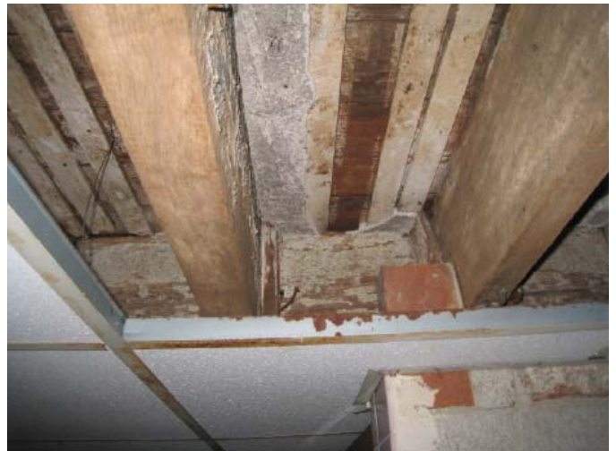
Floor joists above ceilings in the basement
