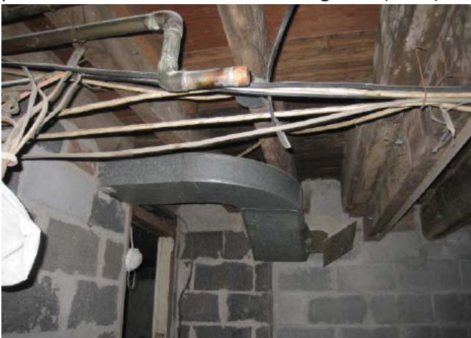
Remains of electricity facilities, 1900s-1960s
