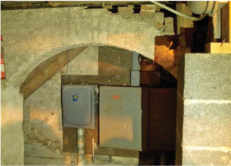
Remaining brick arch at front portion of basement
