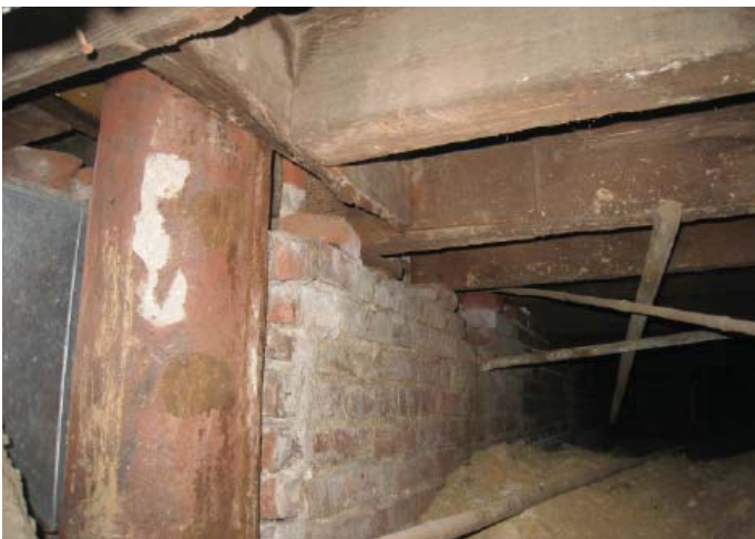
Basement addition under former alley
