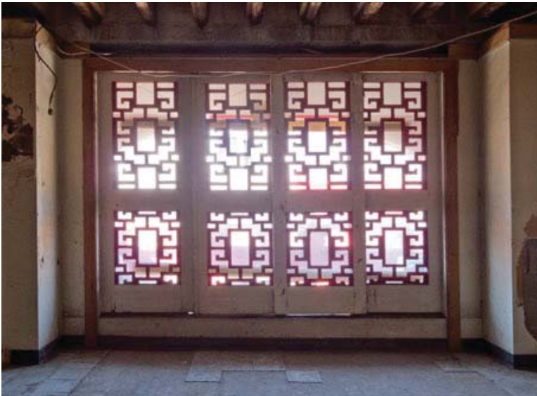
The third floor balcony, with a sliding screen door
